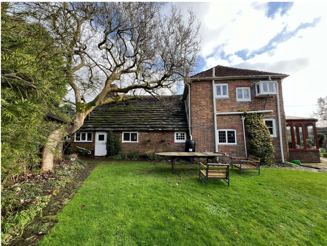
Looking East at rear elevation of house
