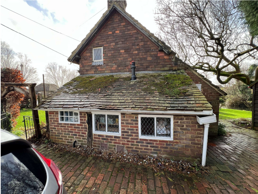
Looking South at side elevation
