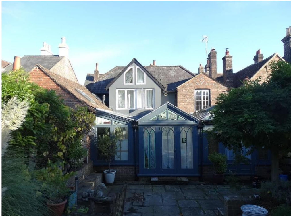
Figure 7: Marlow House, west elevation, prior to the implementation of the scheme not approved
