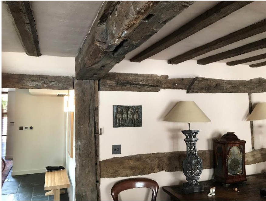
Figure 12: main E-W ceiling beam to the living room showing the location of an original partition and doorway adjacent to the northwest wall.
