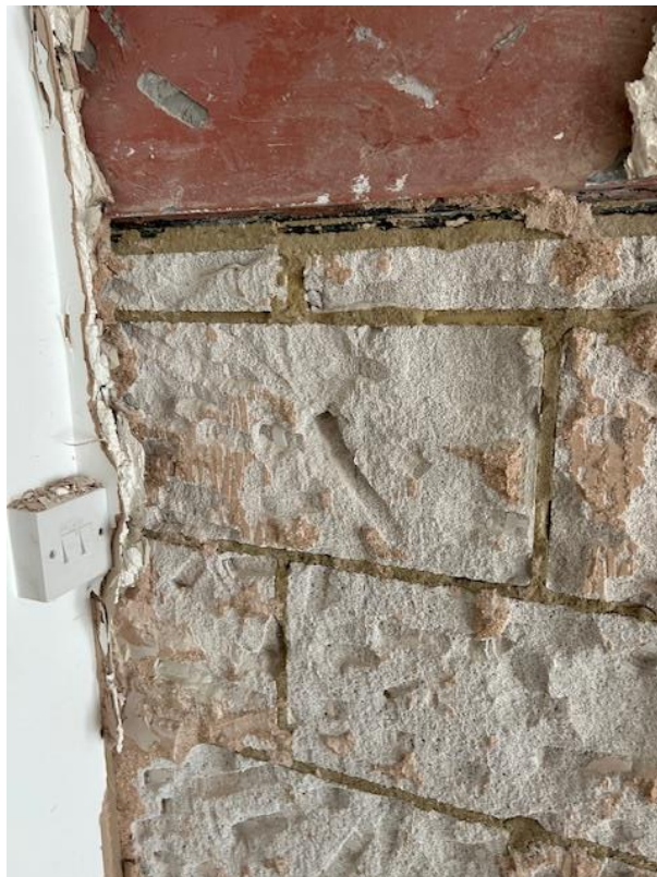
Figure 35: Blockwork construction underlying the exposed timber stud wall with stonework nogging shown at Figure 16
