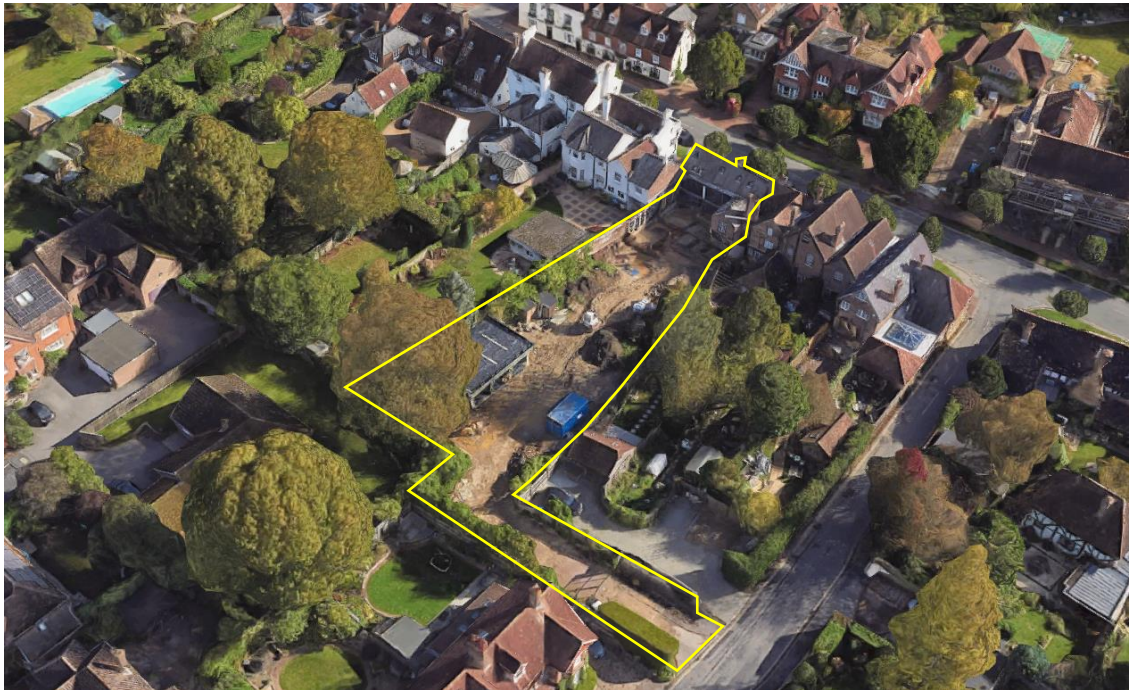
Figure 3: Bird's Eye View of the Site from the west (outlined in yellow)
