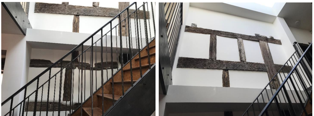
Figure 37: Box framing to west wall of the 15 th century house with internal windows infilled with wood wool panels and lime plaster.
