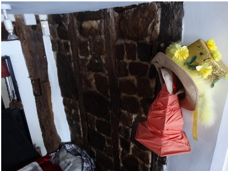
Figure 16: feature wall to the partition between the entrance hall and southern bay dining room. Source: Desbruslais Chartered Surveyors Statement of Heritage Significance of 13 th October 2022
