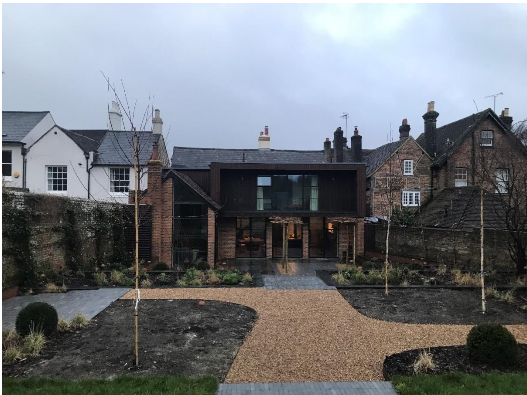
Figure 32: View of Marlow House from the rear garden (west). Note the prominence of the restored 15 th century roofscape.
