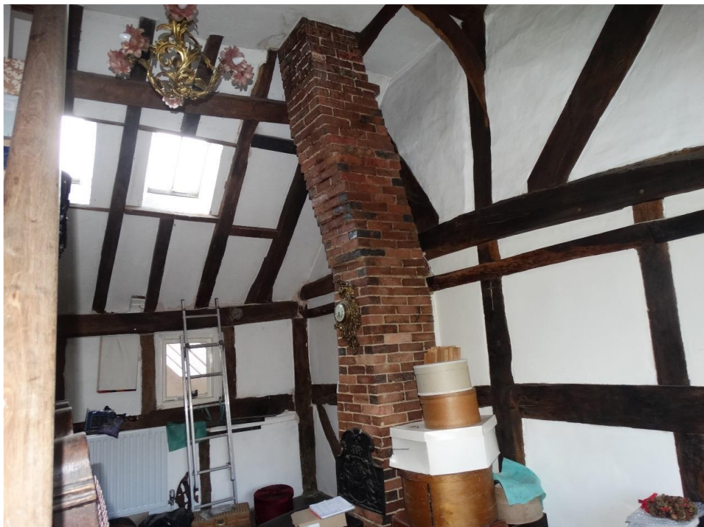
Figure 9: 19 th century brick stack adjacent to the north wall of the 15 th century house prior to its removal. Source: Desbruslais Chartered Surveyors Statement of Heritage Significance of 13 th October 2022
