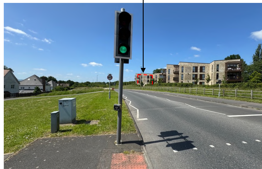
VIEW A - VIEW WEST ALONG ROCKY LANE
