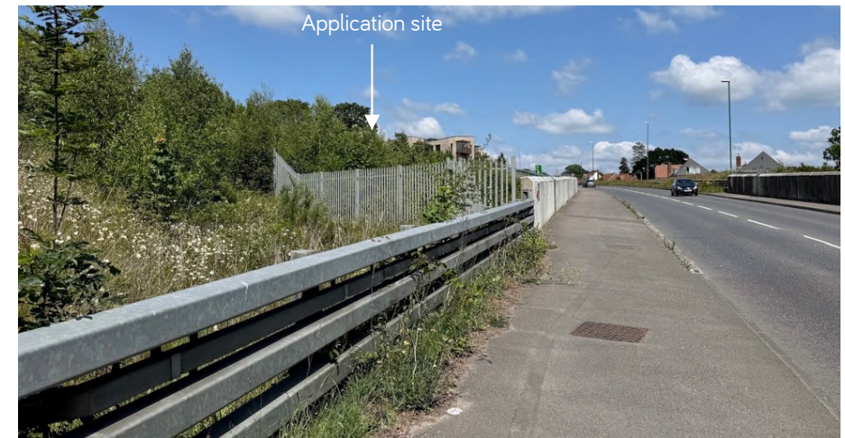
Fig.5 View of site looking east along A272
