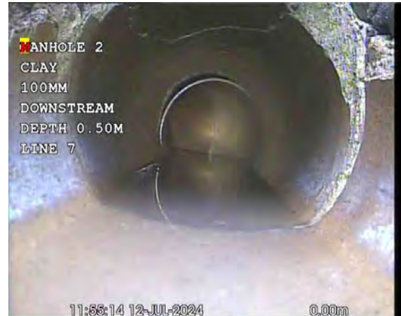
MH2X_71184cee-8274-417a-b5b5-87d394df23a5_20240725_092449_717.jpg, 00:00:28, 0.00 m Water level, 10% of the vertical dimension
