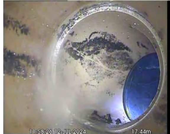
MH2X_ecbc01d4-5401-430c-a4cc-4e8128ef4209_20240725_093238_853.jpg, 00:02:20, 17.44 m Line deviates right
