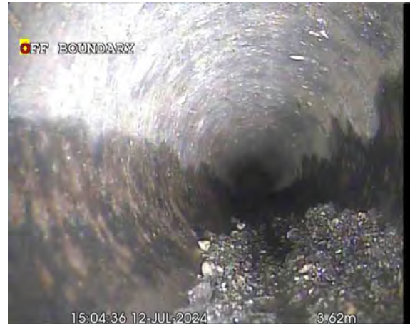
MANHOLEX_d574a494-dbda-46c8-9c0c-5e761cd3587d_2024 0725_102253_591.jpg, 00:01:02, 3.62 m General remark, **BOUNDARY POINT**
