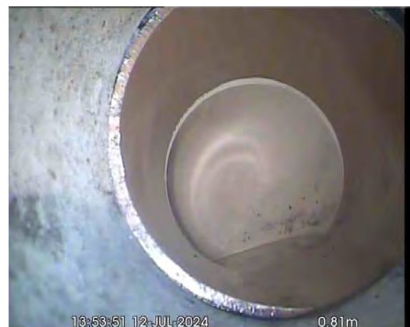
SVPX_6dc84003-04ba-4f4b-a2bc-ade636d85d44_20240725_095258_153.jpg, 00:00:43, 0.81 m Material changes to polyvinyl chloride
