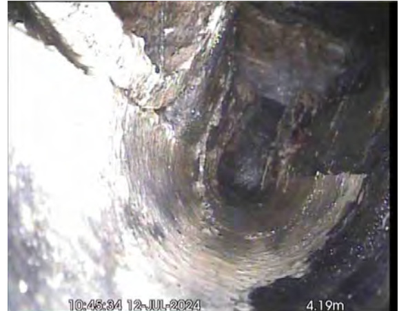
MH6X_27aff4e3-af3d-432c-bcaa-89feb1b6036e_20240725_092322_445.jpg, 00:01:15, 4.19 m Finish node, manhole, reference: MANHOLE 6 (MH6)
