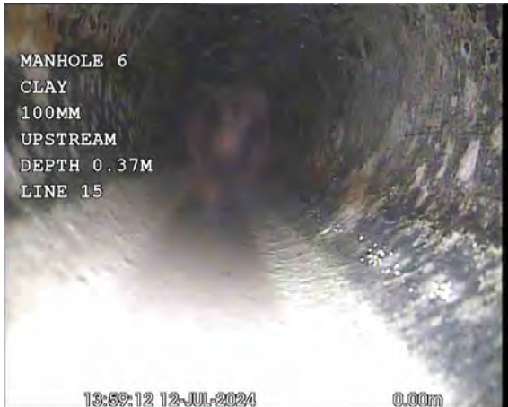
BASINX_06fc371f-58ec-4fc7-ae67-9aa21aea31b2_20240725_100939_050.jpg, 00:00:16, 0.00 m Start node, manhole, reference: MANHOLE 6 (MH6)
