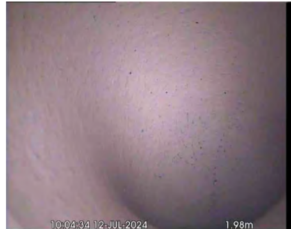
GULLYX_ea8e3b67-ae80-4672-8aa1-6d7696ac026d_20240725_090241_494.jpg, 00:01:10, 1.98 m Finish node, gully, reference: GULLY
