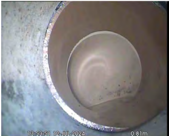
SVPX_37643050-054d-409b-a034-ef1a40900360_20240725_095307_792.jpg, 00:00:43, 0.81 m Size changes, new size(s), 110mm high
