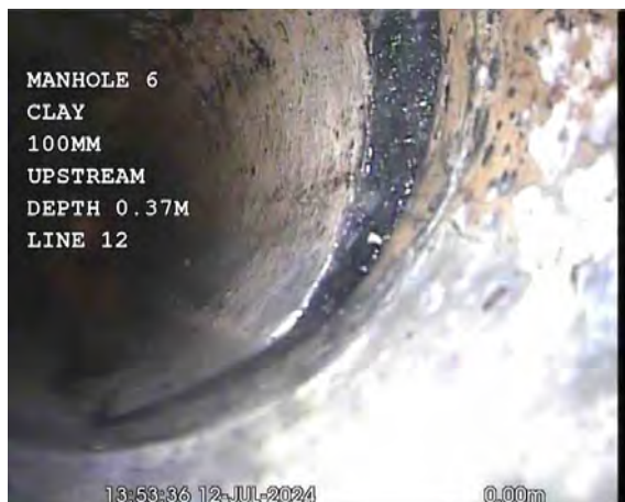
SVPX_1032148c-1afa-44ba-b9d4-c41939b75ca1_20240725_095215_787.jpg, 00:00:28, 0.00 m Start node, manhole, reference: MANHOLE 6 (MH6)
