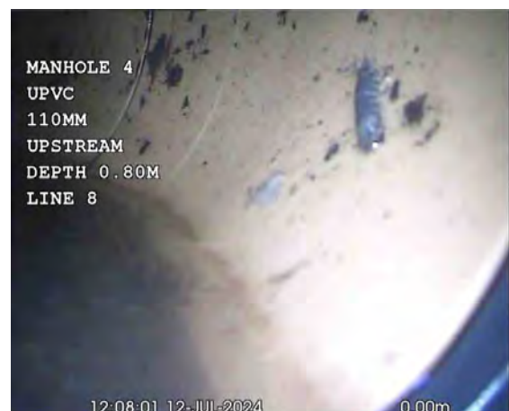
CAPPED OFFX_93c2d75d-b2fd-43d0-9440-17bfa1c0c76e_20240725_093409_690.jpg, 00:00:39, 0.00 m Water level, 5% of the vertical dimension
