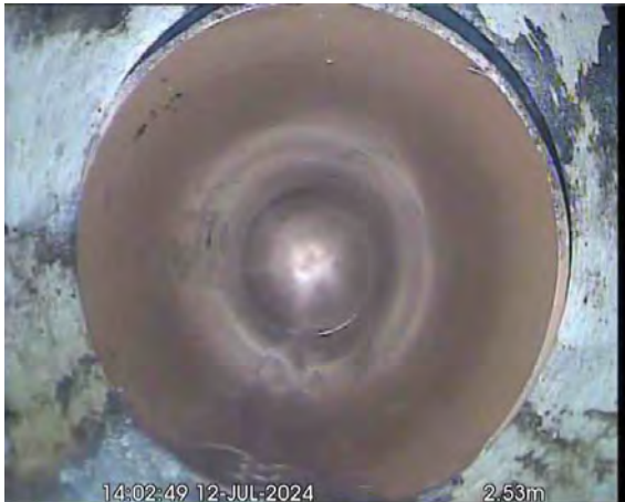
GULLYX_28ba29e2-e34d-48d9-9e89-110dddac1be6_20240725_101336_880.jpg, 00:01:00, 2.53 m Material changes to polyvinyl chloride
