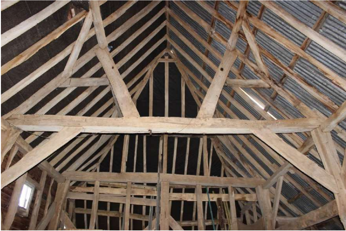
Tie-beam of frame B looking east with raking struts supporting the purlins with wind-braces below them
