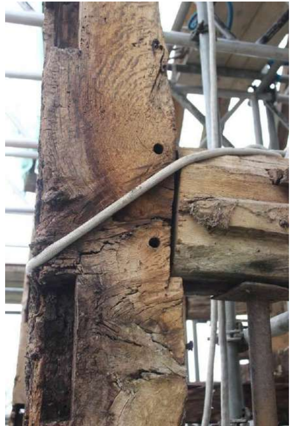
Frame A interval post with taper burn on south face and ledge supporting the axial beam
