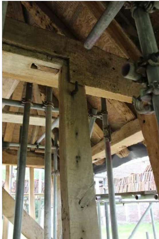
Upper pintle for internal 1 st floor door to east of post B1 Note original stud mortice was to the east
