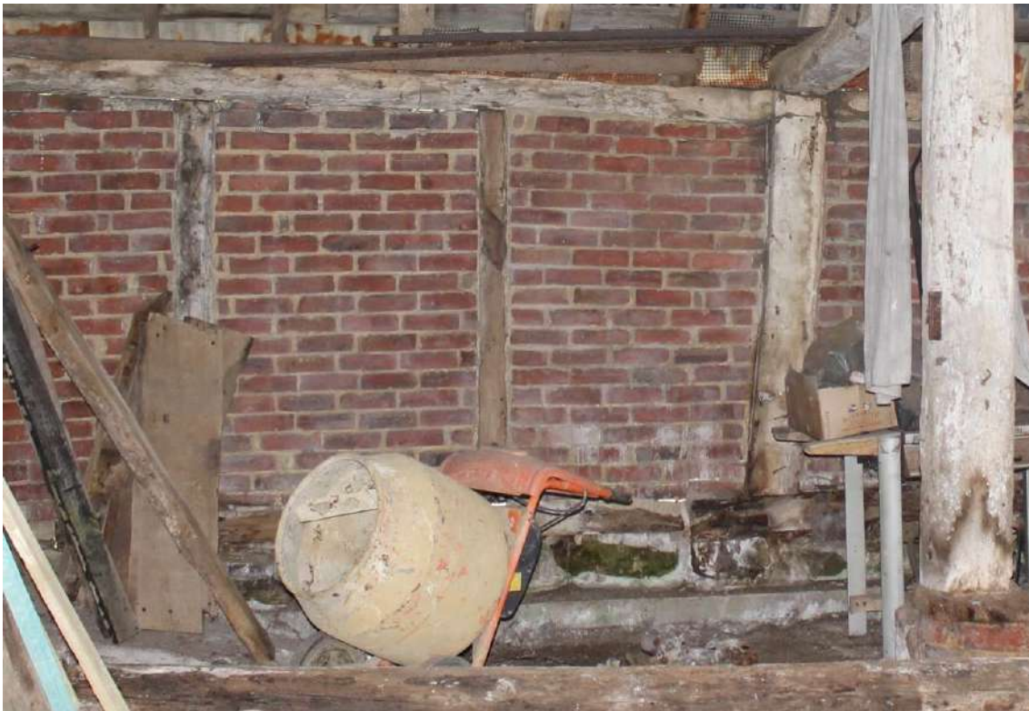
Aisle wall east of frame C showing concrete below stone plinth & brick infill both with cementitious mortar
