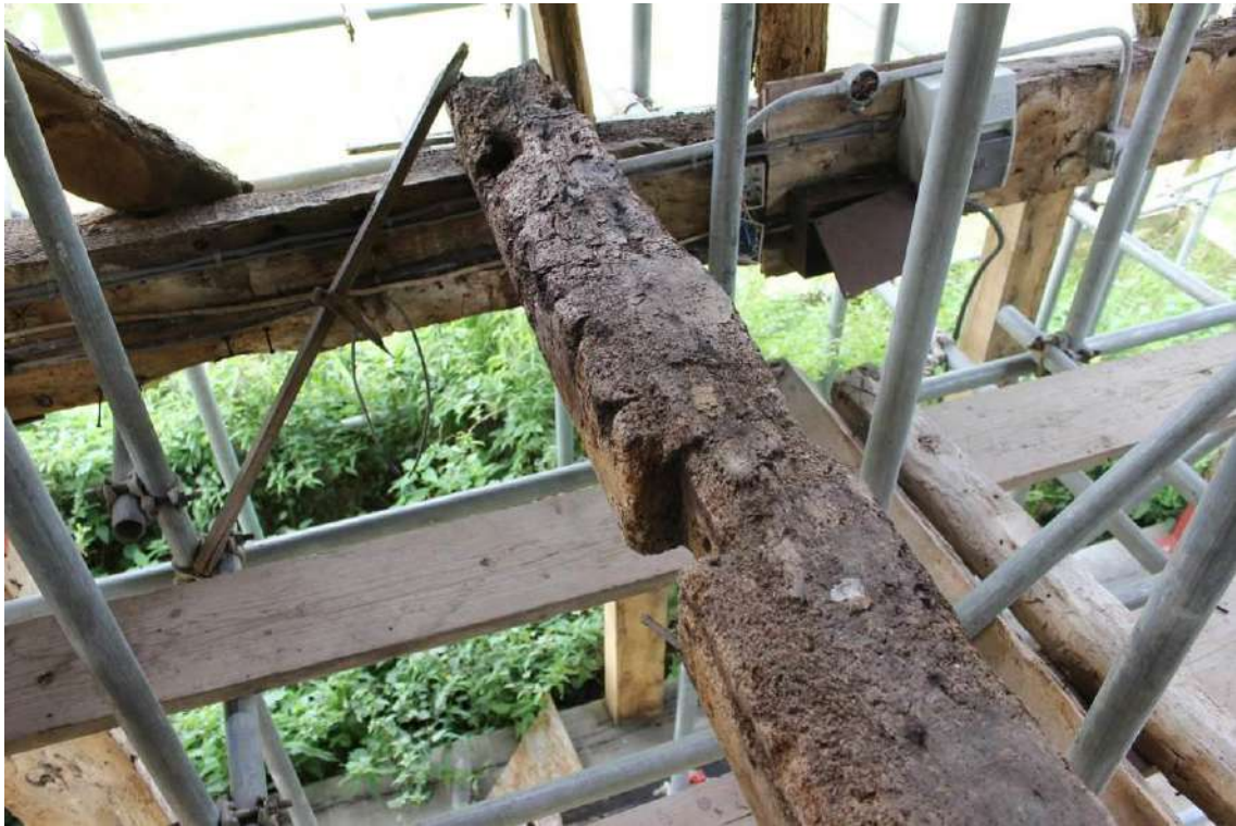
South face of joist 7 has lap joint for a vertical timber
