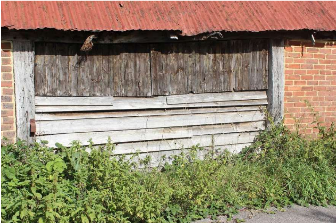
South elevation doorway between post D3 and C3
