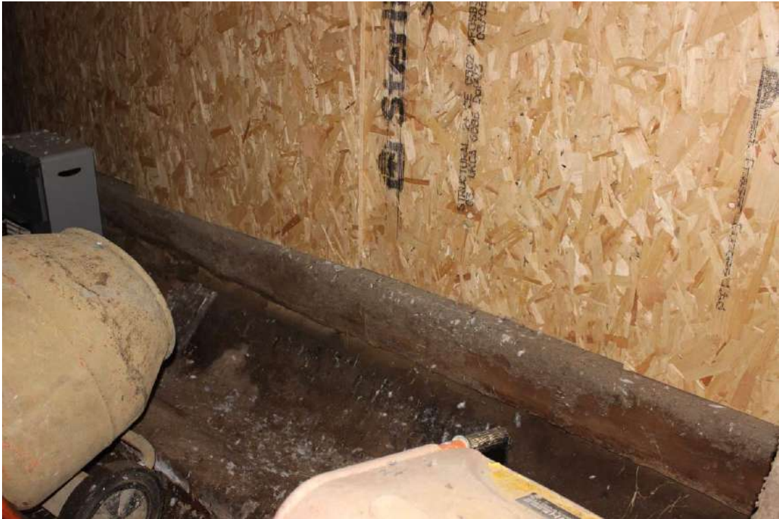
Concrete and brick food trough on west side of frame A
