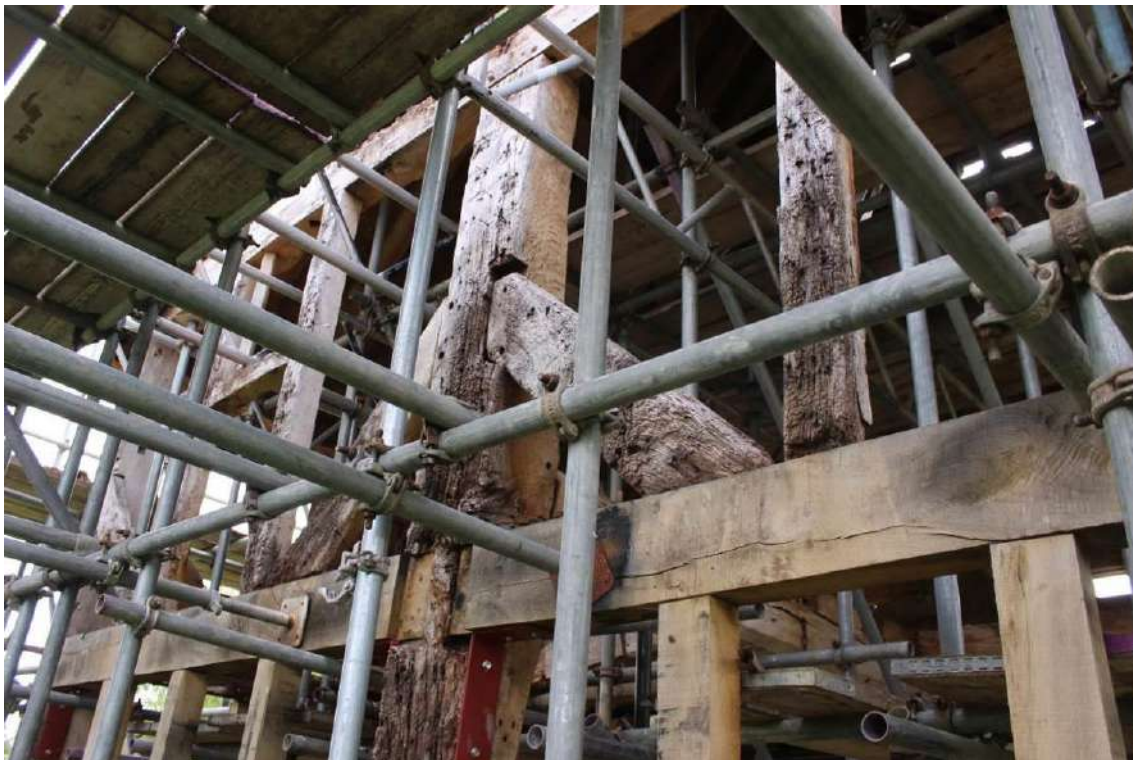
North Elevation showing short straight down-braces and mullion window above left
