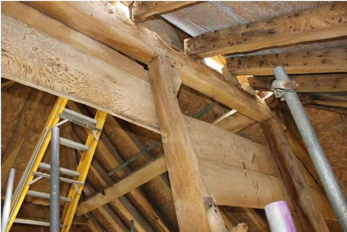
South side of frame B collar supporting reused timbers as rafters for later roof on right
