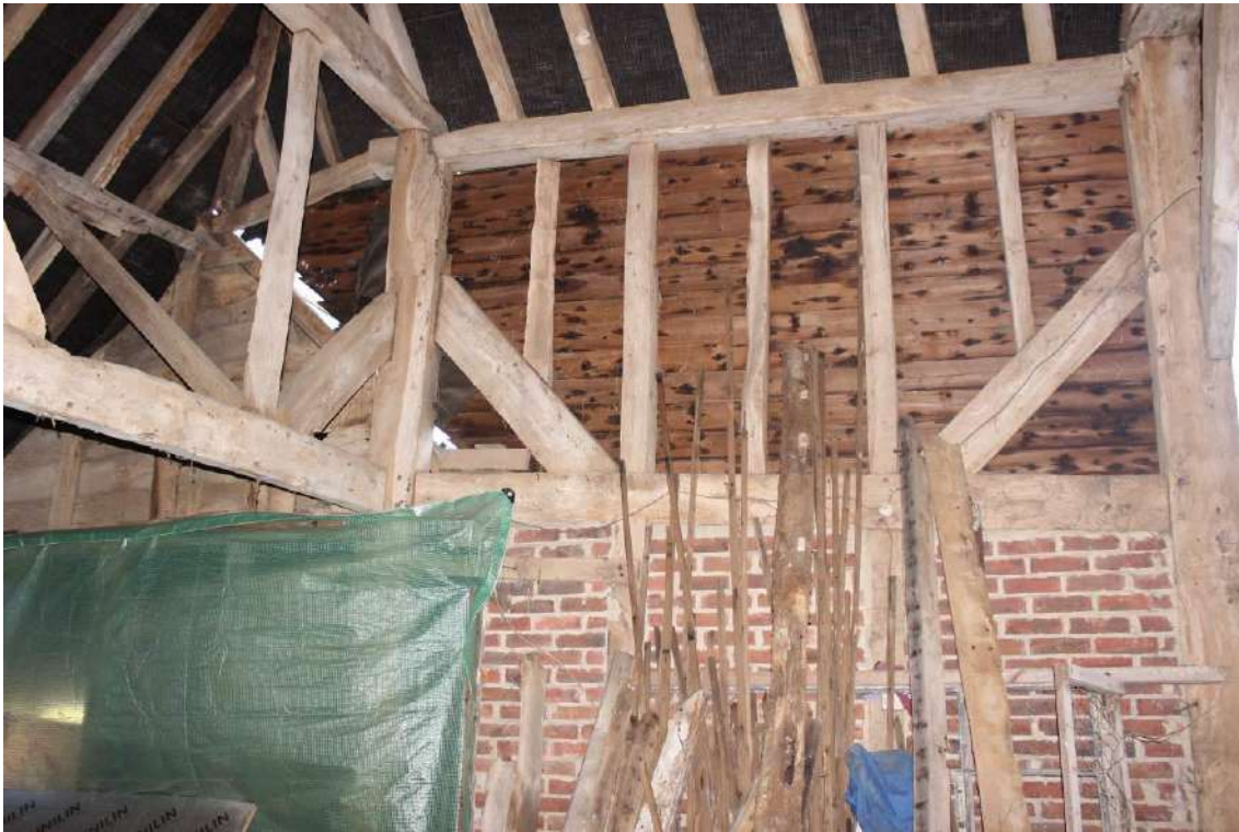
Typical construction of main range north elevation, post E1 on left and post D1 on right
