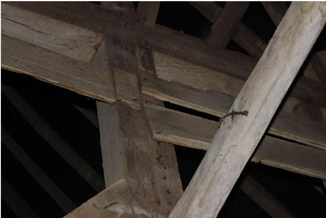
Surviving individual weatherboards on east side of frame A, just below tie-beam
