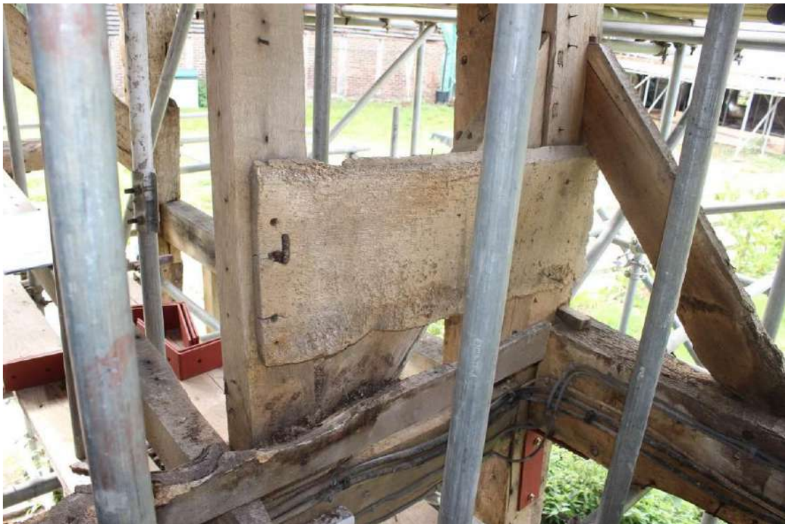
Lower pintle for internal 1 st floor door to east of post B1
