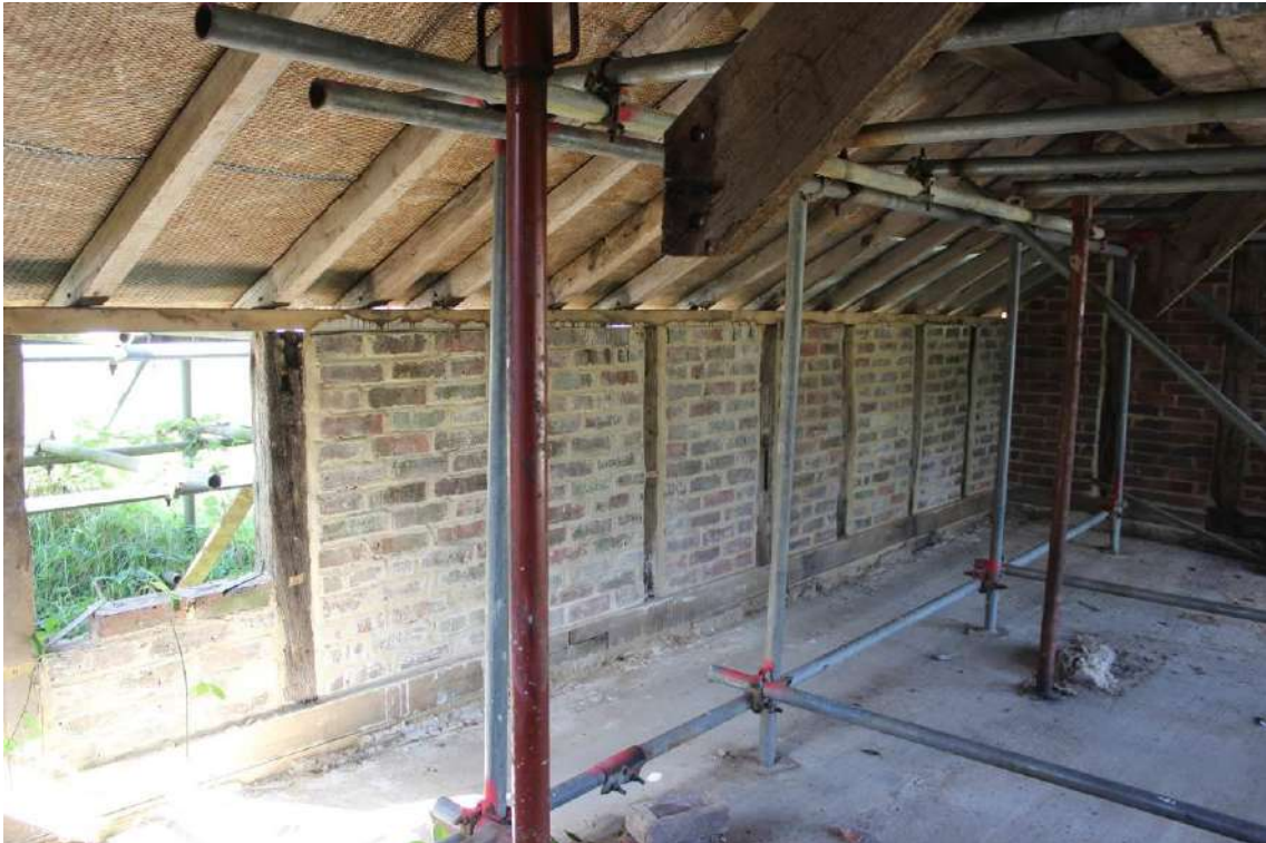
Looking northwest within west end face-wing, later outshot to its west with modern brick infill
