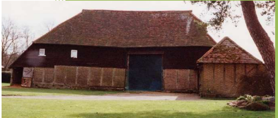
Barn. North (front) Elevation (2007)
