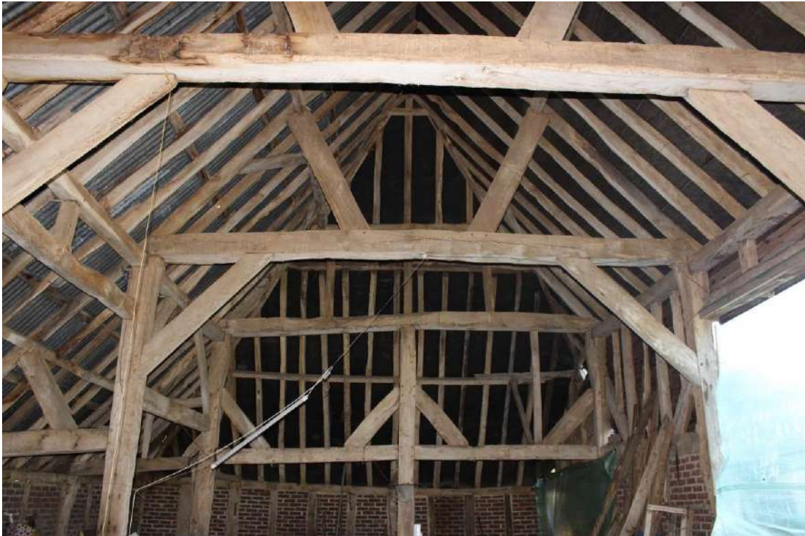
Looking west. Frame C tie-beam at top of image with frames D and E beyond
