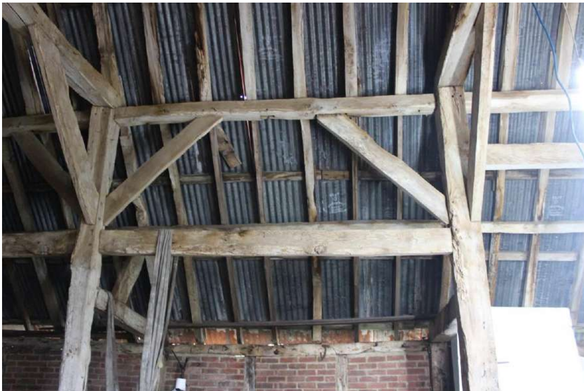
Typical construction of main range south elevation with girthing beam and up-braces. This is post B2 on left, post C2 is on right, note higher girthing beam C2-D2 at south of midstrey.
