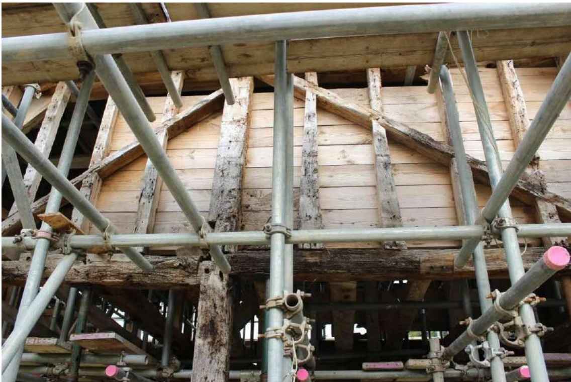
South face of frame C showing phase 3 infill with long diagonal braces
