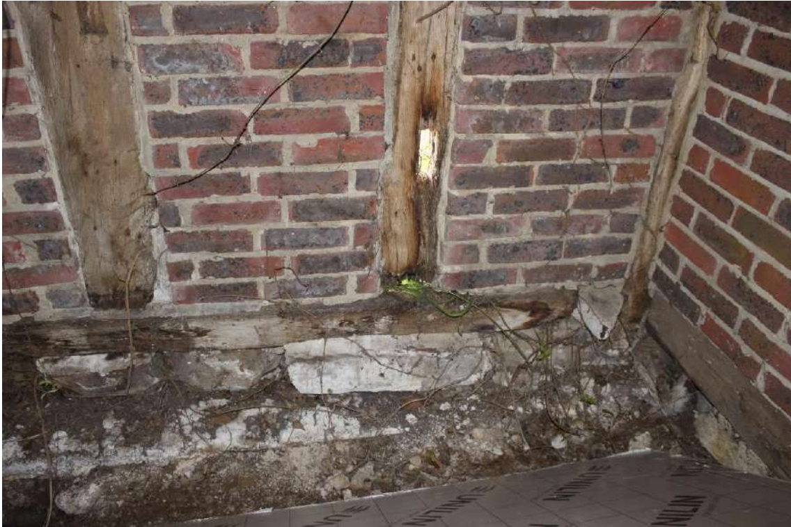
Concrete below stone plinth of west outshot. Looking south at corner L1
