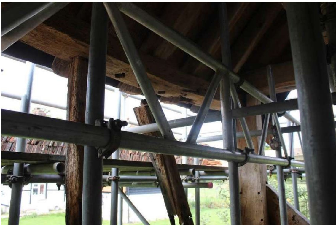
First floor mullion window in wall A1-B1
