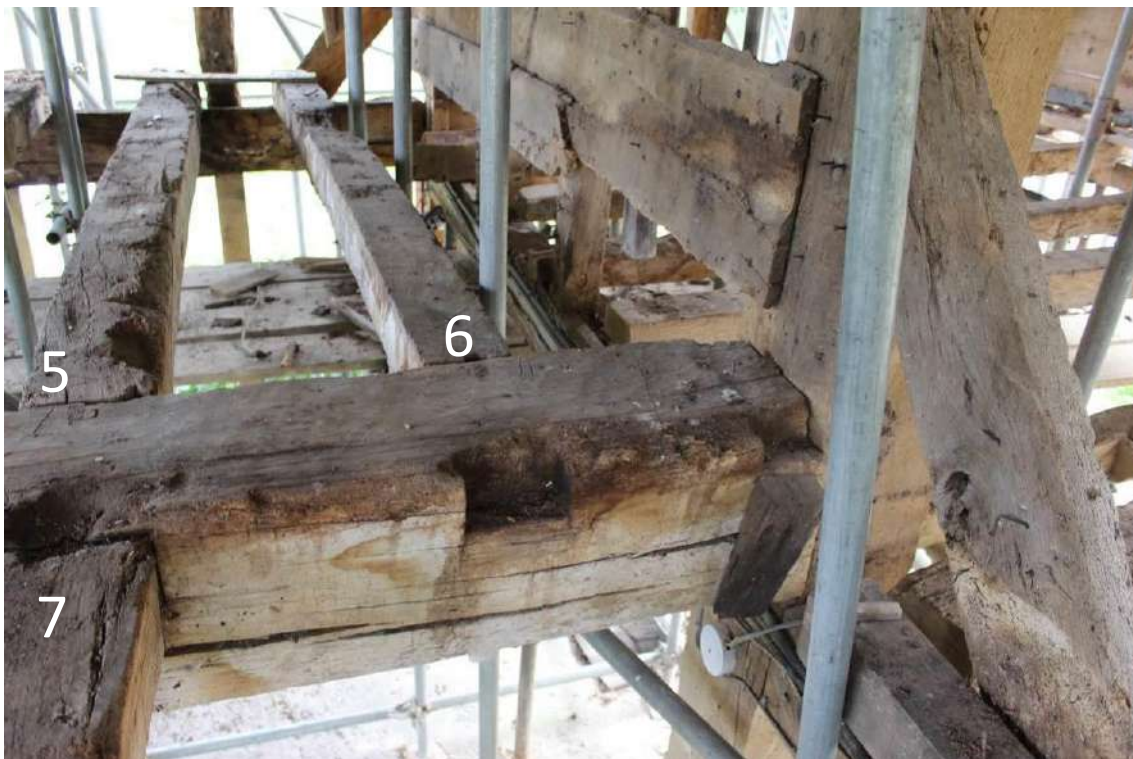
South end of axial beam A-B. Assembly mark numbers indicate no joist opposite No.6 Note remnant of original internal boarding
