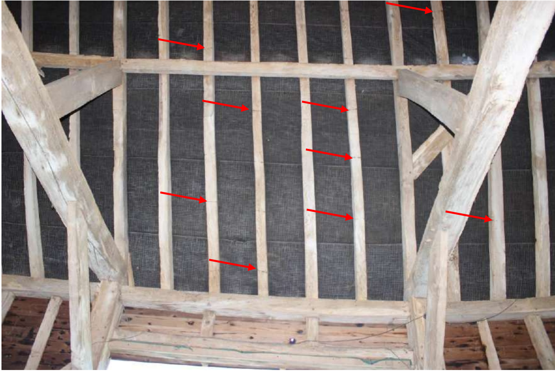
Roof above door D1-C1 in north elevation. Note thatching rope tar marks on original rafters
