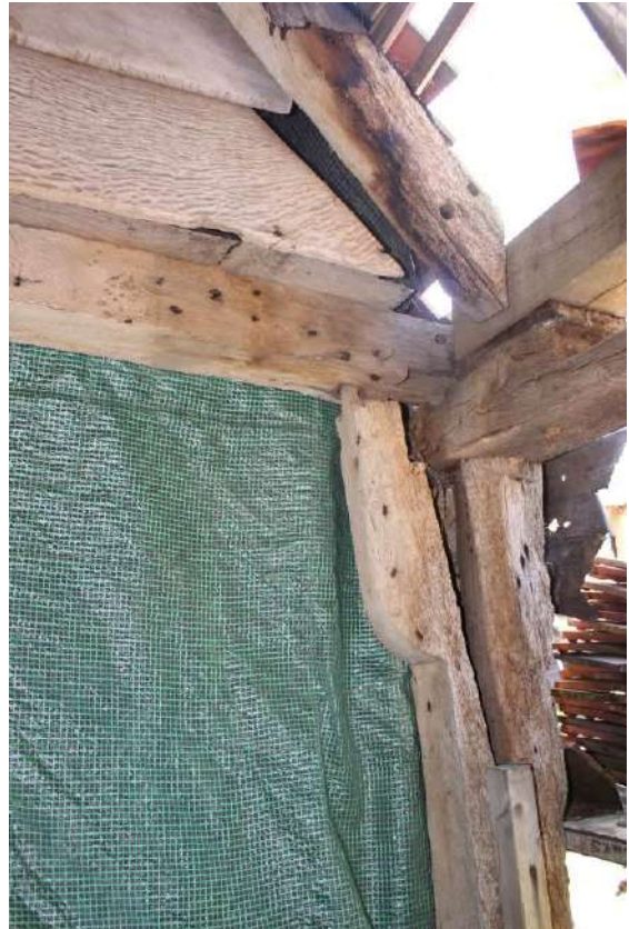
Gunstock jowl of post I1 and extended wall-plate for face-wing
