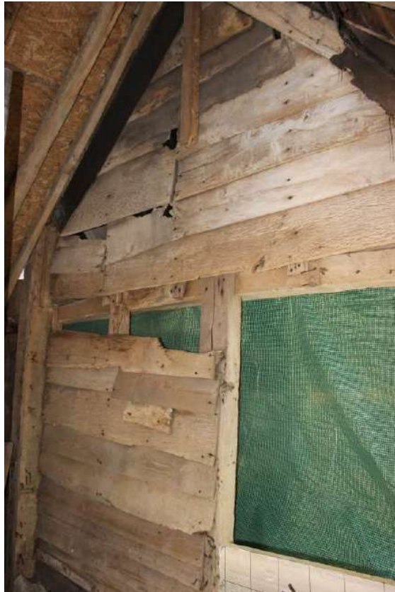
Earlier weatherboards where west end face-wing covers the north wall of main range
