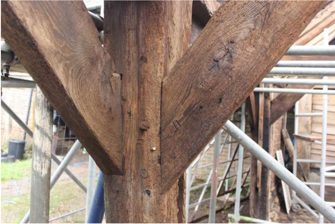
Chiselled assembly marks on post G2 looking southeast
