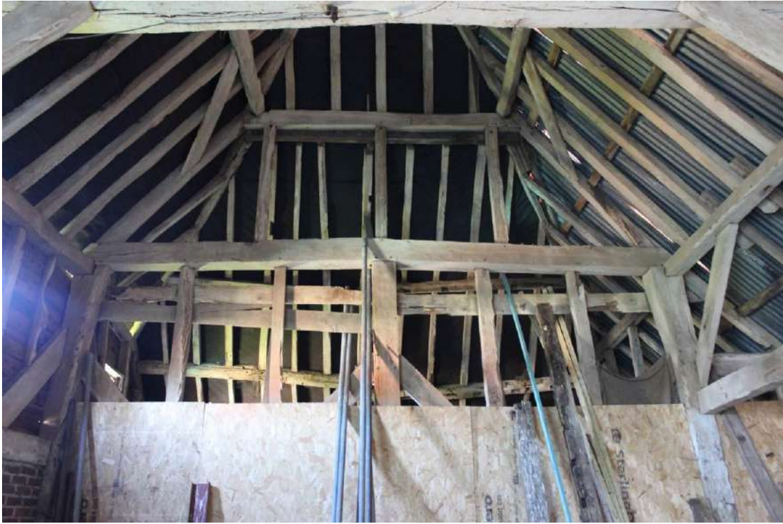
Upper view of frame A looking east with the eastern end outshot beyond
