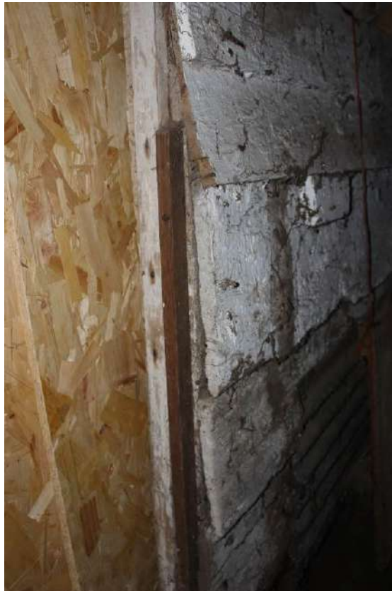
Surviving section of early weatherboards on east side of frame A
