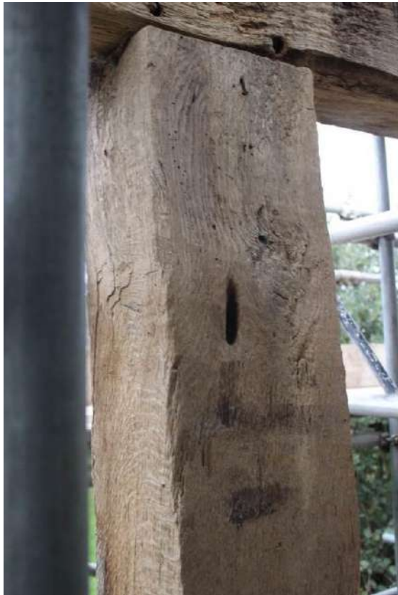
Frame A interval post with taper burn on south face and ledge supporting the axial beam
