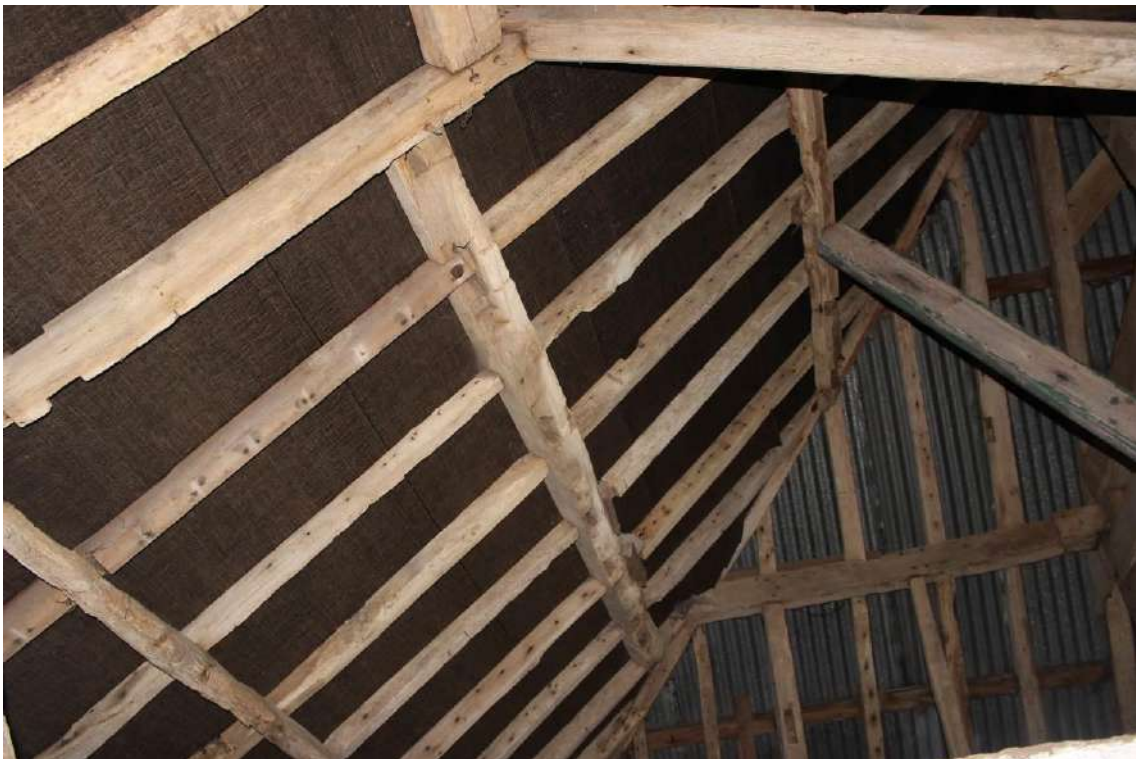
Staggered butt-purlin roof of east outshot (looking south)
