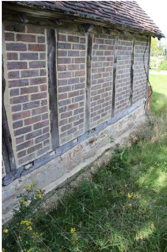
East end showing concrete below the stone plinth and brick infill of panels both with cementitious mortar
