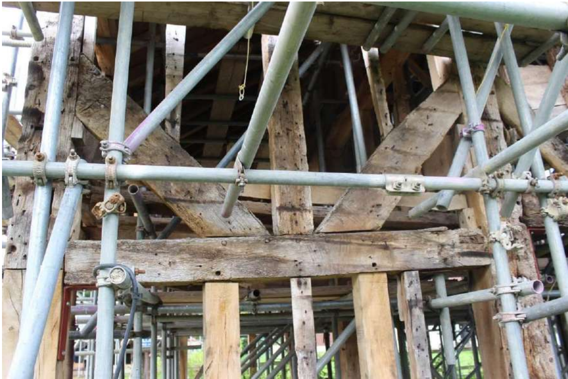
Girding beam C2 (left) - B2 (right). Note assembly mark 4 on the right hand down-brace
