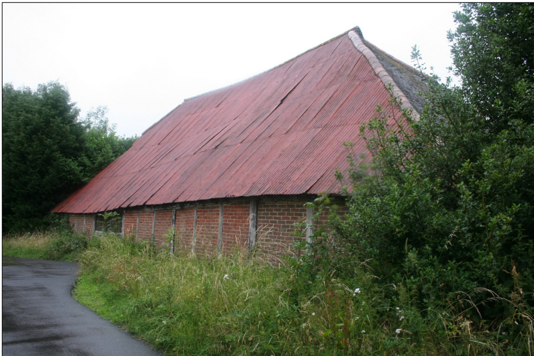
Photo 4: View of the southern elevation of the Grade II Listed Barn from Furnace Farm Road.
