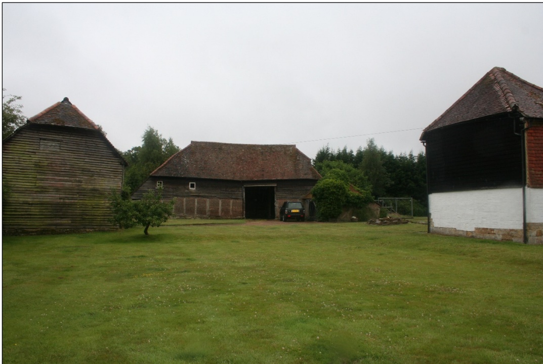
Photo 2: View of the Grade II Listed Granary, Barn and Farmhouse from the north.
