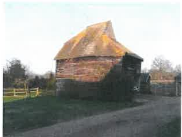
Photograph 25. The granary building at Gibbshaven Farm seen from the west on the entrance drive to Gibbshaven Farm.
