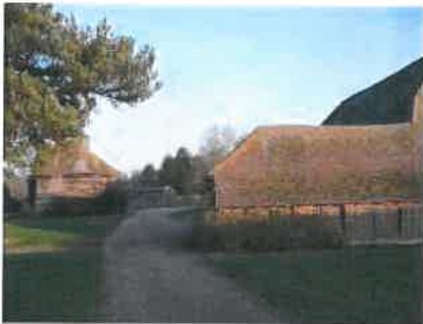
Photograph 26. The west elevation of the single-storey offshot to Gibbshaven barn, with the granary in the background.
