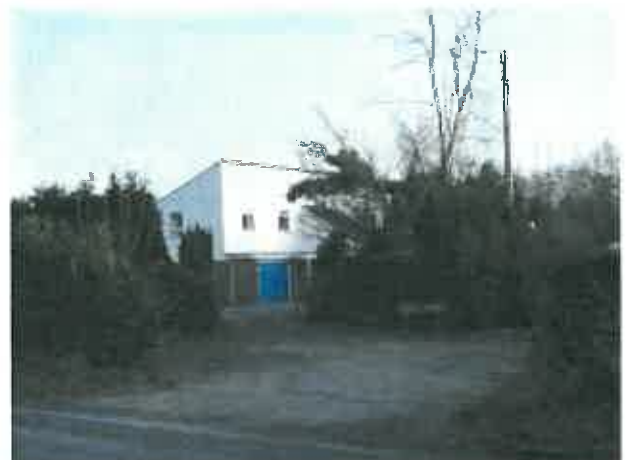
Photograph 10. The dwelling house associated with Felbridge Nursery on the east side of Felbridge Road.
