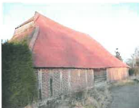
Photograph 34. The south elevation of the barn facing onto Furnace Wood Road showing the corrugated iron pent roof, and the half hip west return. The elevation comprises oak posts with brick infill panels. The threshing ventilation aperture is infilled with timber boarding.
