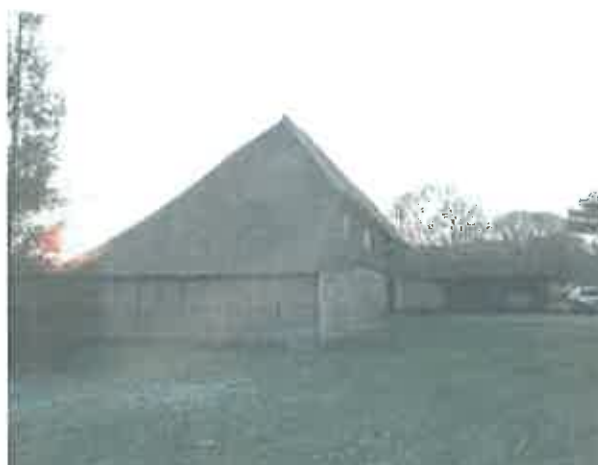
Photograph 33. The east elevation of the barn below the pent roof. The single storey offshot beyond
