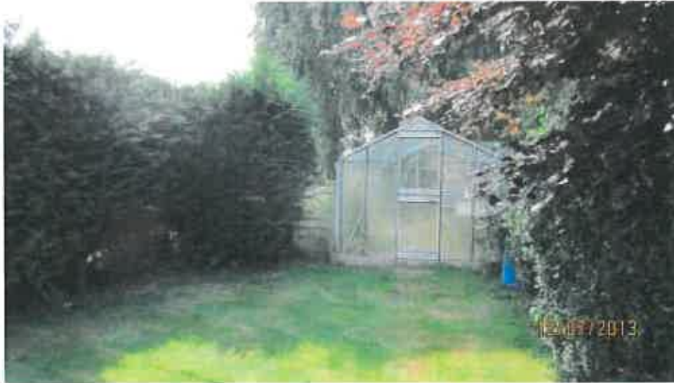
Photograph 285. View of the simple modern greenhouse at the west end of the lawn located to the west of the barn and adjoining offshot. The standard greenhouse has no architectural or historic merit and its proposed demolition will not result in any harm whatsoever to the setting or significance of the nearby listed buildings.
