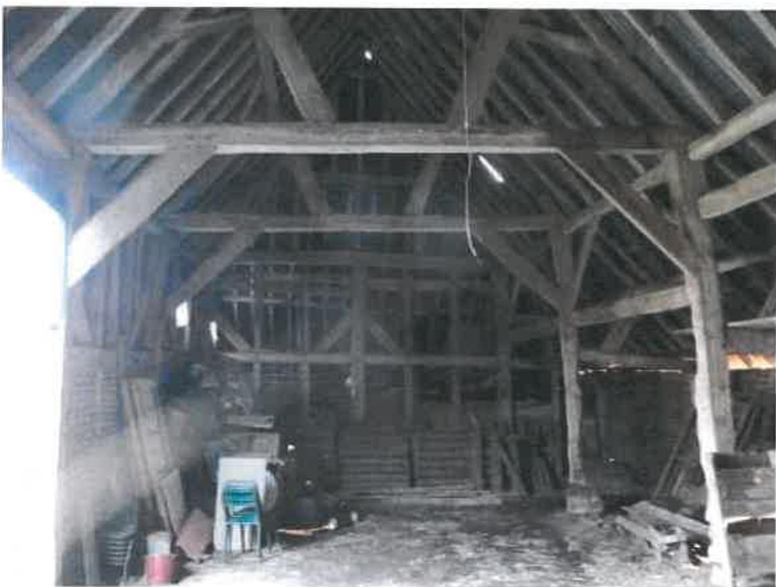
Photograph 37. The barn interior looking east, with an oak framed partition separating off the easternmost pent-roofed bay.
