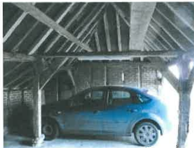
Photograph 42. The interior of the single storey offshot to the north of the main barn, looking north. Note the central oak post separating the two entrance-ways.
