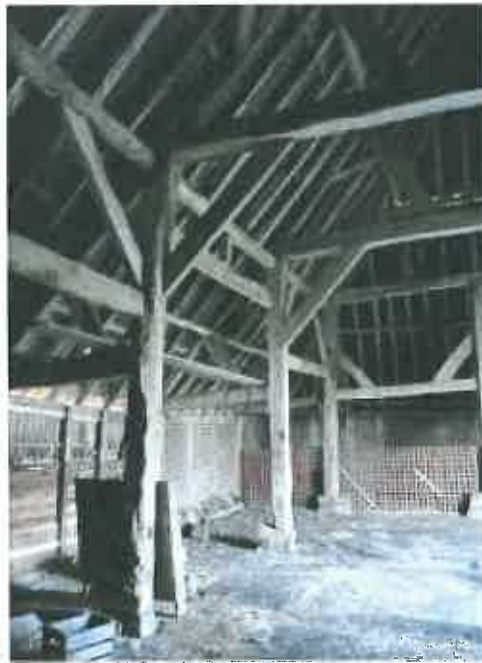
Photograph 38. The barn interior looking south-west showing the south aisle with the low threshing aperture boarded up.
