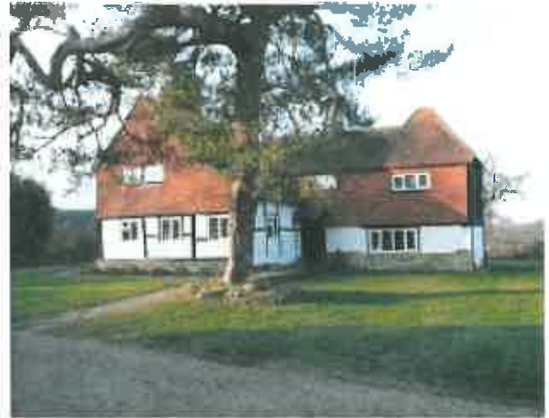
Photograph 19. The principal south facing elevation of the farmhouse at Gibbshaven Farm.
