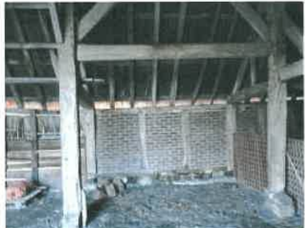
Photograph 41. Detail of the internal face of the south elevation to the barn.
