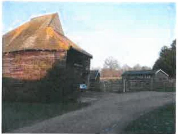
Photograph 27. View east along the entrance drive to Gibbshaven Farm with the granary on the left.
