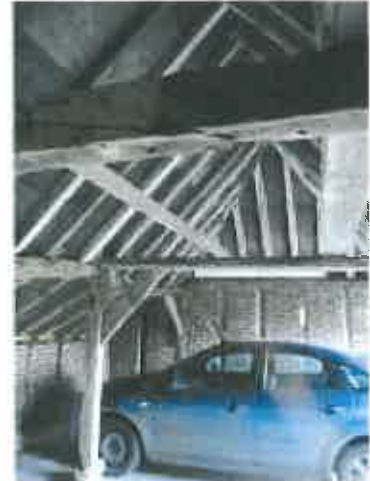
Photograph 43. The north west internal corner of the barn offshot
