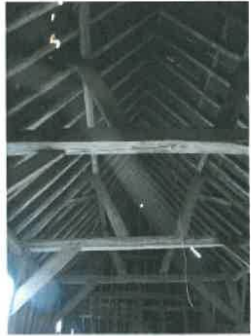
Photograph 39. The barn roof looking east.
