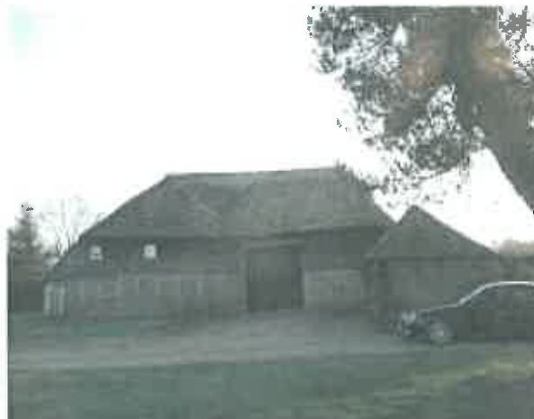
Photograph 31. The north elevation of Gibbshaven Barn showing the timber frame with brick infills to the panels on the lower level and oak weatherboarding with two windows above
