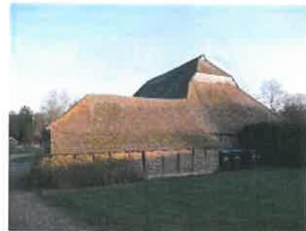
Photograph 29. The west elevation of Gibbshaven Barn.
