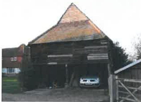
Photograph 24. The south elevation of the granary building at Gibbshaven Farm
