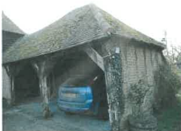
Photograph 30. The two bay open entrance to the single storey offshot to Gibbshaven Barn
