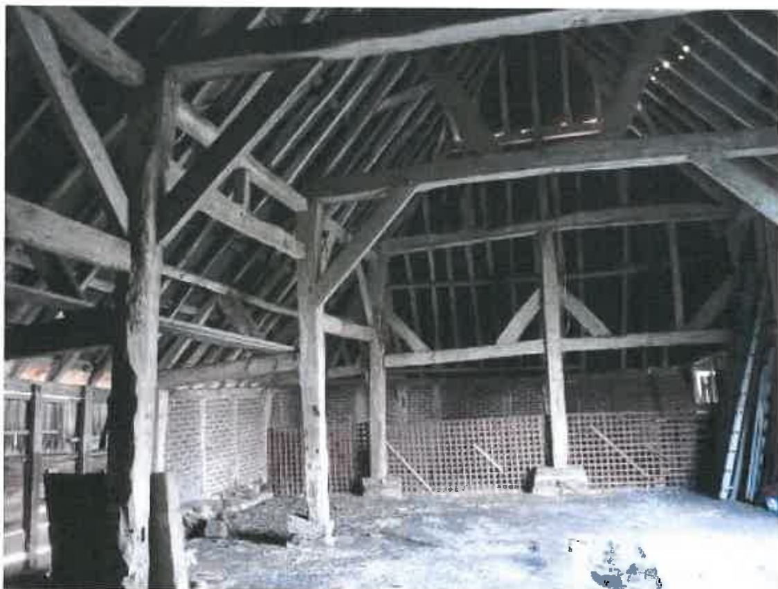
Photograph 36. The interior of the barn looking west. The oak posts are seated on stone plinths. Trussed box frames separate each of the four main bays and the end pent roofed bays. The roof slopes down as a pent roof over an aisle to the south, and the aisle returns under the hipped pent roof at the west end of the barn.
