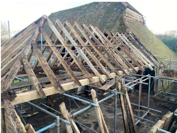
New purlin supporting existing rafters and ready for existing outshot rafters to be installed
