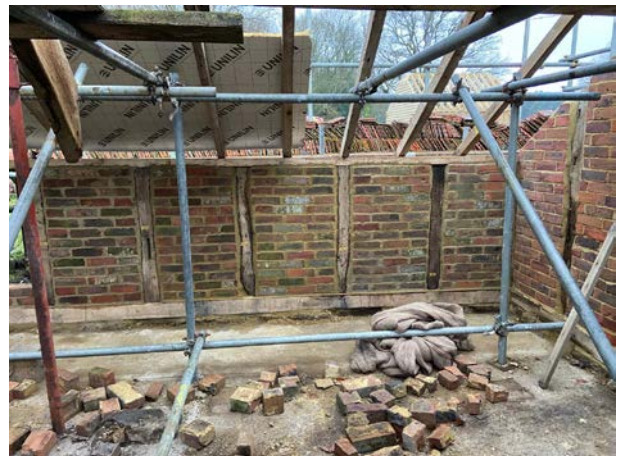
Rebuilt wall, with new sole, wall plates, and existing outshot rafters reinstalled
