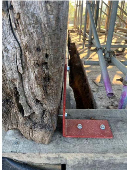
Existing wall member fixed to new sole Plate. (No tenon remaining)
