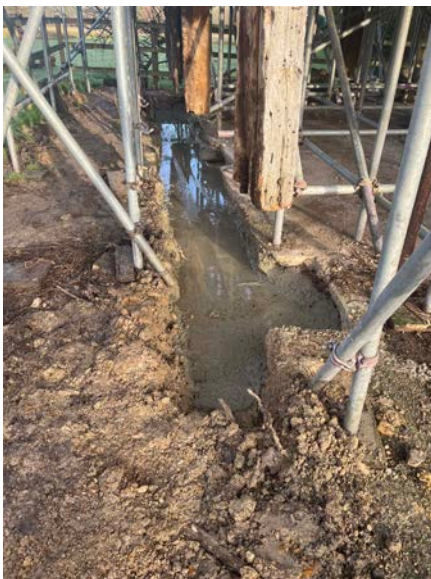
New concrete footings to support existing stone plinth
