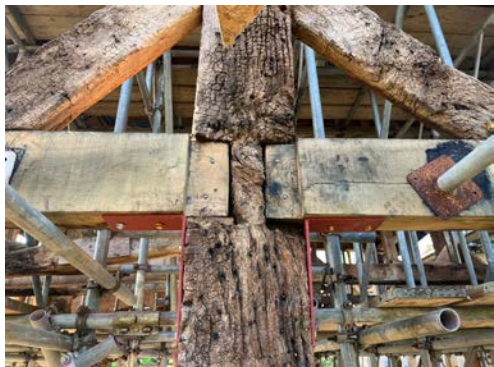
New oak roof truss members housed into existing damaged mortice. (New face to be spliced in)
