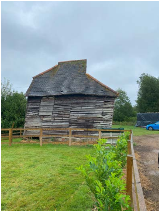
Granary west elevation showing racking
