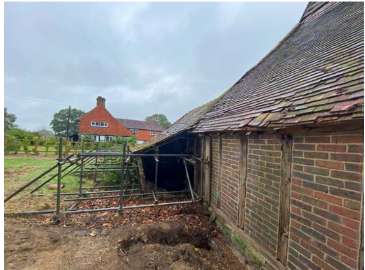
Scaffolding support frame prior to roof removal
