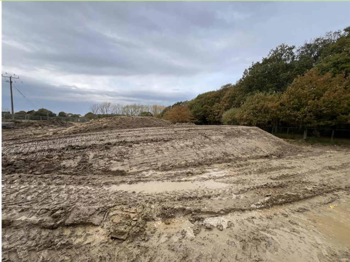
Plate 1 – Overview of topsoil stockpile TSP1 (Dated 05.11.2025)
