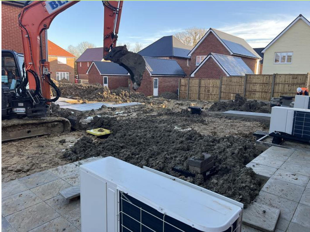
Plate 11 – Overview of topsoil being placed in Plots 3, 4, and 5 (Dated 03.12.2025)
