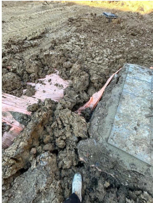
Plate26 – Photographs of membranes being installed within Plot 3-5, Plot 34
