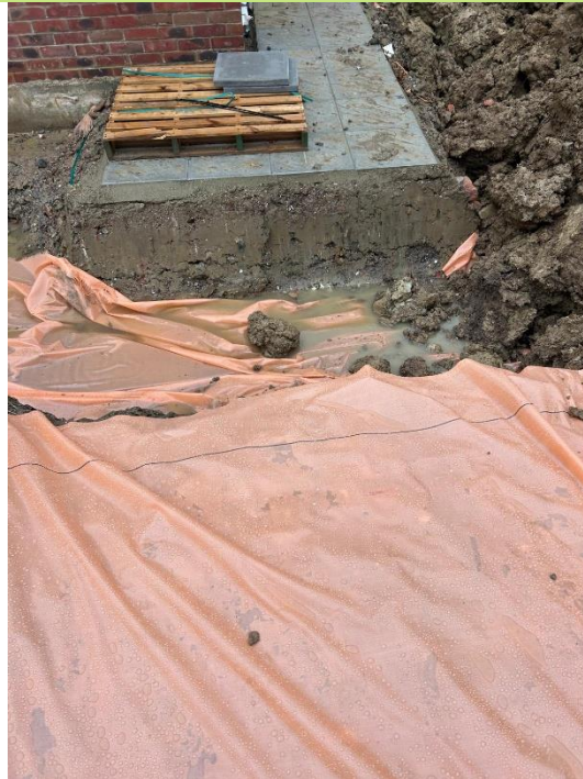
Plate 29 – Photographs of membranes being installed within Plot 3-5, Plot 34
