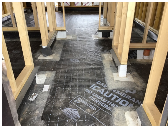
Overview of the Juta GP1 Gas Membrane that has been installed as an infill to plot 17.
