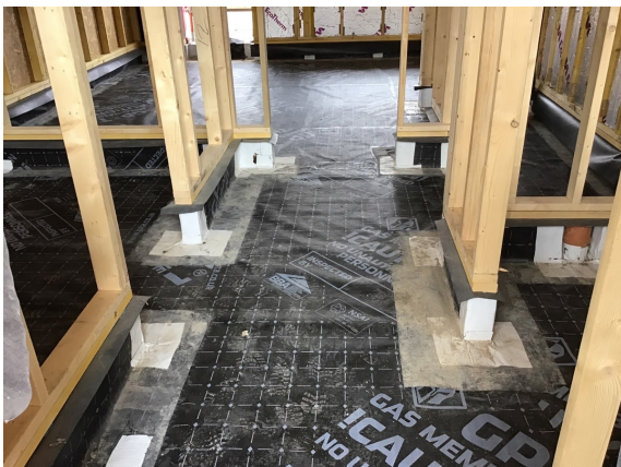
Overview of the Juta GP1 Gas Membrane that has been installed as an infill to plot 16.
