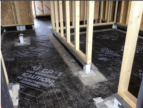
Overview of the Juta GP1 Gas Membrane that has been installed as an infill to plot 18.
