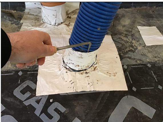
Probe testing a typical pipe penetration detail in plot 16.
