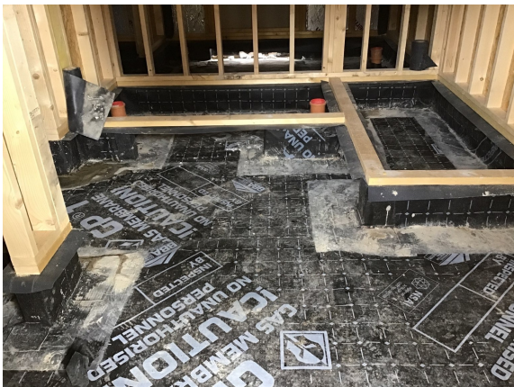
Overview of the Juta GP1 Gas Membrane that has been installed as an infill to detached plot 38.
