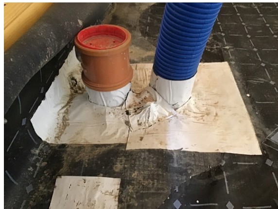
Typical double pipe penetration detailing in plot 18.
