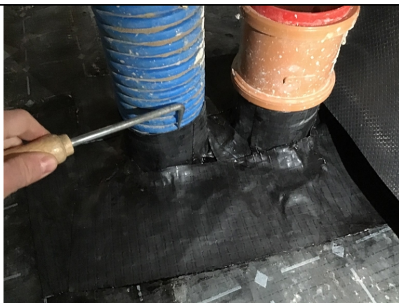
Probe testing all pipe penetration detailing in plot 38.
