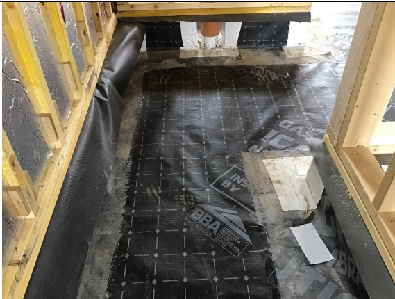
Overview of the infilled membrane in plot 16.
