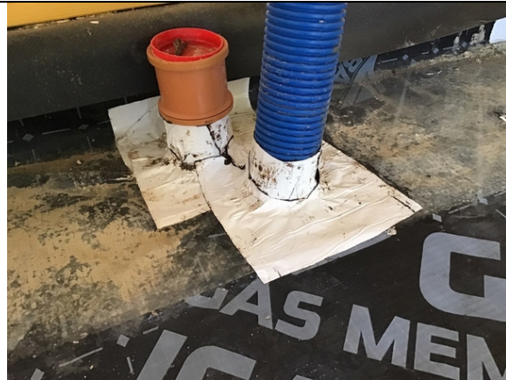
Typical pipe penetration detailing in plot 17.
