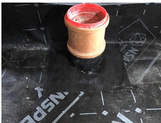
Typical pipe penetration detailing in plot 38.
