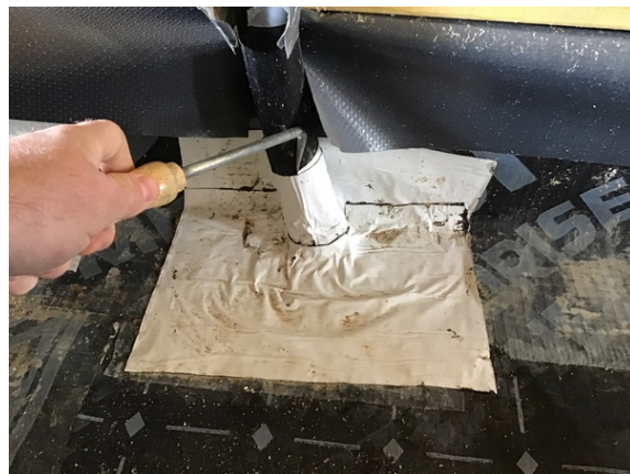
Probe testing all pipe penetration detailing in plot 17.
