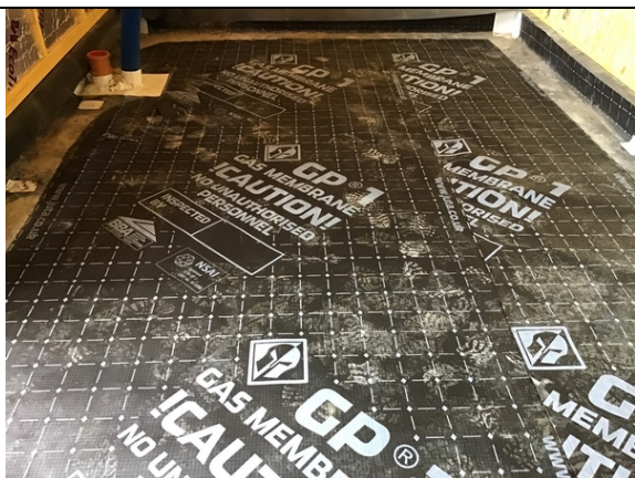
Overview of the infilled membrane to the room at the rear of plot 18.
