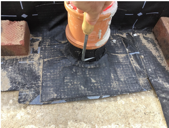
Probe testing a typical pipe penetration detail in plots 6 & 7.
