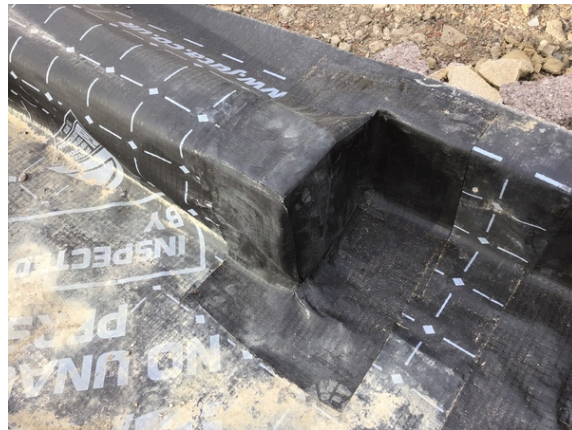
Typical door threshold detail in plots 6 & 7.
