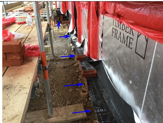
Overview of the extended Juta GP1 gas membrane that has been hand welded to the previously installed gas membrane that didn't span the cavity to the fronts of terrace plots 16-18.
