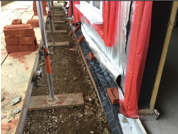
Overview of the extended Juta GP1 gas membrane that has been hand welded to the previously installed gas membrane that didn't span the cavity to the rear of terrace plots 16-18.
