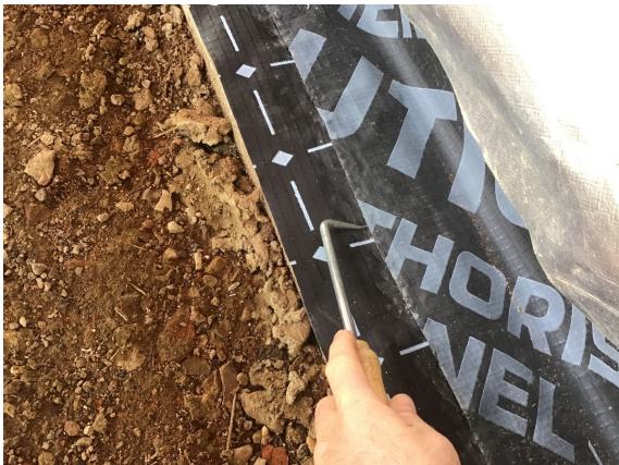
Probe testing all hand welded membrane laps.
