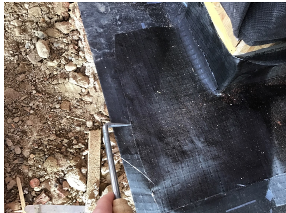
Probe testing a typical corner detail.
