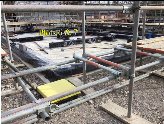
Overview of the Juta GP1 Gas Membrane installation to the perimeter and internal walls in maisonette plots 6 & 7.
