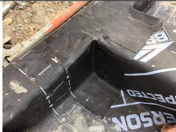
Typical corner detailing in plots 6 & 7.
