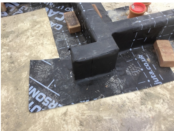
Overview of the the Juta GP1 gas membrane installed across the internal masonry brickwork on plots 6 & 7.
