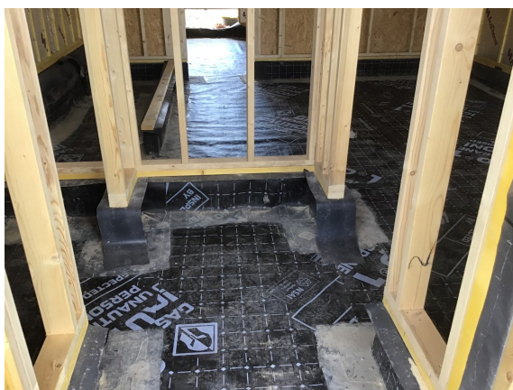
Overview of the Juta GP1 Gas Membrane that has been installed as an infill to plot 11.
