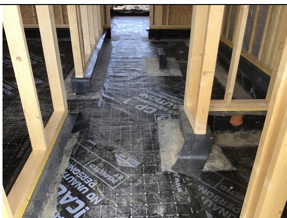
Overview of the Juta GP1 Gas Membrane that has been installed as an infill to plot 10.
