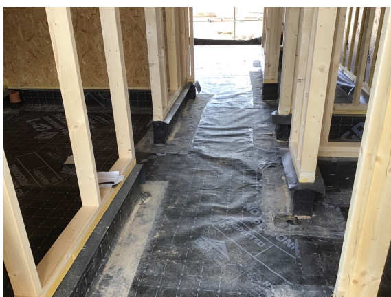
Overview of the Juta GP1 Gas Membrane that has been installed as an infill to plot 12.
