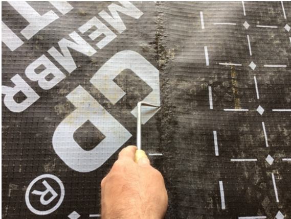
Probe testing all hand welded membrane laps in plot 13.
