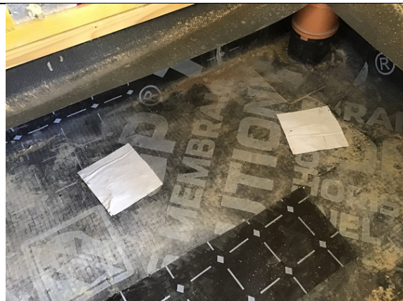
Patch repairs in plot 8 that were completed prior to our inspection by mb membranes.
