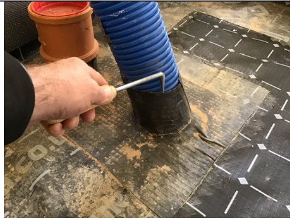
Probe testing a typical pipe penetration detail in plot 13.
