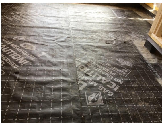
Typical hand welded membrane lap in plot 12.
