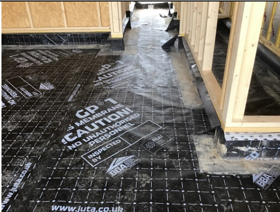
Overview of the Juta GP1 Gas Membrane that has been installed as an infill to plot 13.
