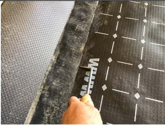
Probe testing all hand welded membrane laps in plot 12.
