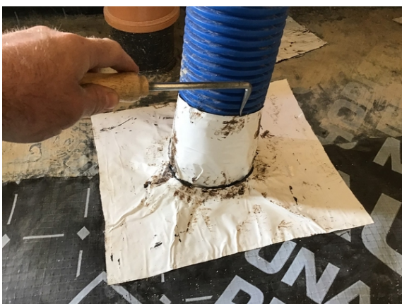
Probe testing a typical pipe penetration detail in plot 8.
