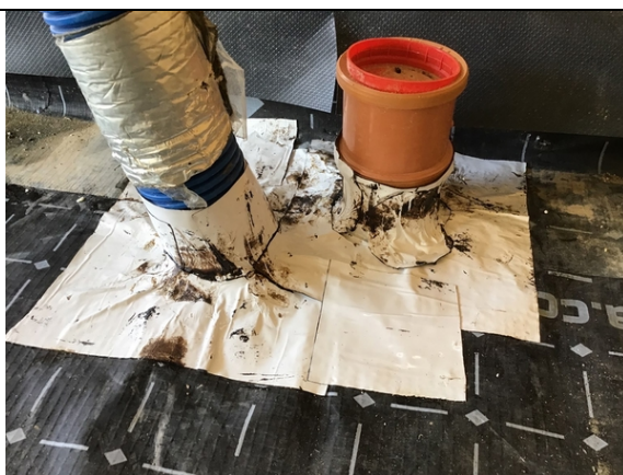
Typical double pipe penetration detailing in plot 10.
