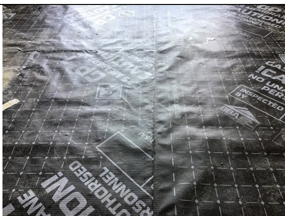
Overview of a typical hand welded membrane lap in plot 9.
