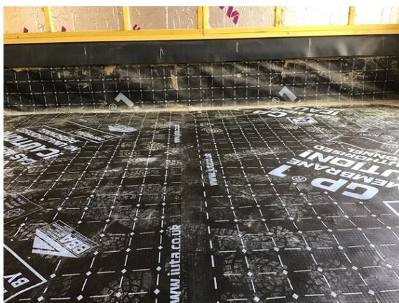
Overview of a typical hand welded membrane lap in plot 11.
