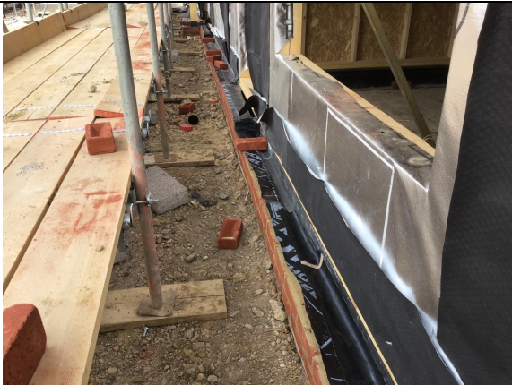
Overview of the extended Juta GP1 gas membrane that has been hand welded to the previously installed gas membrane which now spans the perimeter cavity wall across plots 3-5.
