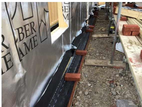
Overview of the extended Juta GP1 gas membrane that has been hand welded to the previously installed gas membrane which now spans the perimeter cavity wall across plots 6 & 7.
