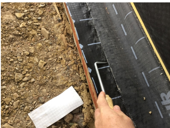
Probe testing the hand welded membrane lap in plot 4.
