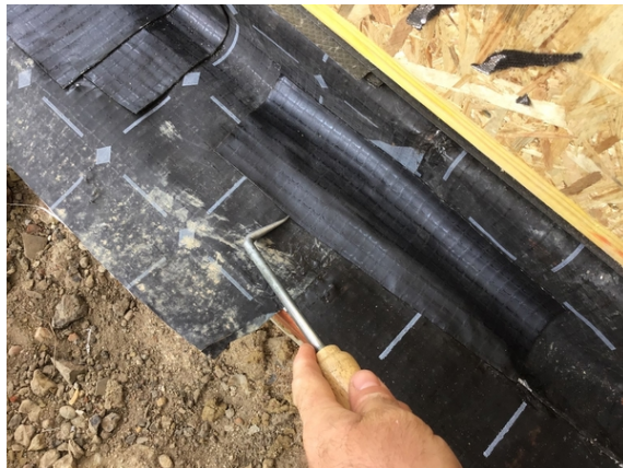
Probe testing the repaired weld defect in plot 5.
