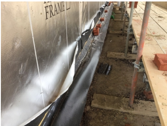
Overview of the extended Juta GP1 gas membrane that has been hand welded to the previously installed gas membrane which now spans the perimeter cavity wall across plot 11.
