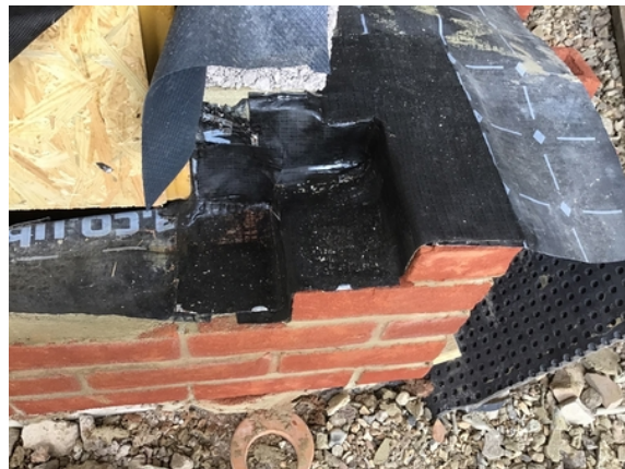
Detailing work to the extended perimeter membrane to plot 11.
