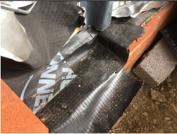
Door threshold detailing at the back of plot 13.
