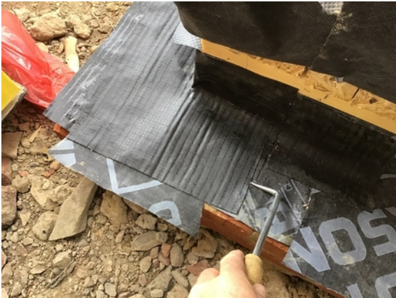
Probe testing the corner detailing in plots 14 & 15.
