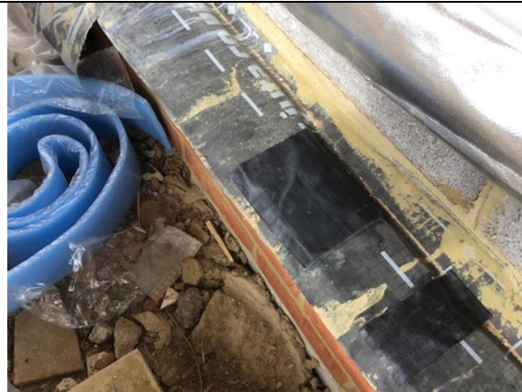
Repaired hole in membrane using Juta GP1 SAM to plot 10.
