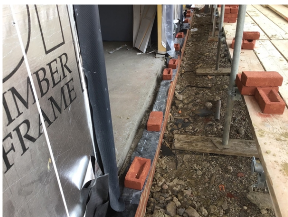
Overview of the extended membrane to the back elevation of plots 8 & 9.
