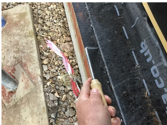
Probe testing the hand welded extended membrane around the perimeter of plot 9.
