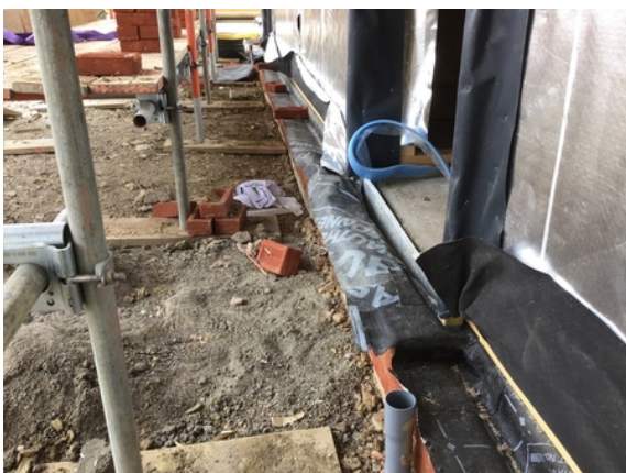
Overview of the extended Juta GP1 gas membrane that has been hand welded to the previously installed gas membrane which now spans the perimeter cavity wall across the front elevation of plots 12 & 13.
