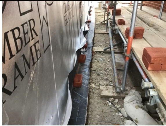
Overview of the extended Juta GP1 gas membrane that has been hand welded to the previously installed gas membrane which now spans the perimeter cavity wall across plots 14 & 15.
