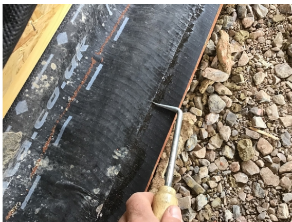
Probe testing all hand welded membrane laps on plot 10.
