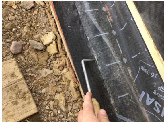
Probe testing all hand welded membrane laps in plots 14 & 15.
