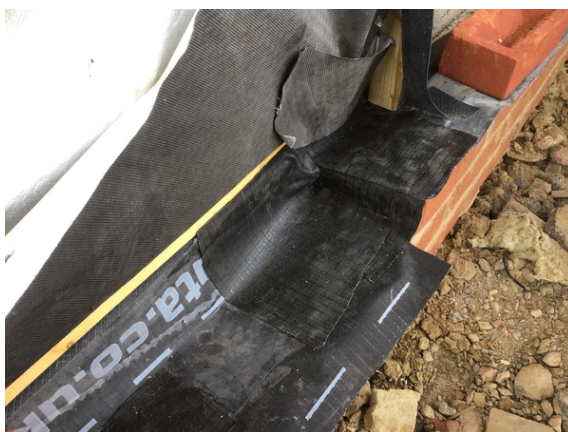
Detailing work to the back of the door threshold in plot 8.
