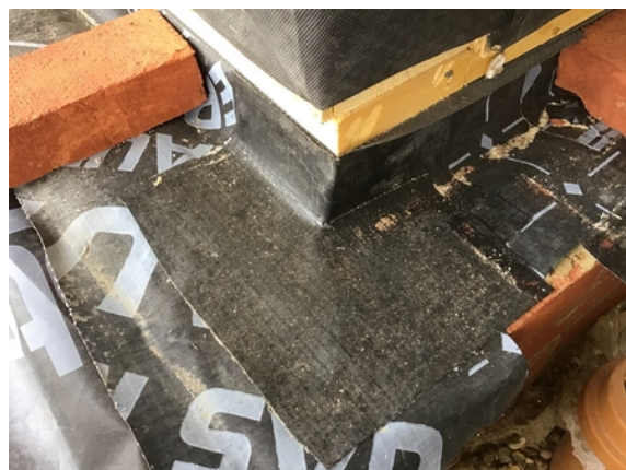
Corner detailing work to plot 12.
