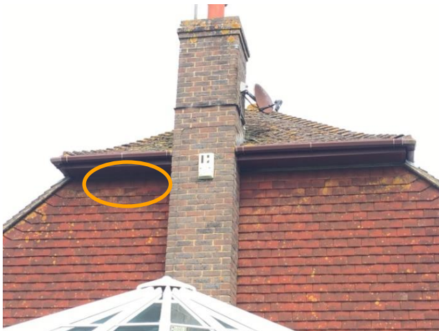
Survey 1 (B2): Point of emergence at 20.40 on 15 August (south elevation common pipistrelle x 1); and Survey 2 (B2): Point of re-entry at 05.32 on 12 September (south elevation common pipistrelle x 1)
