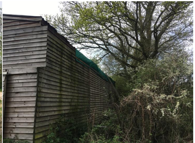
North face of the barn, sound construction
