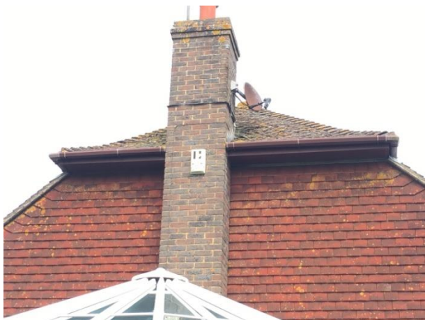
Many hanging tiles in good condition
