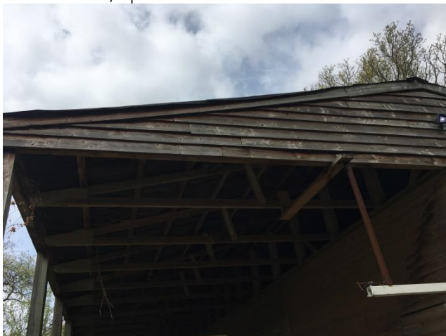
Exposed south face of roof void
