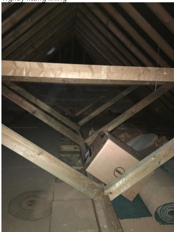
Internal flight space, some cross beams
