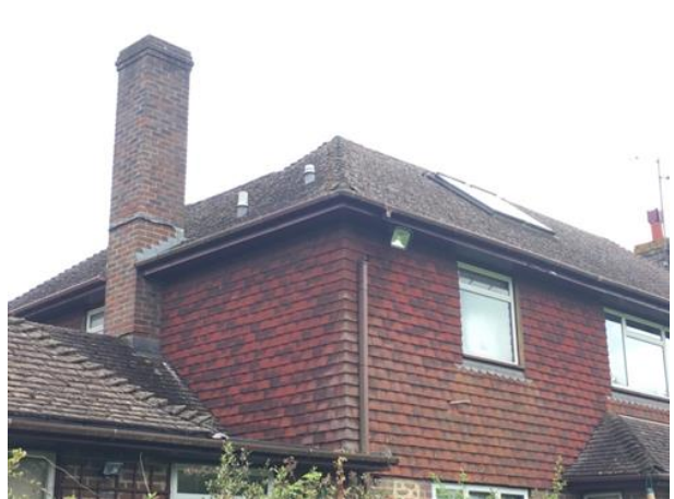
Tightly fitting lead flashing to the window, drainage pipe
