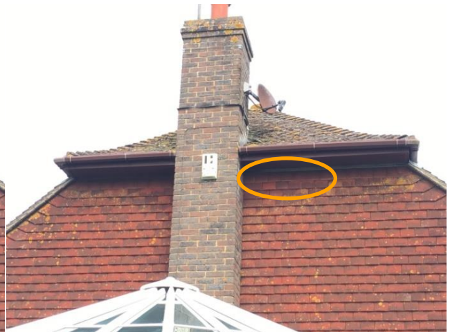
Survey 1 (B2): Point of emergence at 20.40 on 15 August (south elevation, common pipistrelle x 1).
