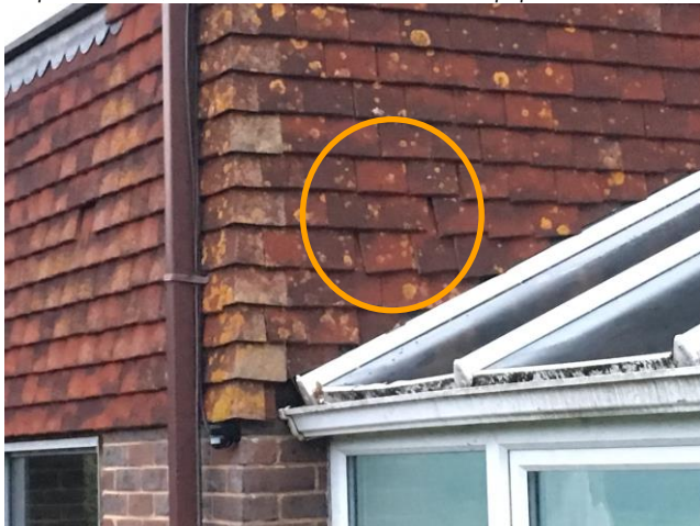
Survey 2 (B2): Point of re-entry at 05.50 on 29 August (south elevation, common pipistrelle x 1)
