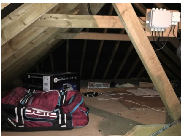
Rough timber beams
