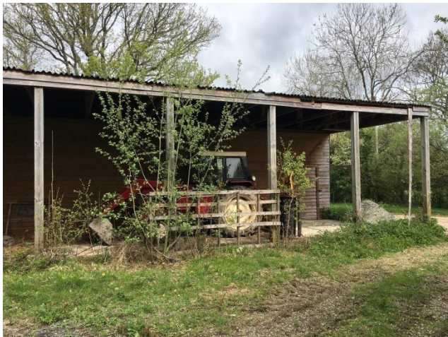
Exterior view, open sided to the south
