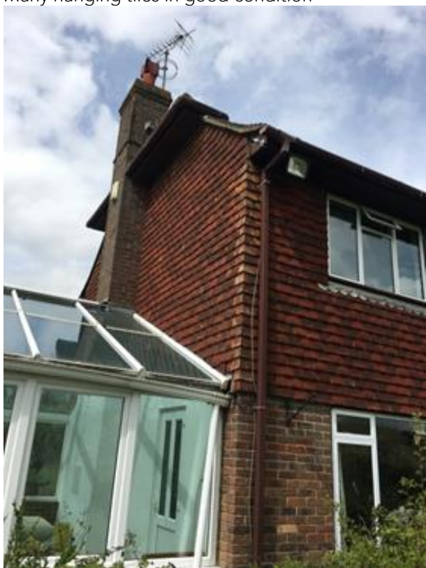
Brickwork in good condition
