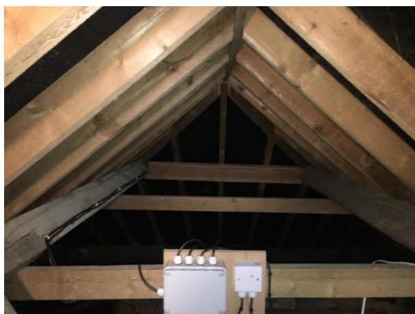
South east void
