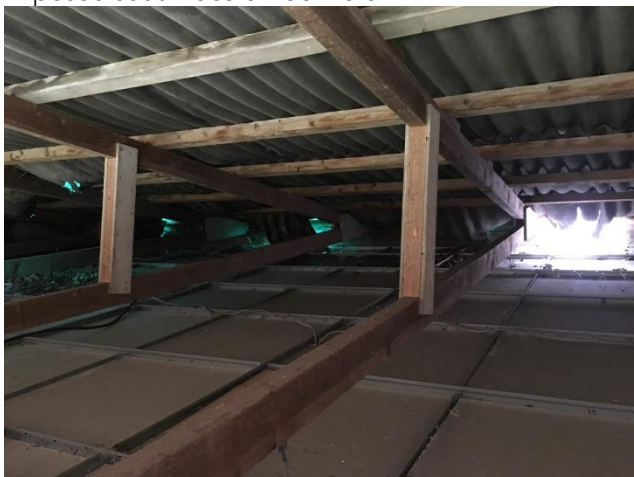
Exposed timbers, tightly fitting
