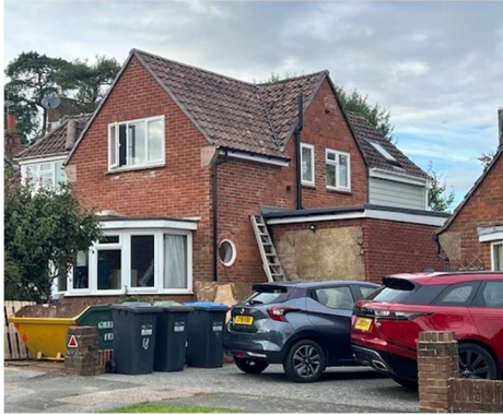
20 Highfield Drive (during building works)
