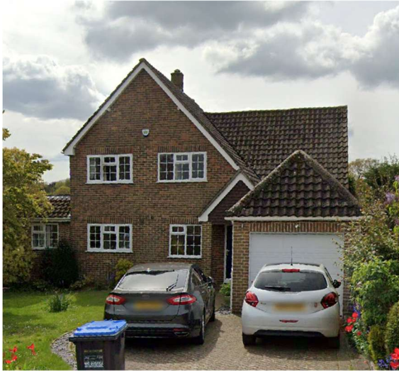
1 Highfield Drive, Neighbouring 2 storey property directly adjacent to the applicant site.
