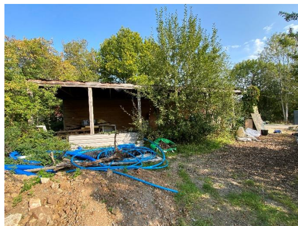
Photo 2: Southern elevation and vegetation (T5)
