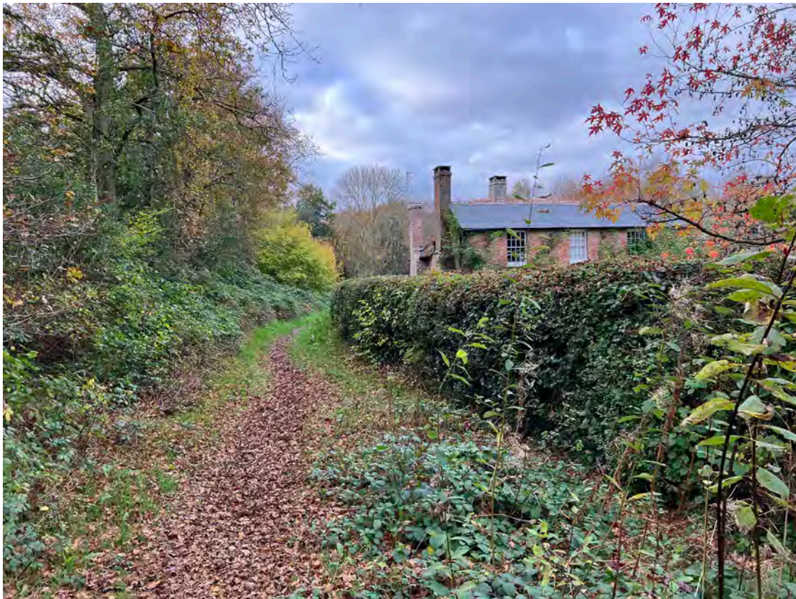
Plate 1: Grade II listed Westlands as viewed from the entrance to the PRow
