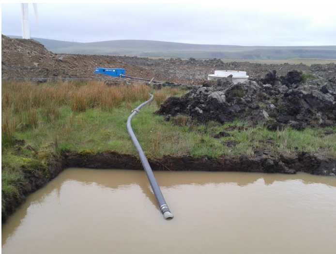
Figure 3: Typical 'Siltbuster' and settlement lagoon
