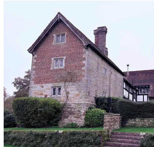
east gable of C15th range
