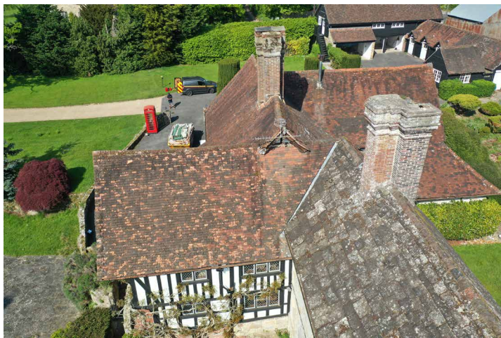
east elevation of C17th range
