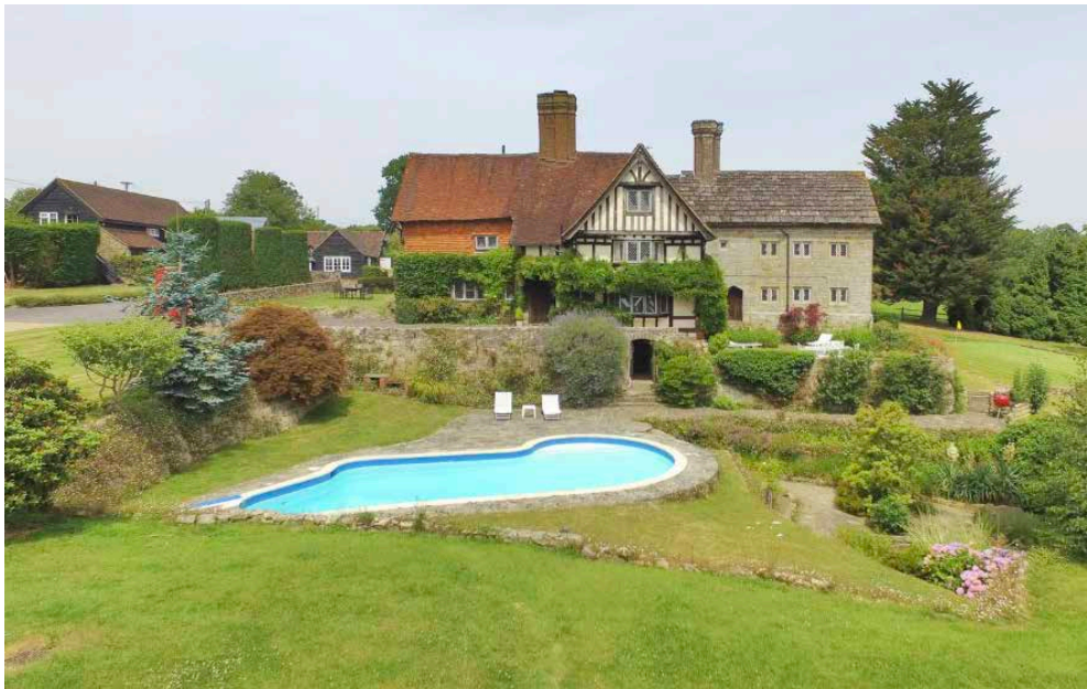
south elevation showing sunken pool terrace
