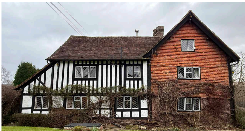
tile hanging to western elevation
