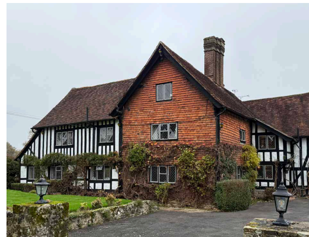
west elevation of C17th range
