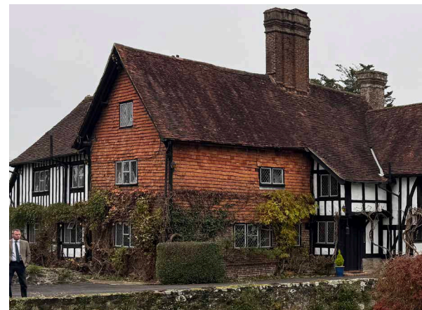
tile hanging southern elevation
