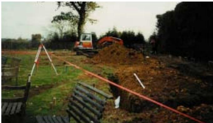
Image 3: Foundations for car park being created (Nymans Archives)
