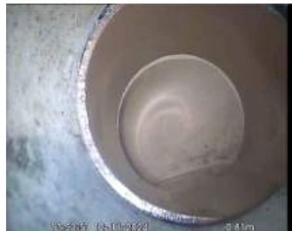
SVPX_6dc84003-04ba-4f4b-a2bc-ade636d85d44_20240725_095258_153.jpg, 00:00:43, 0.81 m Material changes to polyvinyl chloride
