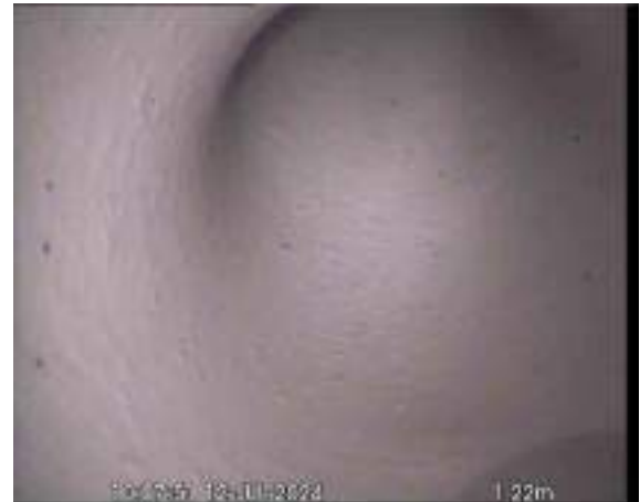
W_CX_e67dc308-cdad-4b4f-8f22-12bae3fd920a_20240725_090718_061.jpg, 00:00:43, 1.22 m Line deviates up, REST BEND
