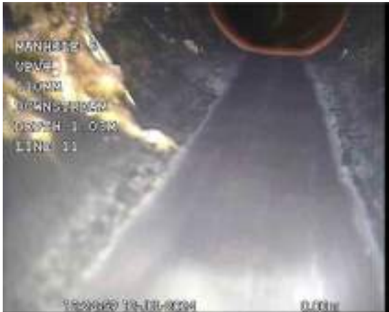
MH5X_bd5530c6-c89a-41b5-b33d-6c50f69b0280_20240725_094513_170.jpg, 00:00:29, 0.00 m Start node, manhole, reference: MANHOLE 5 (MH5)
