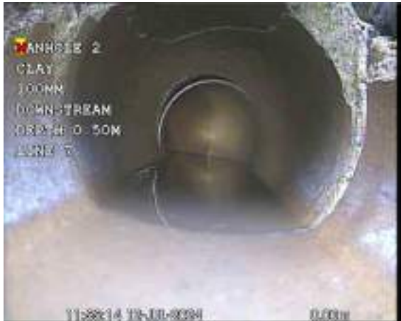
MH2X_c0af95fe-3efa-4666-b634-8d5993f92b03_20240725_092442_596.jpg, 00:00:28, 0.00 m Start node, manhole, reference: MANHOLE 2 (MH2)
