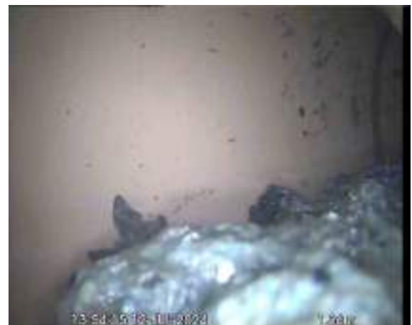
SVPX_7b6e8666-8fb9-44b5-8e1a-aafe5937a5df_20240725_095424_962.jpg, 00:01:07, 1.36 m Line deviates right
