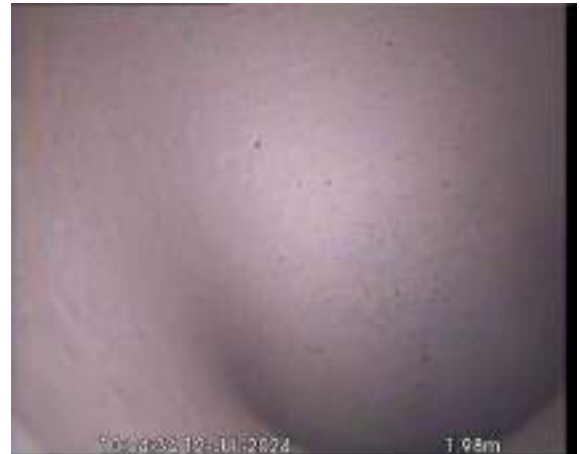
GULLYX_ea8e3b67-ae80-4672-8aa1-6d7696ac026d_20240725_090241_494.jpg, 00:01:10, 1.98 m Finish node, gully, reference: GULLY
