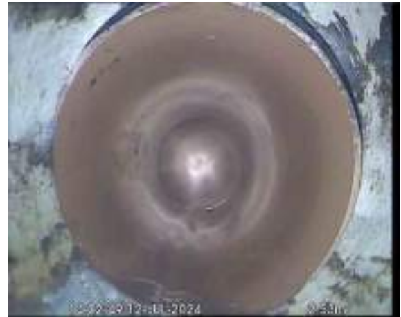
GULLYX_ae4d2037-60f9-42b2-acb6-9ea13a7fabb5_20240725_101346_335.jpg, 00:01:00, 2.53 m Size changes, new size(s), 110mm high
