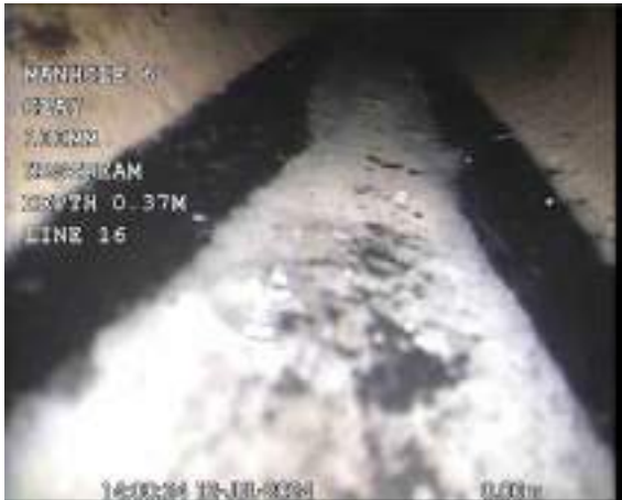
GULLYX_d2c349c2-d30e-442d-af5f-1d65018bdba0_20240725_101122_416.jpg, 00:00:17, 0.00 m Start node, manhole, reference: MANHOLE 6 (MH6)
