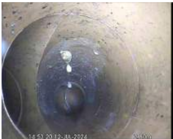
RWDPX_77261d0d-3cf9-4a7a-b815-6f3534f8d7cb_20240725_101701_695.jpg, 00:00:51, 2.80 m Junction at 9 o'clock, diameter: 110mm, RAINWATER DOWNPIPE (RWDP)
