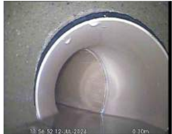
MH2X_2ccdc70-8b88-4cef-8827-dddf496b7eb6_20240725_092644_239.jpg, 00:00:56, 0.30 m Size changes, new size(s), 110mm high
