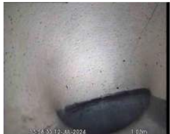
GULLYX_c67647b2-92e2-40c2-a9d7-fb213594d517_20240725_100025_314.jpg, 00:00:28, 1.03 m Finish node, gully, reference: GULLY
