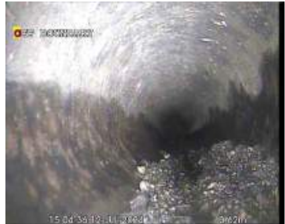
MANHOLEX_d574a494-dbda-46c8-9c0c-5e761cd3587d_20240725_102253_591.jpg, 00:01:02, 3.62 m General remark, **BOUNDARY POINT**
