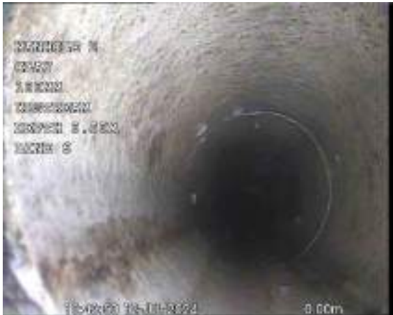
MH6X_83d29d4f-b593-490d-9743-99f8d8e575c1_20240725_091534_732.jpg, 00:00:16, 0.00 m Start node, manhole, reference: MANHOLE 2 (MH2)
