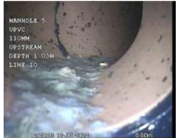
CAPPED OFFX_0b21e724-26bb-4d91-bb97-1640846d3795_20240725_094202_515.jpg, 00:00:37, 0.00 m Water level, 0% of the vertical dimension
