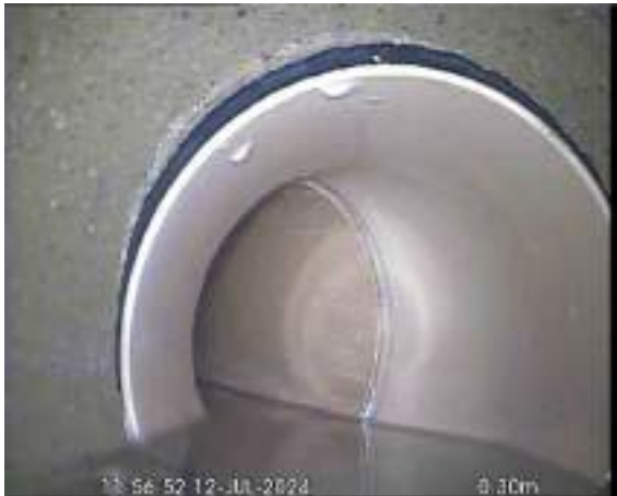
MH2X_b91b3937-c37a-452d-9c54-7c35945f681d_20240725_092617_600.jpg, 00:00:56, 0.30 m Material changes to polyvinyl chloride
