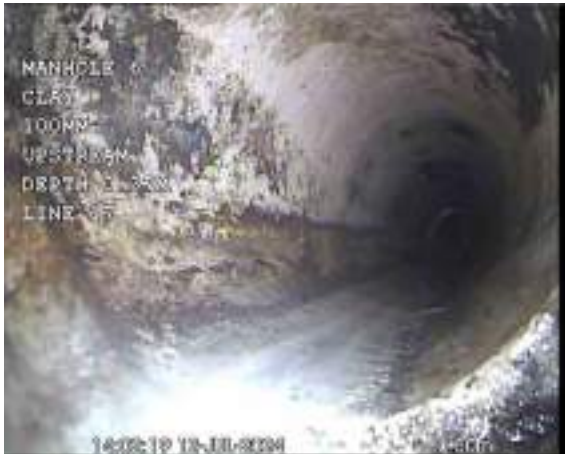
GULLYX_f6cd9efa-6157-4a0b-8db5-4b277d0362a3_20240725_101255_468.jpg, 00:00:30, 0.00 m Start node, manhole, reference: MANHOLE 6 (MH6)
