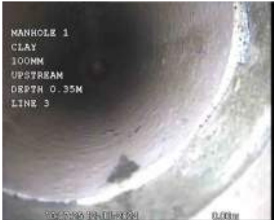
W_CX_aa28def7-6b17-4c5f-98d5-70f28f303849_20240725_090538_420.jpg, 00:00:17, 0.00 m Start node, manhole, reference: MANHOLE 1 (MH1)
