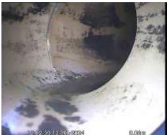
MH4X_047d0d34-fc87-401f-a4c3-3433783703f4_20240725_093918_923.jpg, 00:00:42, 0.06 m Line deviates right
