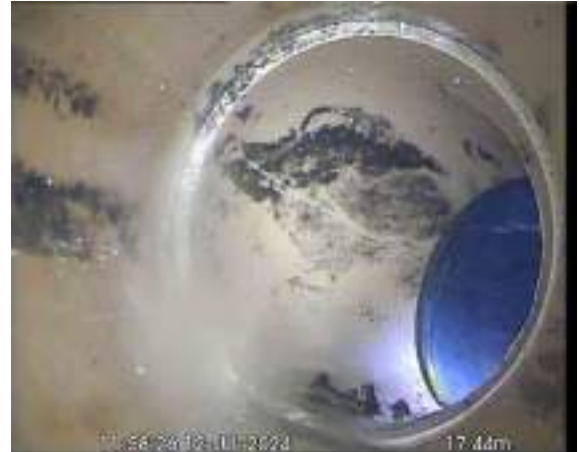
MH2X_ecbc01d4-5401-430c-a4cc-4e8128ef4209_20240725_093238_853.jpg, 00:02:20, 17.44 m Line deviates right
