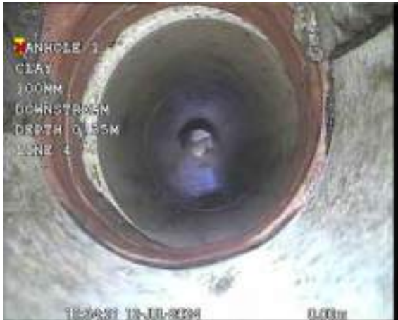
MH1X_8529fe95-596a-4229-ab69-a117d3ef1bdf_20240725_090923_983.jpg, 00:00:20, 0.00 m Start node, manhole, reference: MANHOLE 1 (MH1)
