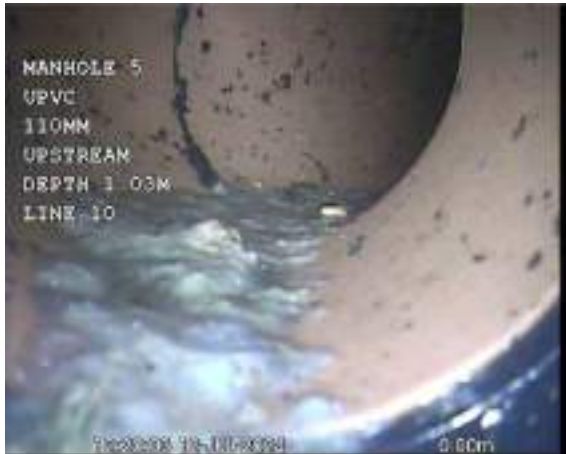
CAPPED OFFX_6c3871bb-4fd5-4855-bbb0-61d06810d0d7_20240725_094152_058.jpg, 00:00:37, 0.00 m Start node, manhole, reference: MANHOLE 5 (MH5)
