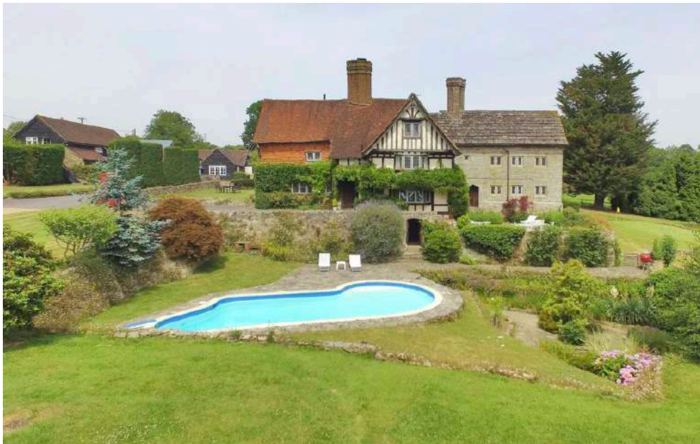
south elevation showing sunken pool terrace
