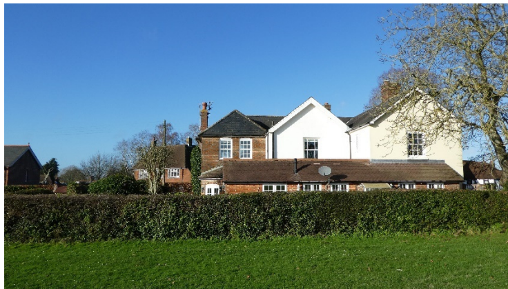
Figure 1 Victoria Cottages & Outbuilding from Horsted Keynes Recreational Ground
