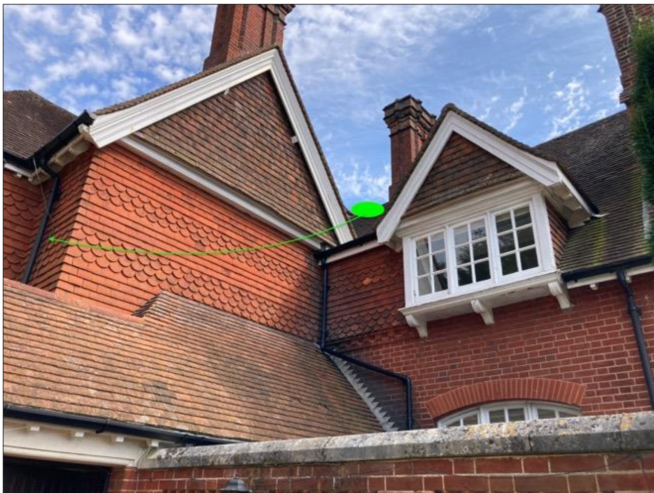
Figure 15. View of the western aspect of the site with the approximate emergence location and flight line of the soprano pipistrelle recorded at 21:33 on survey 2.
