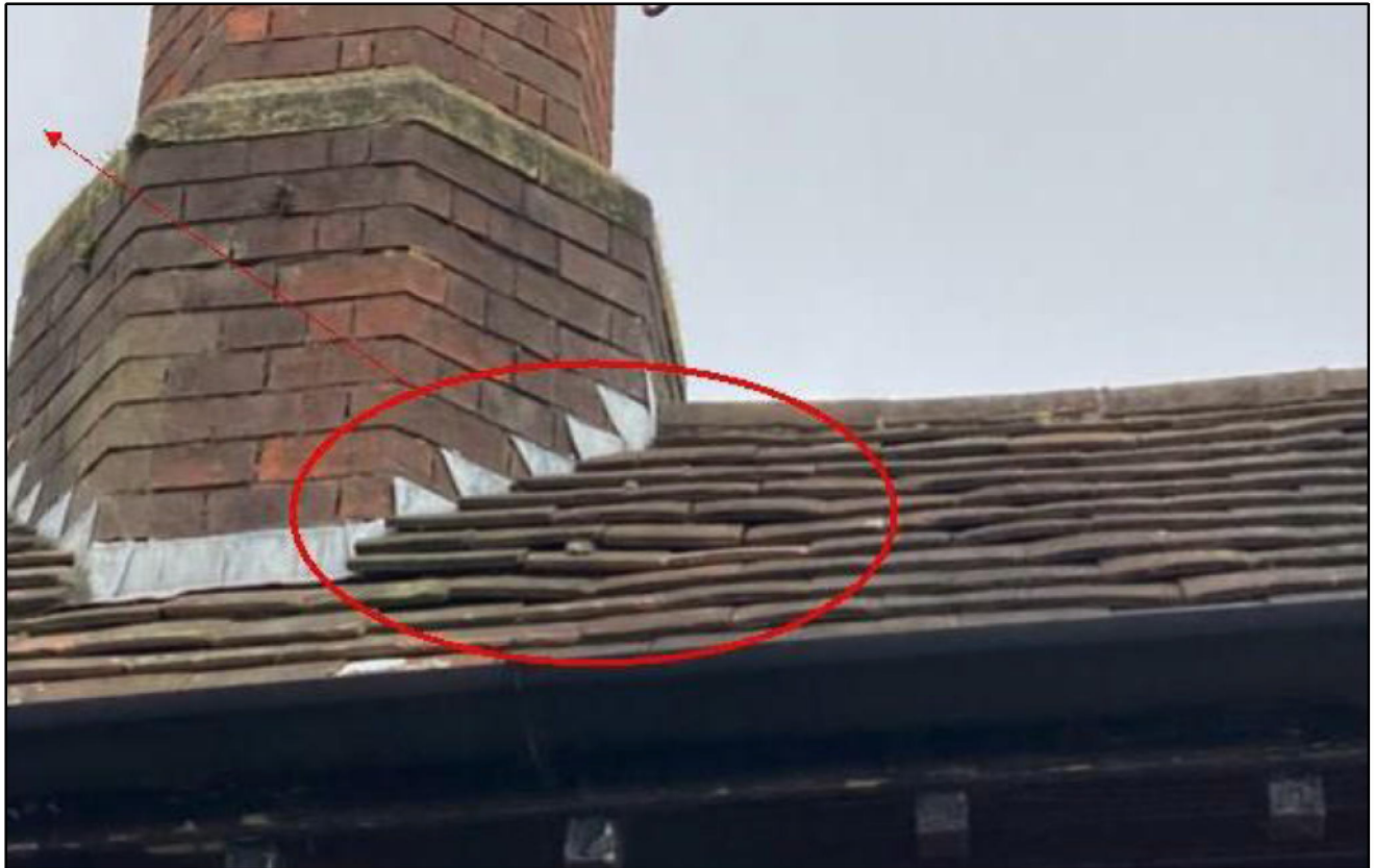
Figure 10. An image of the eastern aspect of North Lodge, showing the approximate emergence location of one common pipistrelle bat (red arrow) from beneath roof tiles to the right of the chimney stack (adjacent to Tower 1), and its flight path during the survey on the 21 st July 2025 indicated.
