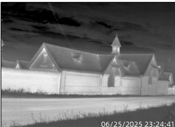
Photograph 4. An image of the thermal vision viewpoint from the first survey of North Lodge (25/06/25).
