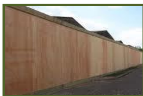
Wooden Hoarding, painted Kew Green
