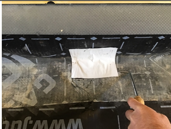
Probe testing a patch repair in plot 4.
