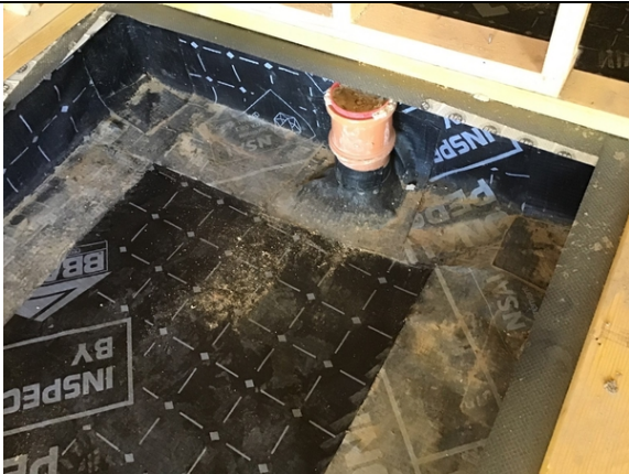
Overview of a pipe penetration detailing that has been inspected on a previous visit in plot 3.
