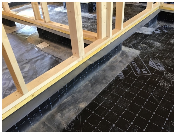
Overview of the internal wall membrane that has been hand welded to the infilled membrane in plot 4.
