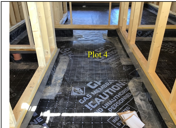
Overview of the Juta GP1 gas membrane installed as an infill in plot 4.
