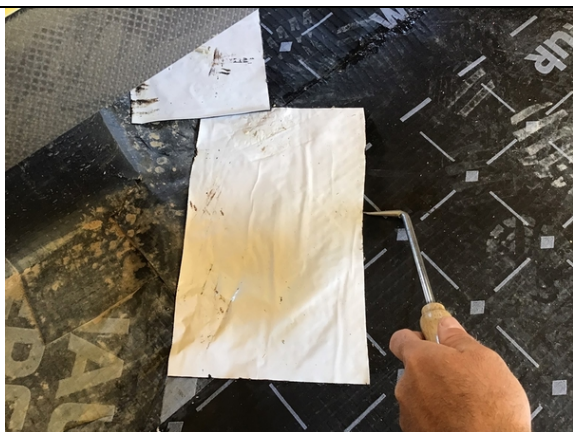
Probe testing a patch repair in plot 5.
