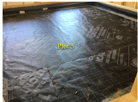
Overview of the Juta GP1 gas membrane installed as an infill in plot 5.
