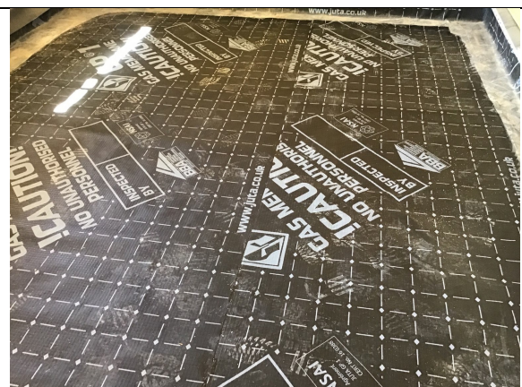
Overview of a hand welded membrane lap in plot 3.
