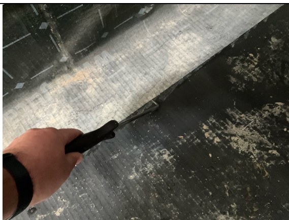
Plot 6. Probe testing along perimeter edge hand welded lap joints.
