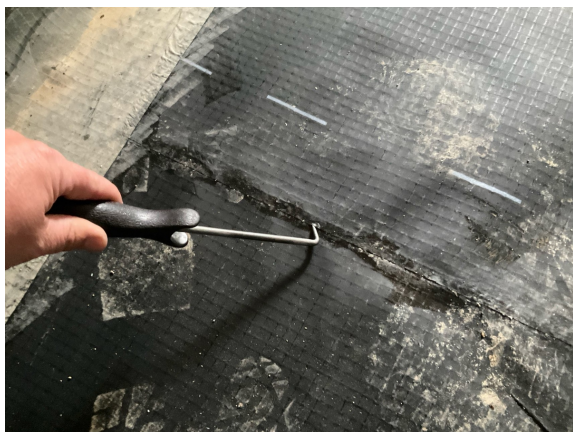
Plot 6. Probe testing along hand welded membrane lap joints.
