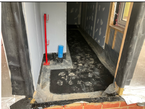
Plot 6. Overview of the Infill installation to Stair core only.
