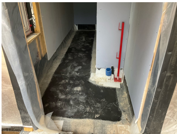
Plot 15. Overview of the Infill installation to Stair core only.
