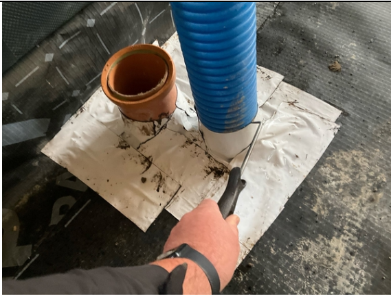
Plot 34. Probe testing to pipe penetration details.
