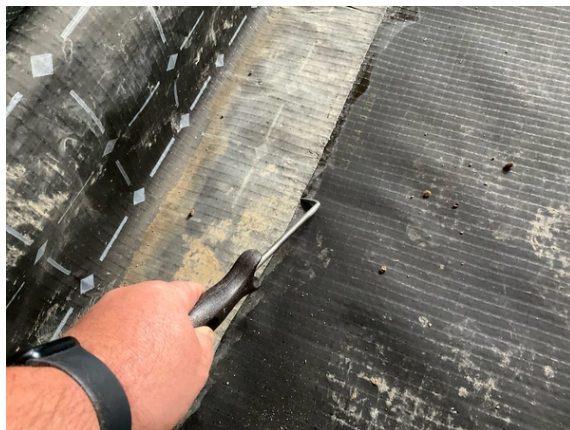
Plot 34. Probe testing along perimeter edge hand welded lap joints.
