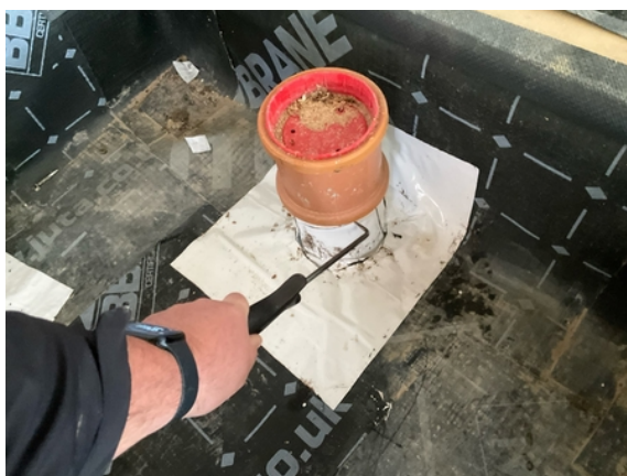
Plot 35. Probe testing to pipe penetration details.
