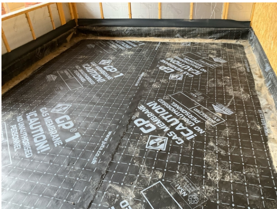
Plot 34. Overview of the Infill installation using Juta GP1.
