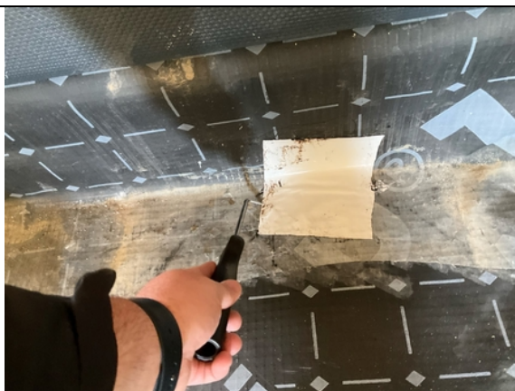
Plot 35. Probe testing to installers own CQA patch repairs.
