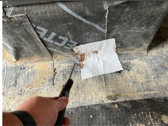
Plot 34. Probe testing to installers own CQA patch repairs.
