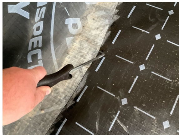
Plot 35. Probe testing along perimeter edge hand welded lap joints.
