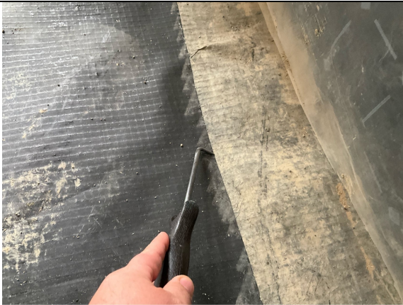
Plot 15. Probe testing along perimeter edge hand welded membrane lap joints.
