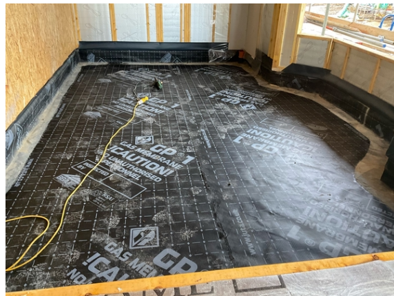
Plot 35. Overview of the Infill installation using Juta GP1.
