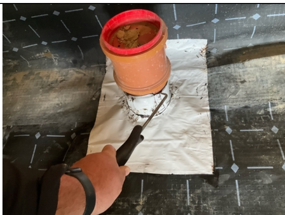
Plot 35. Probe testing to pipe penetration details.
