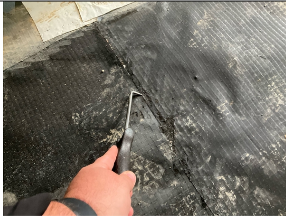
Plot 15. Probe testing along hand welded lap joints.
