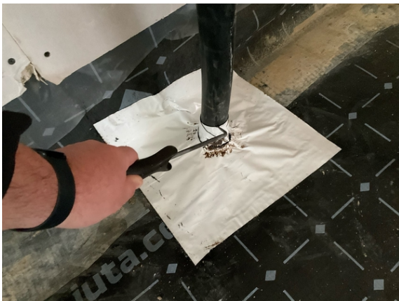
Plot 34. Probe testing to pipe penetration details.
