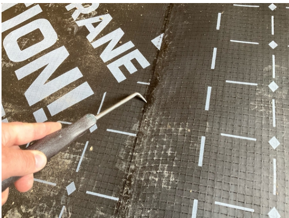
Plot 34. Probe testing along hand welded membrane lap joints.
