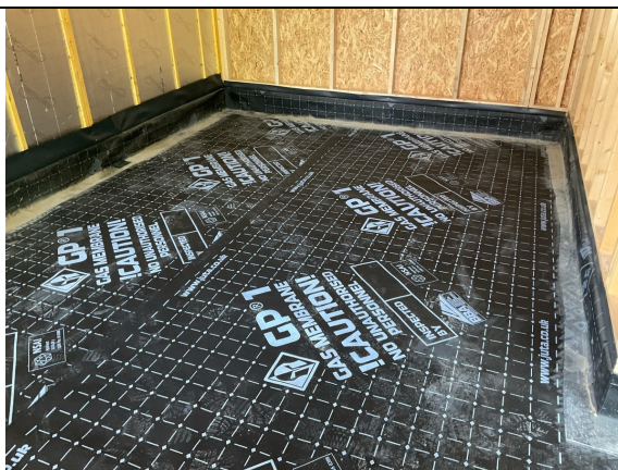
Overview of the infill installation using Juta GP1.
