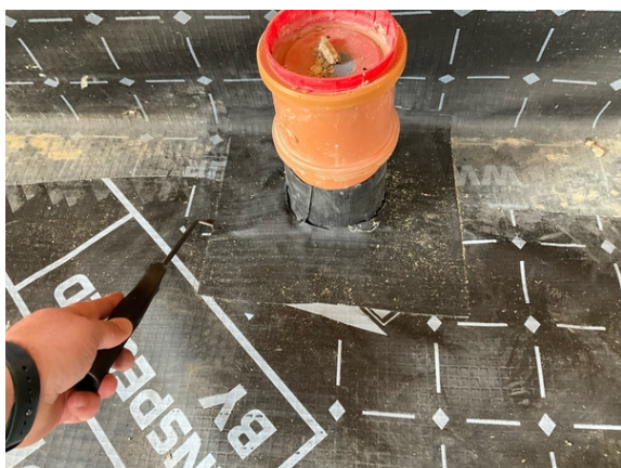
Probe testing to pipe penetration details.
