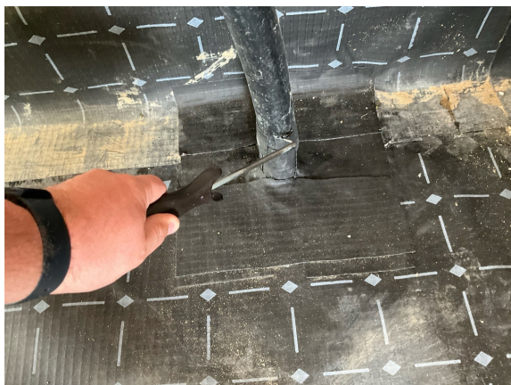
Probe testing to pipe penetration details.
