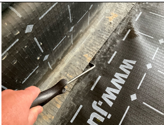
Probe testing along perimeter edge hand welded membrane lap joints.
