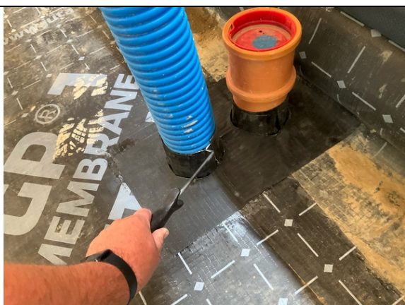
Probe testing to pipe penetration details.
