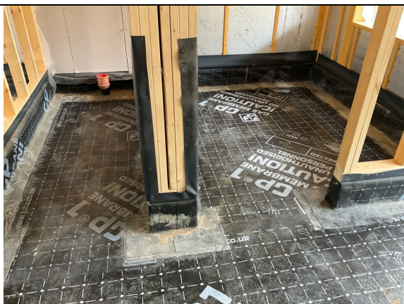
Overview of the infill installation using Juta GP1.
