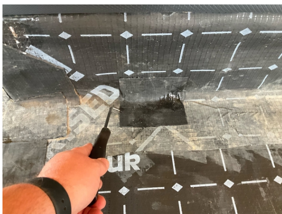
Probe testing to installers own CQA patch repairs.
