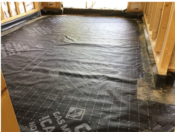
Overview of the Juta GP1 gas membrane that has been installed as an infill in plot 36.
