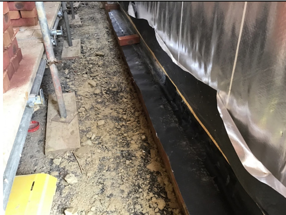
Overview of the extended membrane installation to close off the perimeter cavity on plot 34.
