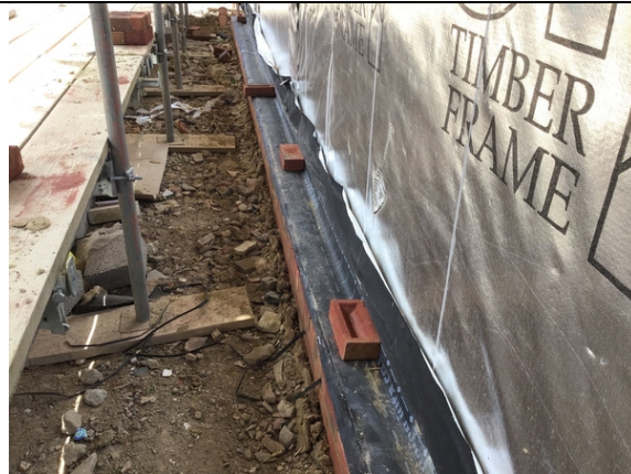
Overview of the extended membrane installation to close off the perimeter cavity on plot 36.
