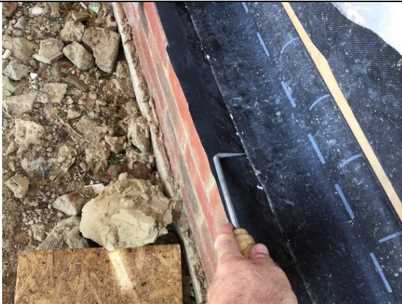
Probe testing the extended hand welded membrane lap around the perimeter of plot 33.
