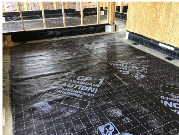
Overview of the Juta GP1 gas membrane that has been installed as an infill to plot 37.
