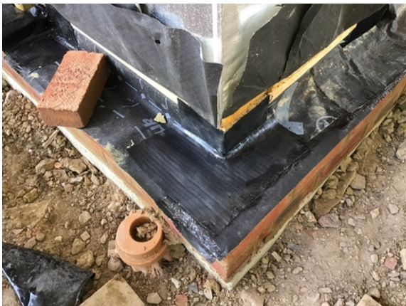
Typical corner detailing around the perimeter of plot 36.
