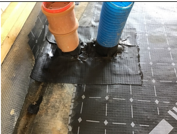
Typical double pipe penetration detailing in plot 36.
