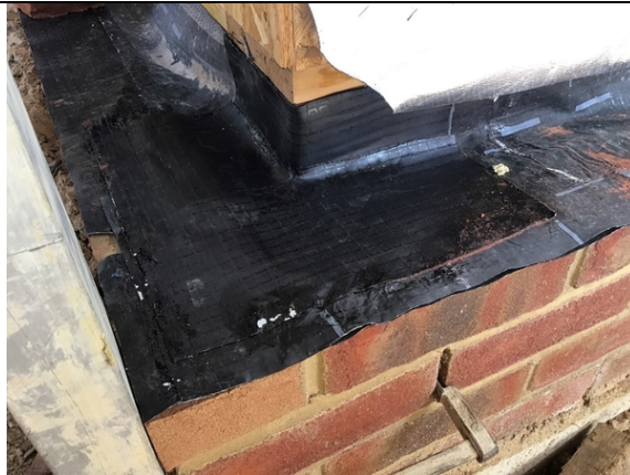
Corner detailing to plot 33.
