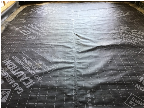
Overview of a typical hand welded membrane lap in plot 36.
