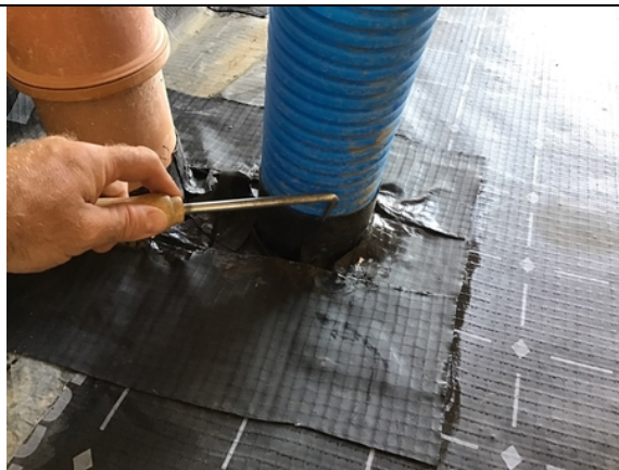
Probe testing a typical pipe penetration detail in plot 36.
