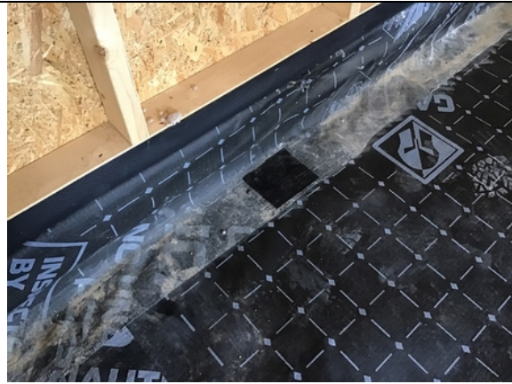
MB Membranes carried out there own CQA repairs prior to our inspection.
