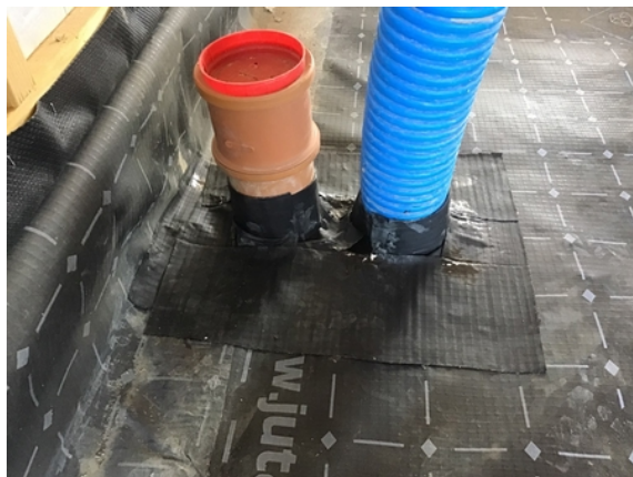
Typical double pipe penetration detailing in plot 37.
