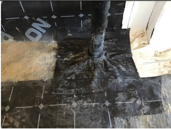
Pipe penetration detailing in plot 37.
