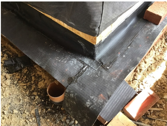
Corner detailing to plot 34.
