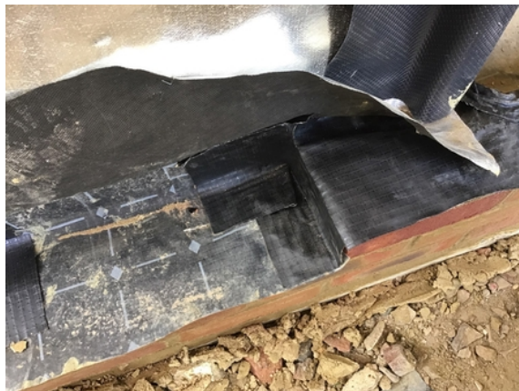
External door threshold detailing in plot 36.
