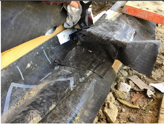
External door threshold detailing in plot 37.
