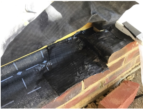
External door threshold detailing in plot 35.
