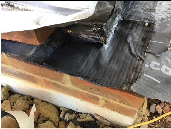
External corner detailing in plot 35.
