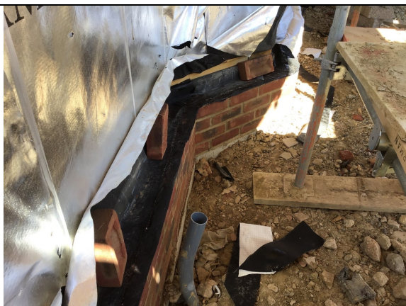
Overview of the extended membrane installation to close off the perimeter cavity on plot 35.
