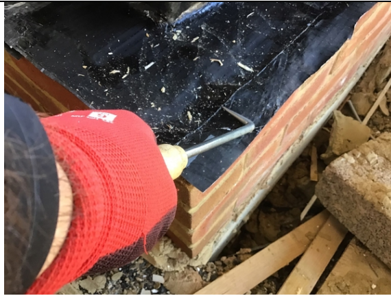
Probe testing a corner detail in plot 35.
