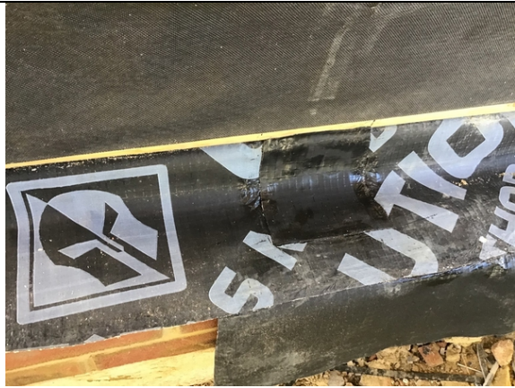
Patch repair using Juta GP1 SAM to the damaged perimeter membrane on plot 37.
