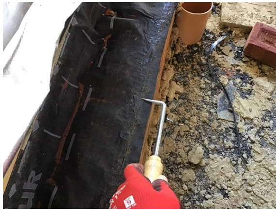
Probe testing a hand welded membrane lap in plot 35.
