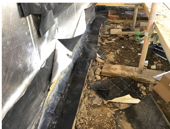
Overview of the extended membrane installation to close off the perimeter cavity on plot 37.
