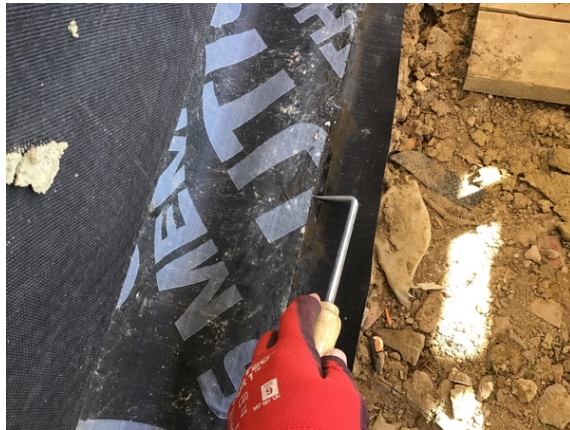
Probe testing a hand welded membrane lap in plot 37.
