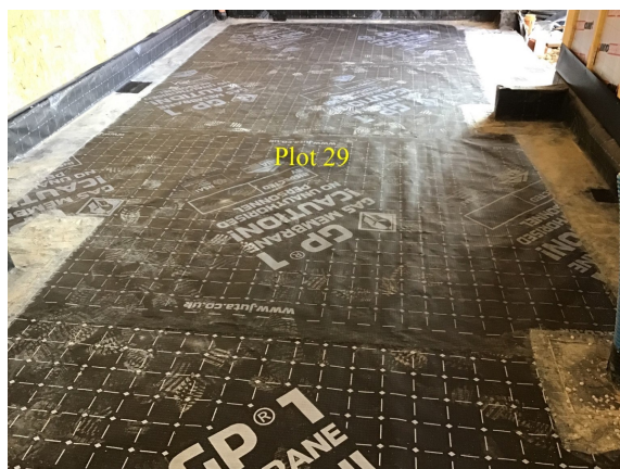
Overview of the Juta GP1 Gas Membrane that has been installed as an infill to plot 29.
