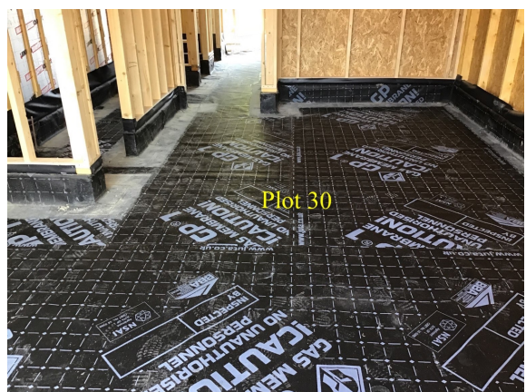
Overview of the Juta GP1 Gas Membrane that has been installed as an infill to plot 30.
