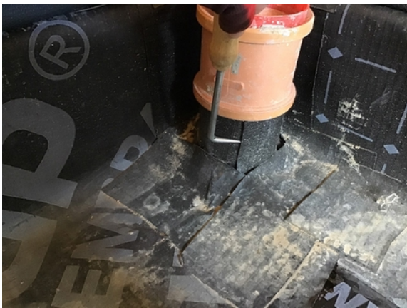
Probe testing a typical pipe penetration detail in plot 31.
