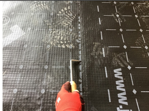
Probe testing a typical hand welded membrane lap in plot 29.
