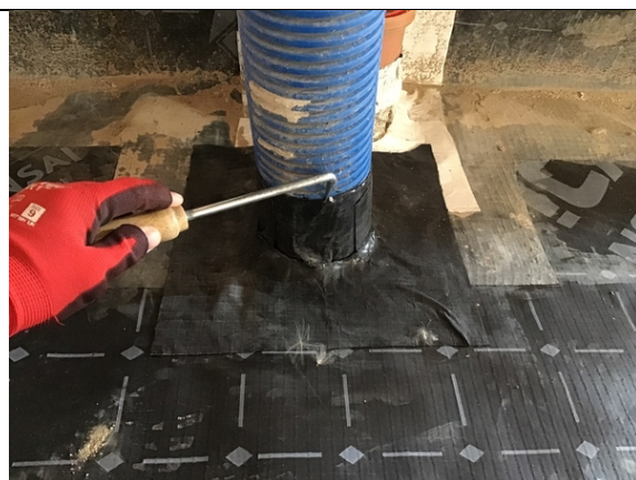
Probe testing a typical pipe penetration detail in plot 14.
