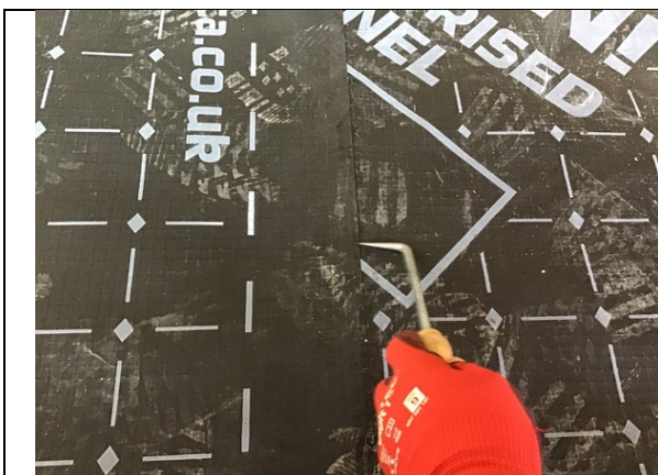
Probe testing a typical hand welded membrane lap in plot 14.
