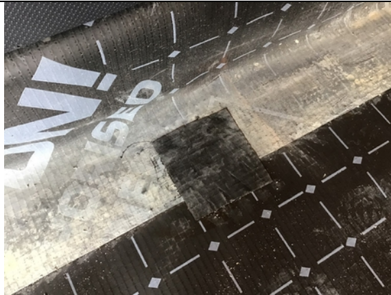
Patch repair using Juta GP1 SAM a that was completed by mb membranes prior to our inspection in plot 31.
