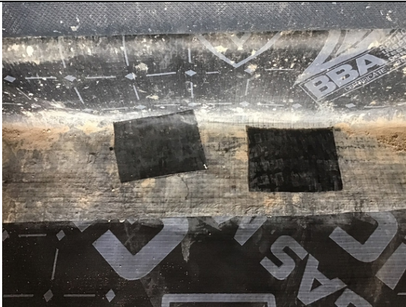
Patch repairs that were carried out by mb membranes prior to our inspection in plot 14.
