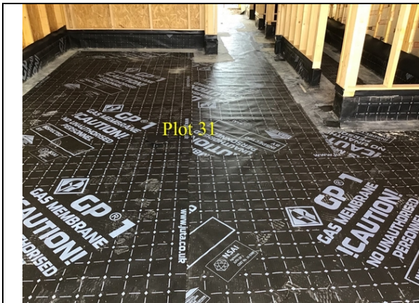
Overview of the Juta GP1 Gas Membrane that has been installed as an infill to plot 31.
