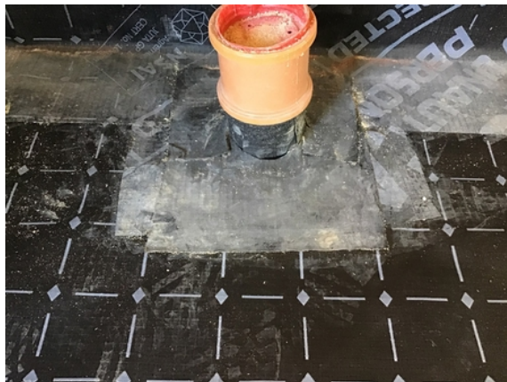
Pipe penetration detailing in plot 32.
