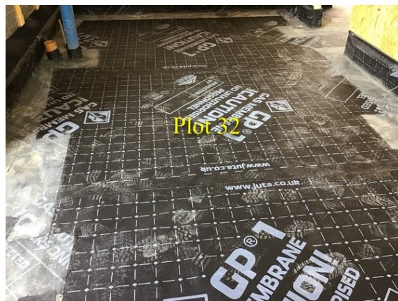
Overview of the Juta GP1 Gas Membrane that has been installed as an infill to plot 32.
