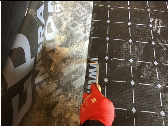
Probe testing a typical hand welded membrane lap in plot 31.
