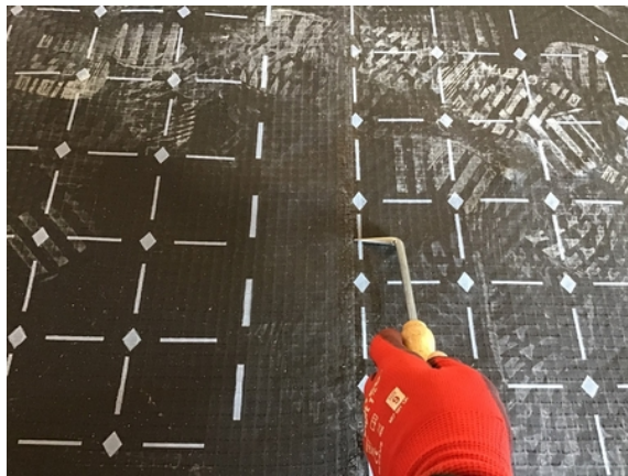
Probe testing a hand welded membrane lap in plot 32.
