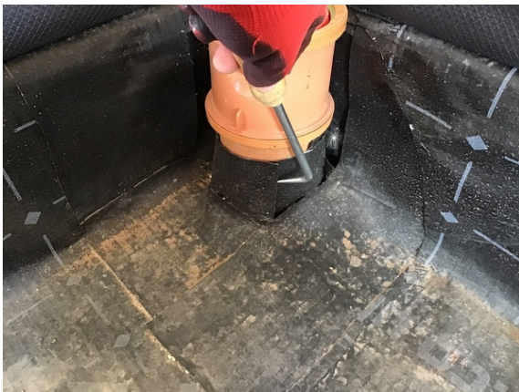
Pipe penetration detailing in plot 29.
