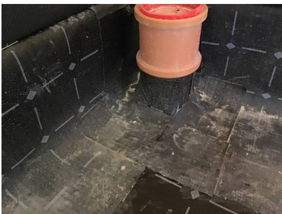
Typical pipe penetration detailing in plot 30.
