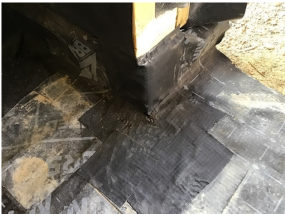
Door threshold detailing in plot 32.
