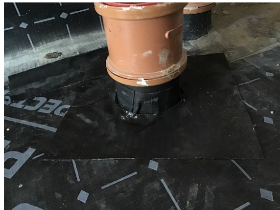
Pipe penetration detailing in plots 6 & 7.
