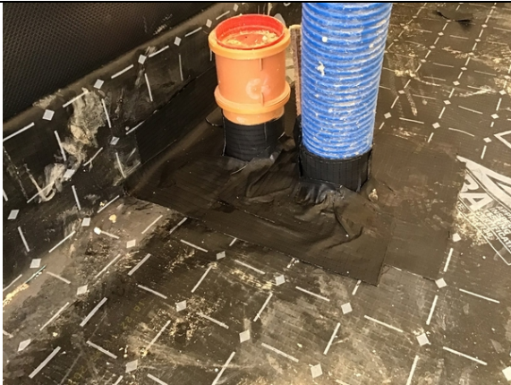
Typical double pipe penetration detailing in plot 27.
