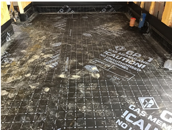
Overview of the Juta GP1 Gas Membrane that has been installed as an infill to plot 28.
