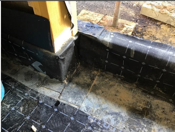
Door threshold detailing in plot 28.
