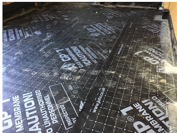
Overview of the Juta GP1 Gas Membrane that has been installed as an infill to plots 6 & 7.
