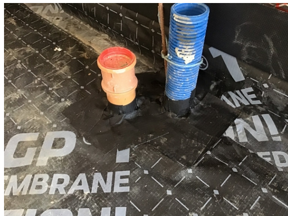
Typical double pipe penetration detailing in plot 28.
