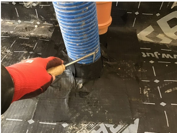
Probe testing a typical pipe penetration detail in plot 27.
