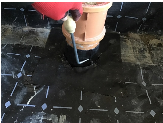
Probe testing a pipe penetration detail in plot 28.
