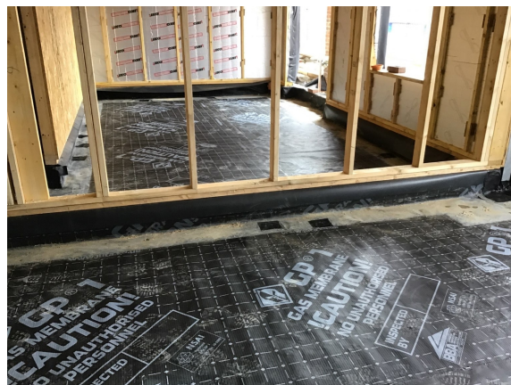
Overview of the Juta GP1 Gas Membrane that has been installed as an infill to plot 25.
