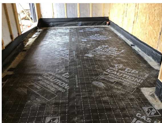
Overview of the Juta GP1 Gas Membrane that has been installed as an infill to plot 26.
