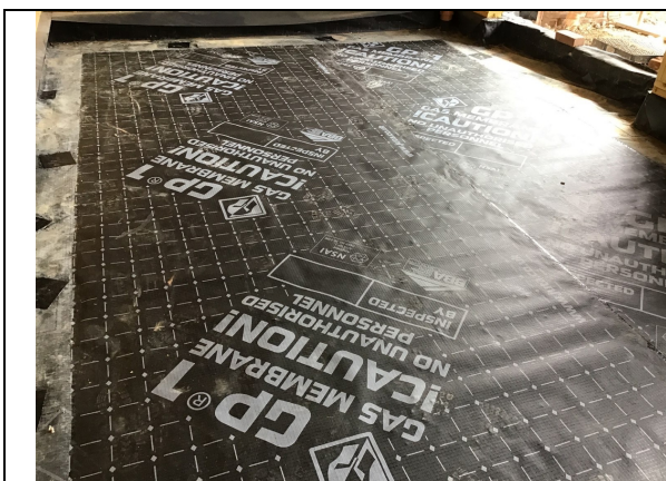
Overview of the Juta GP1 Gas Membrane that has been installed as an infill to plot 25.
