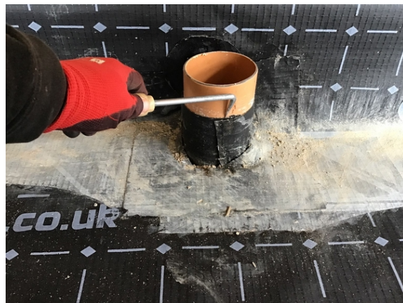
Probe testing a pipe penetration detail in plot 26.
