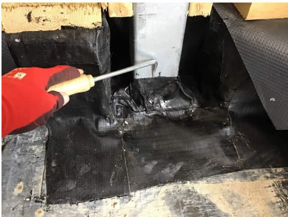
Probe testing a steel stanchion detail in plot 25.
