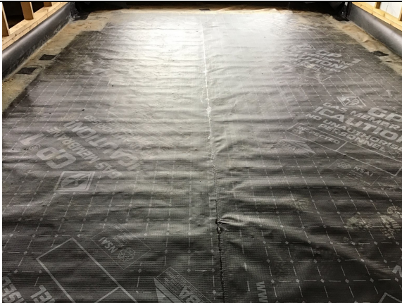
Overview of a hand welded membrane lap in plot 25.
