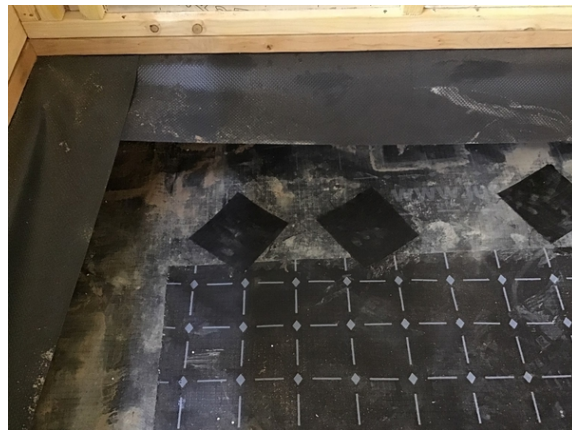
Patch repair detailing in plot 25 that was completed by mb membranes prior to our inspection.
