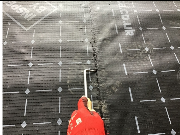
Probe testing a hand welded membrane lap in plot 25.
