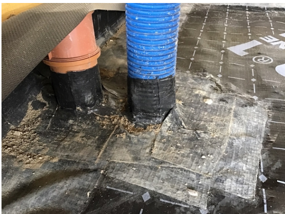
Typical pipe penetration detailing in plot 25.
