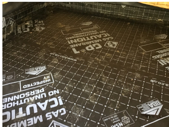
Plot 24 infill installation overview.
