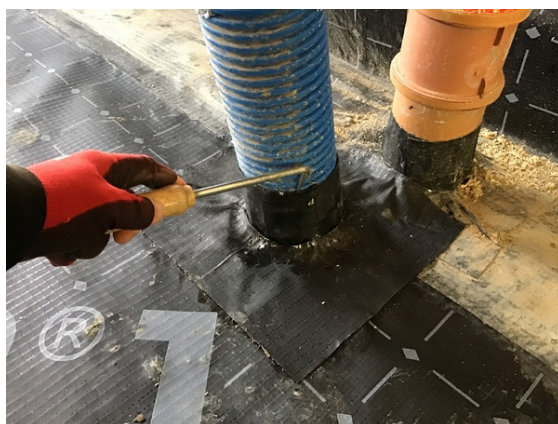
Plot 24 pipe penetration detail testing.
