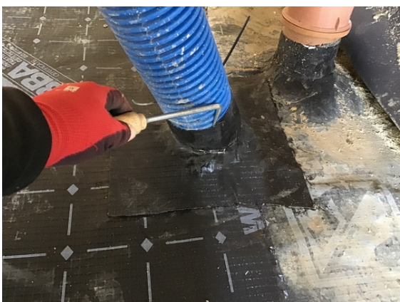
Plot 23 pipe penetration detail testing.
