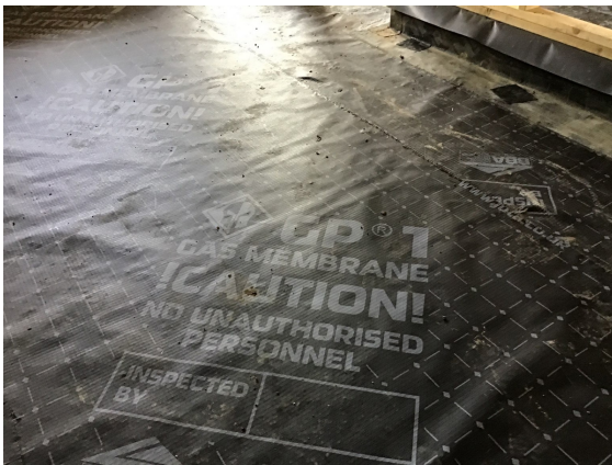
Plot 23 infill installation overview.
