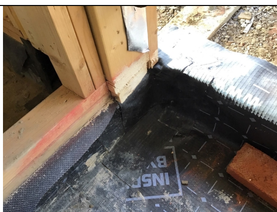
Plot 22 door threshold detailing.
