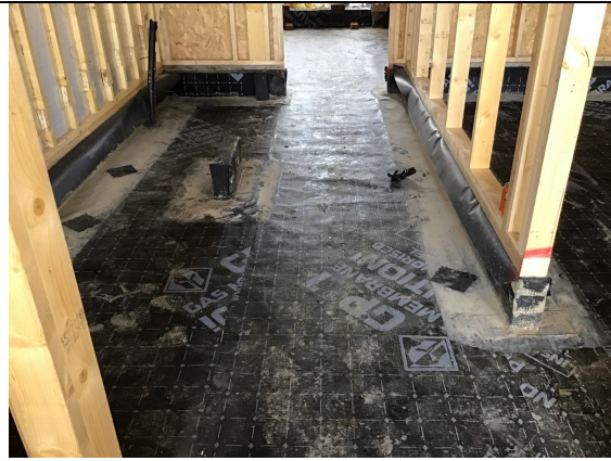
Plot 23 infill installation overview.
