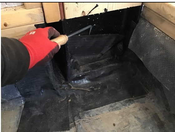
Plot 23 steel stanchion detail testing.
