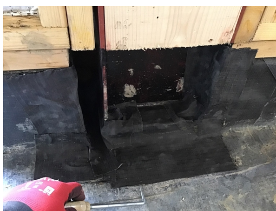
Plot 22 steel stanchion detail testing.
