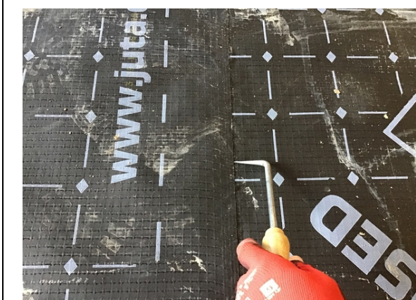
Plot 22 hand welded membrane lap testing.
