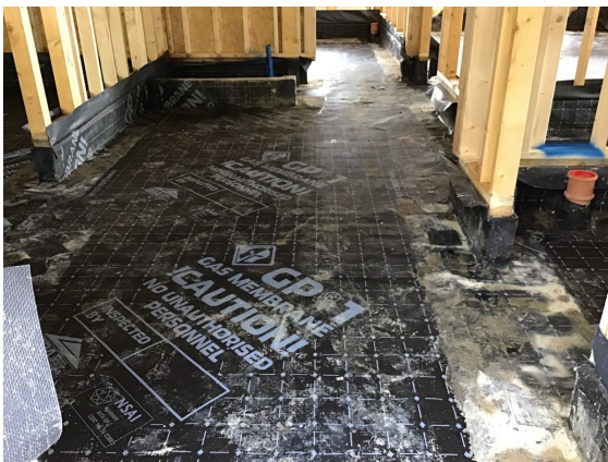
Plot 24 infill installation overview.
