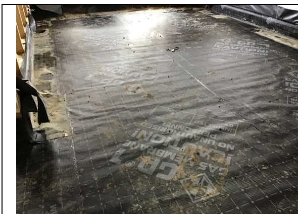
Plot 24 infill installation overview.
