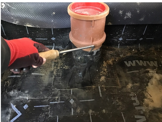
Plot 24 pipe penetration detail testing.
