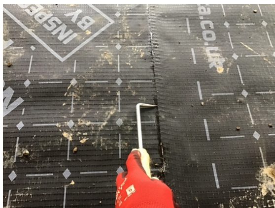
Plot 24 hand welded membrane lap testing.
