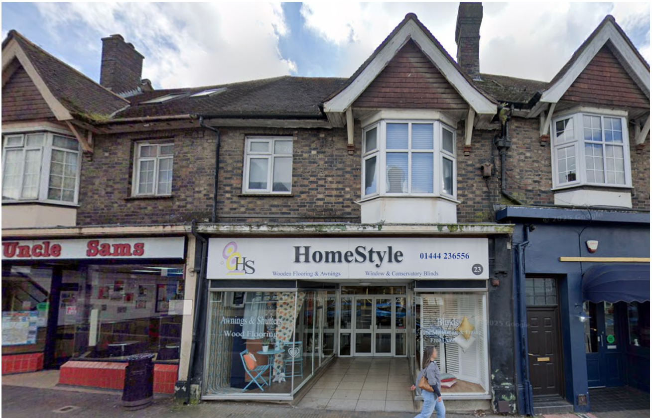
Figure 1: Street view photograph showing the existing shopfront at 23 Station Road, Burgess Hill, prior to the proposed entrance door repositioning. Source: Google Street View
