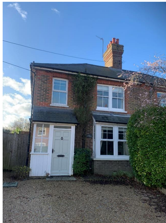
01 – View of front of property. Main chimney stack taking visual dominance.
