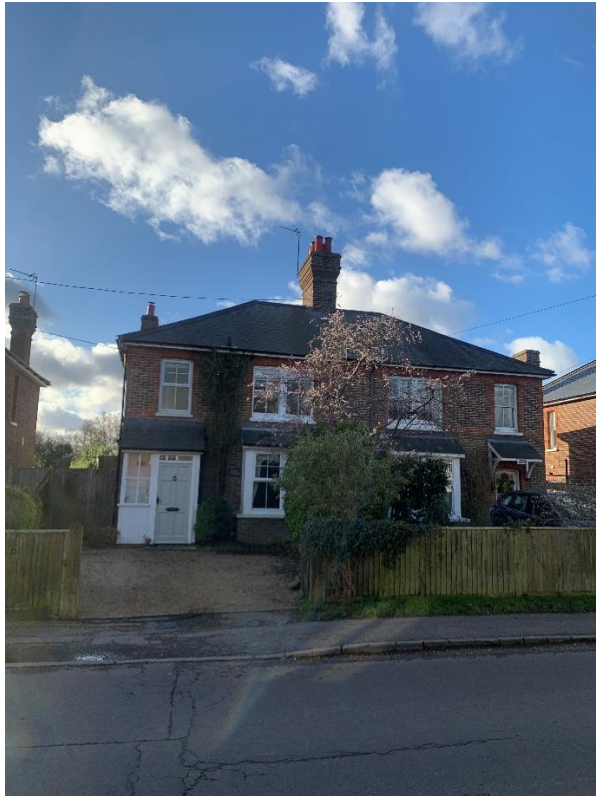
02 – Front of property taken from across road. Side chimney just showing.
