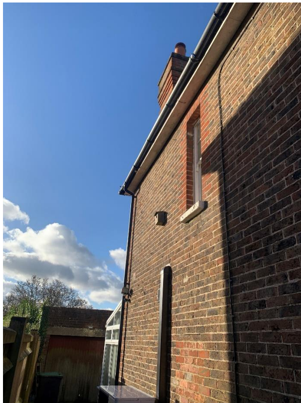
03 – View of side elevation with chimney under application visible above eaves line.
