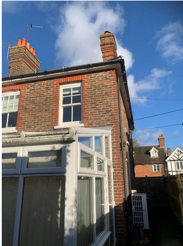
04 – View from rear south corner – chimney to be removed is on right hand side.
