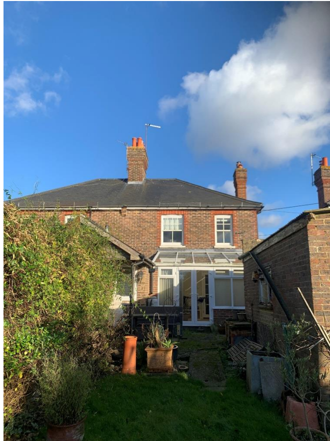
06 – View from rear of property. Note adjoining neighbour's secondary chimney is already removed.
