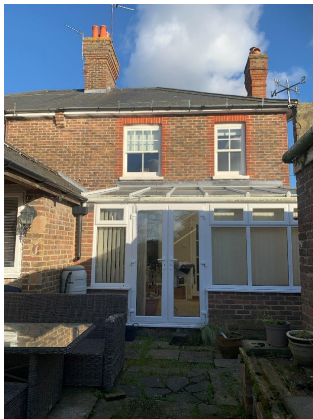
05 – View from rear of property – chimney to be removed is on right hand side.
