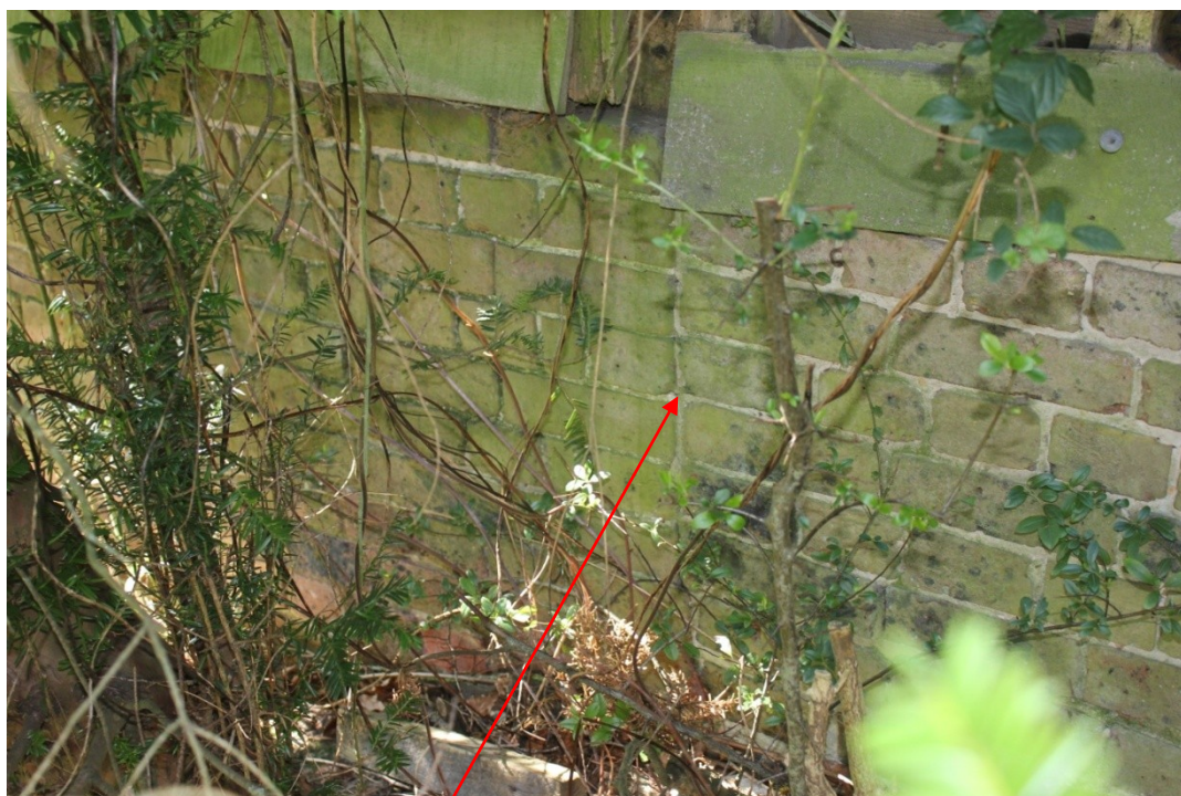
Plate 7. Butt joint in the brickwork of the eastern Midstray.
