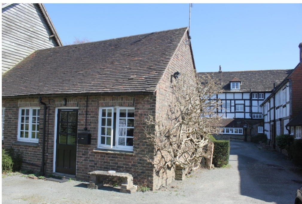
Plate 61. The western elevation of the southern outbuilding.
