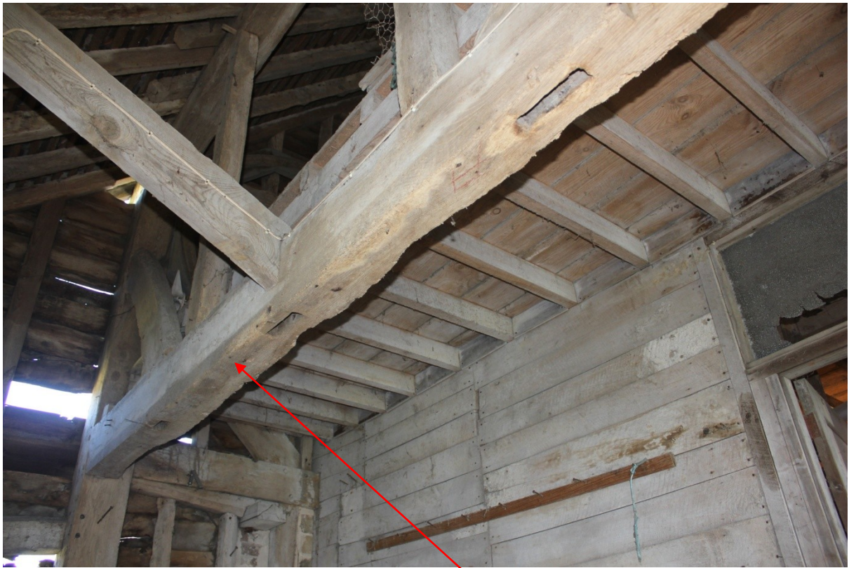
Plate 25. Mortices for missing wall studs and shadow line of missing window head.
