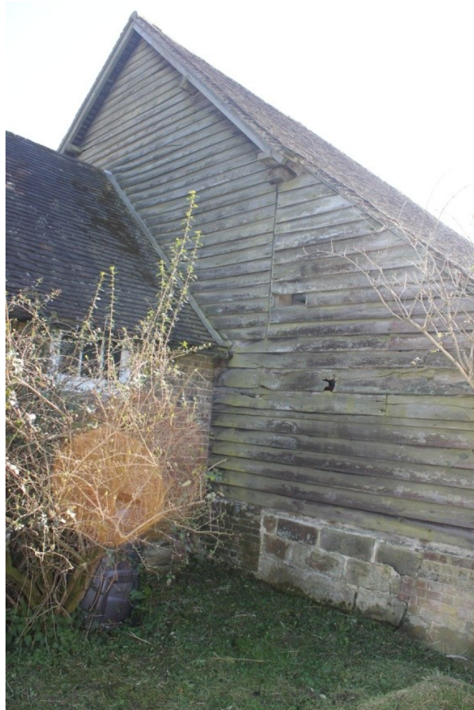
Plate 10. The north side of the single bay outshot attached to the west elevation.
