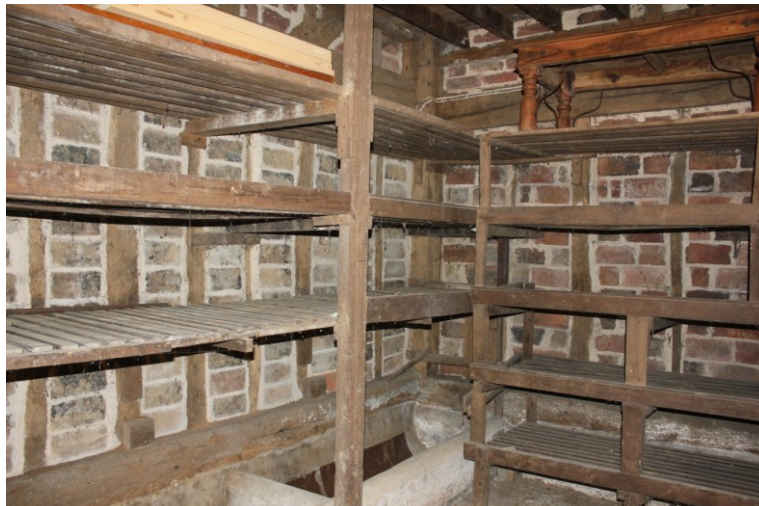
Plate 15. Enclosed north bay with 20 th century racks and infilled walls.
