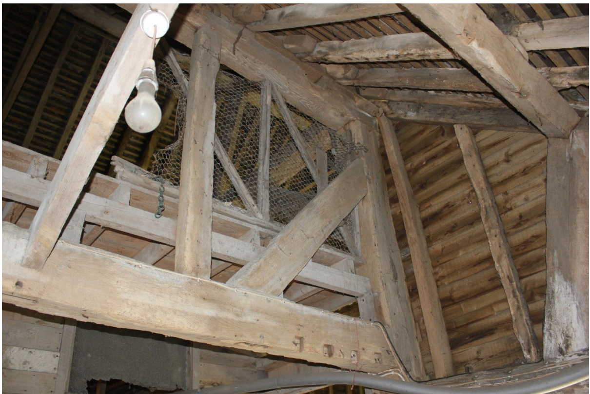
Plate 26. Notches for window mullion in the south side of the western girt.
