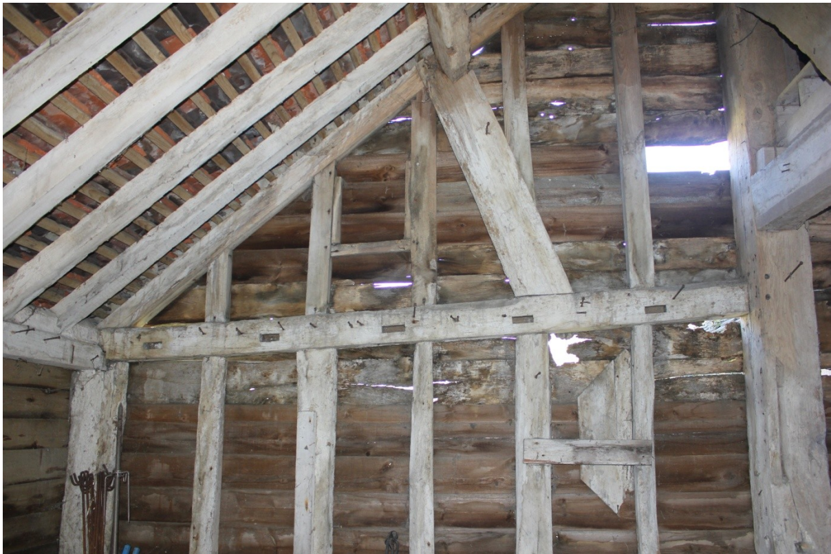
Plate 27. Joist mortices in the northern tie.
