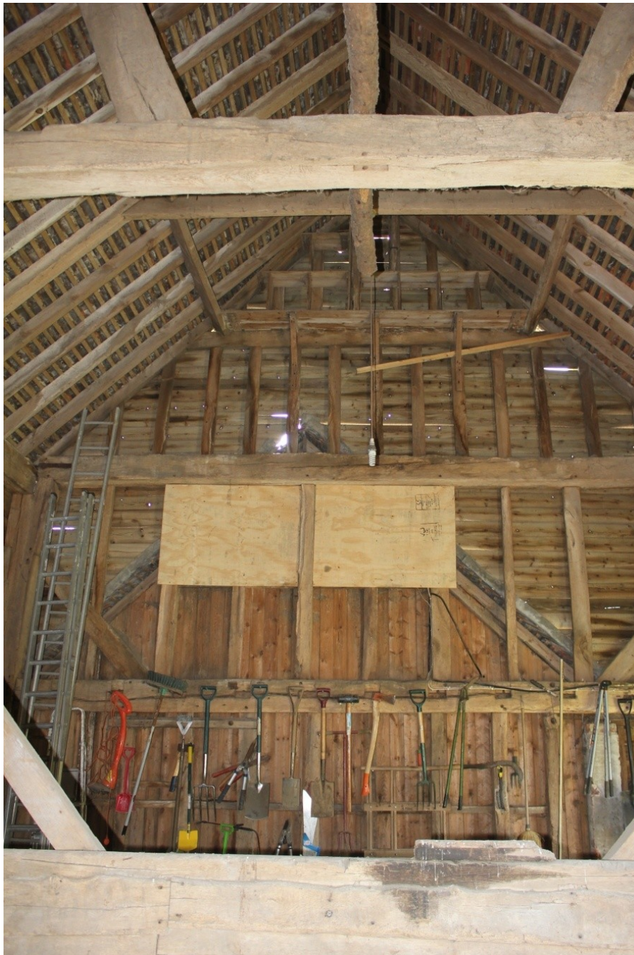
Plate 46. Softwood purlins in the southern bay.
