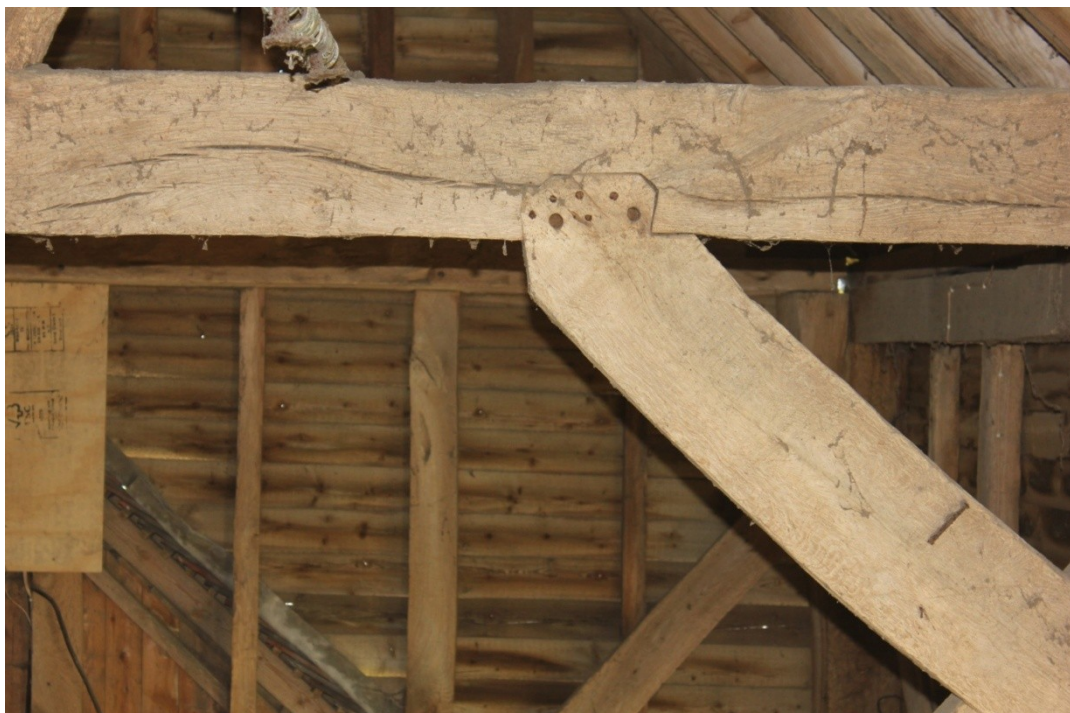
Plate 45. Head bracing in Truss B turned and nailed into place.
