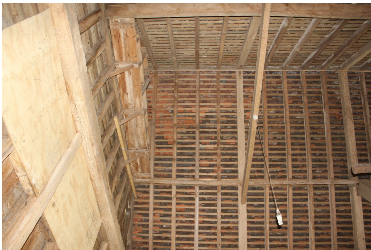
Plate 59. New gable, battens, ridge-board, intermediate collar, rafters and purlins.
