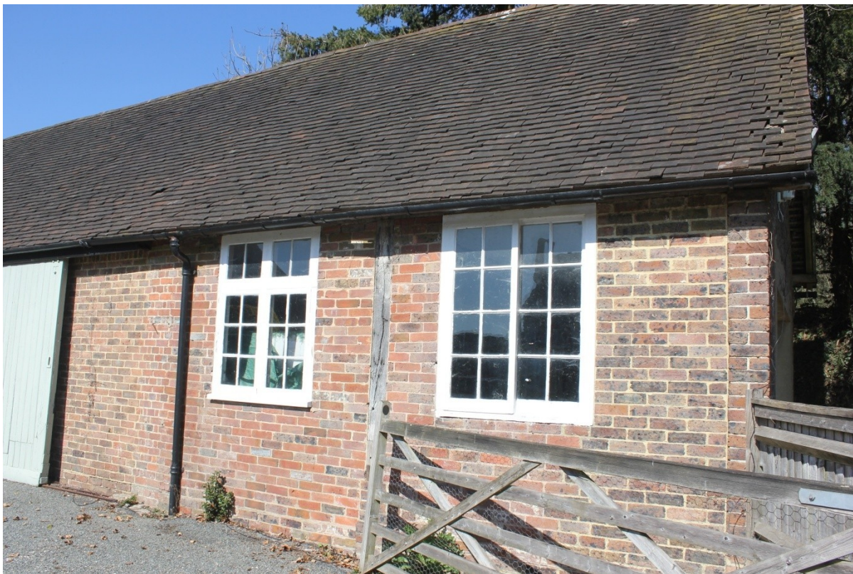
Plate 50. Infilled patched brickwork repairs at the eastern end of the outbuilding.
