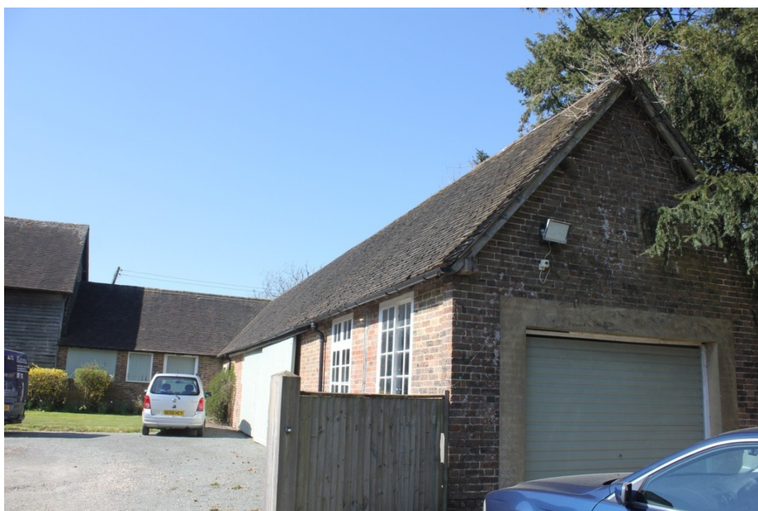
Plate 51. New garage door inserted into the eastern end of the northern outbuilding.
