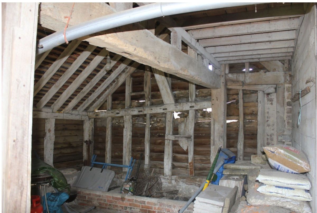
Plate 24. The outshot, looking north.
