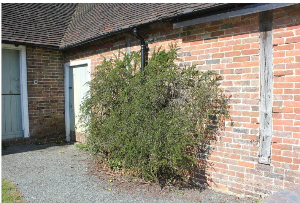
Plate 48. Former post of the open-fronted bay.
