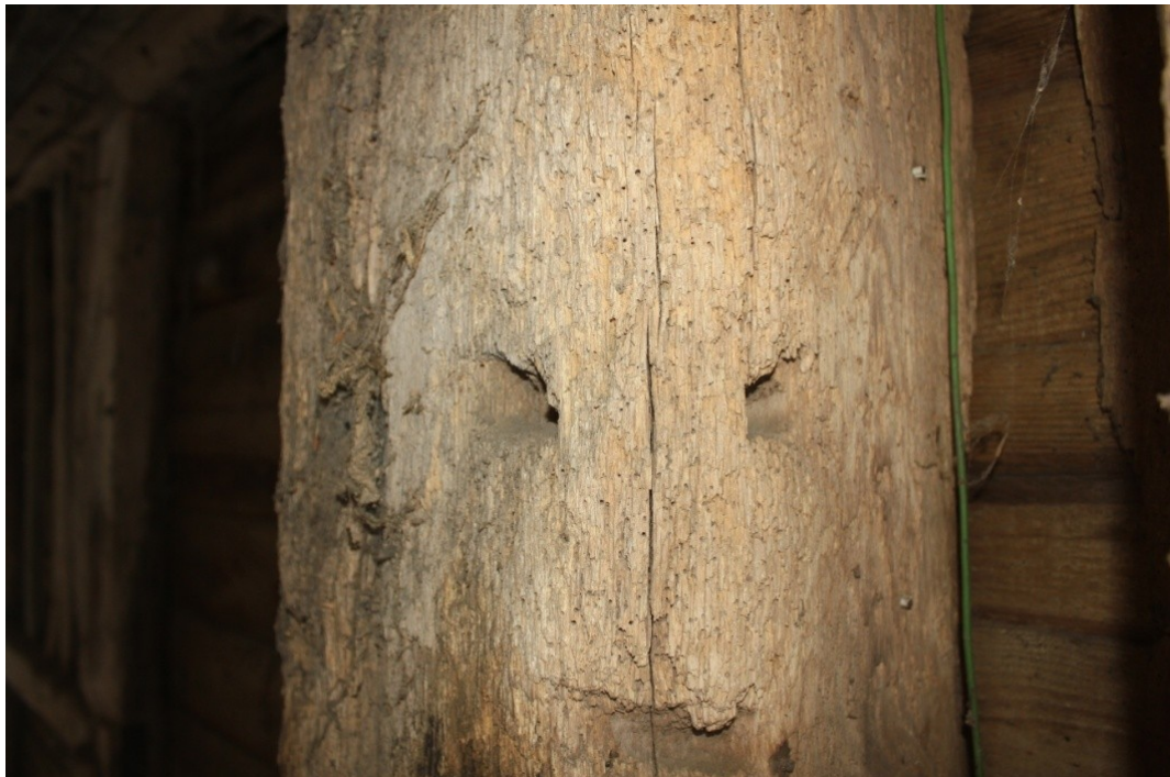
Plate 9. Holes drilled through the corner of a post, possibly for tying rope.
