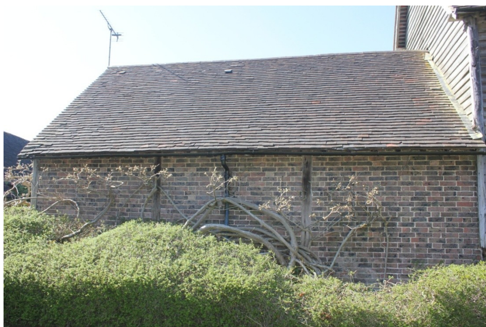
Plate 62. Front, east elevation of the southern outbuilding.
