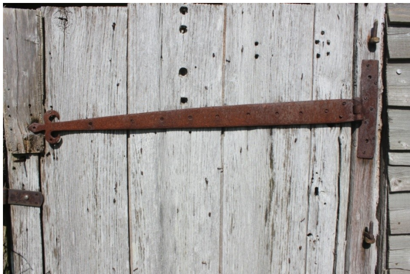
Plate 31. Blacksmith made strap hinges in the outshot door.
