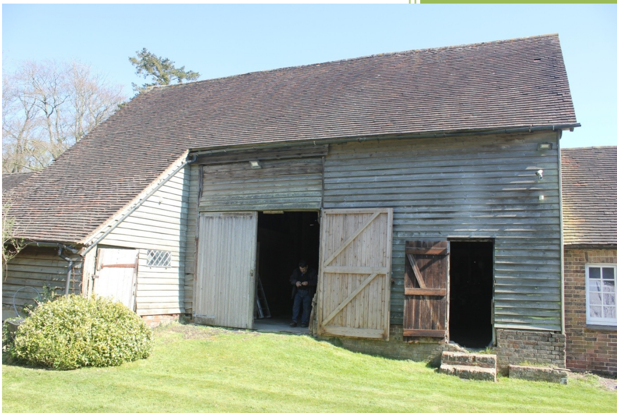
The rear, west facing elevation.
