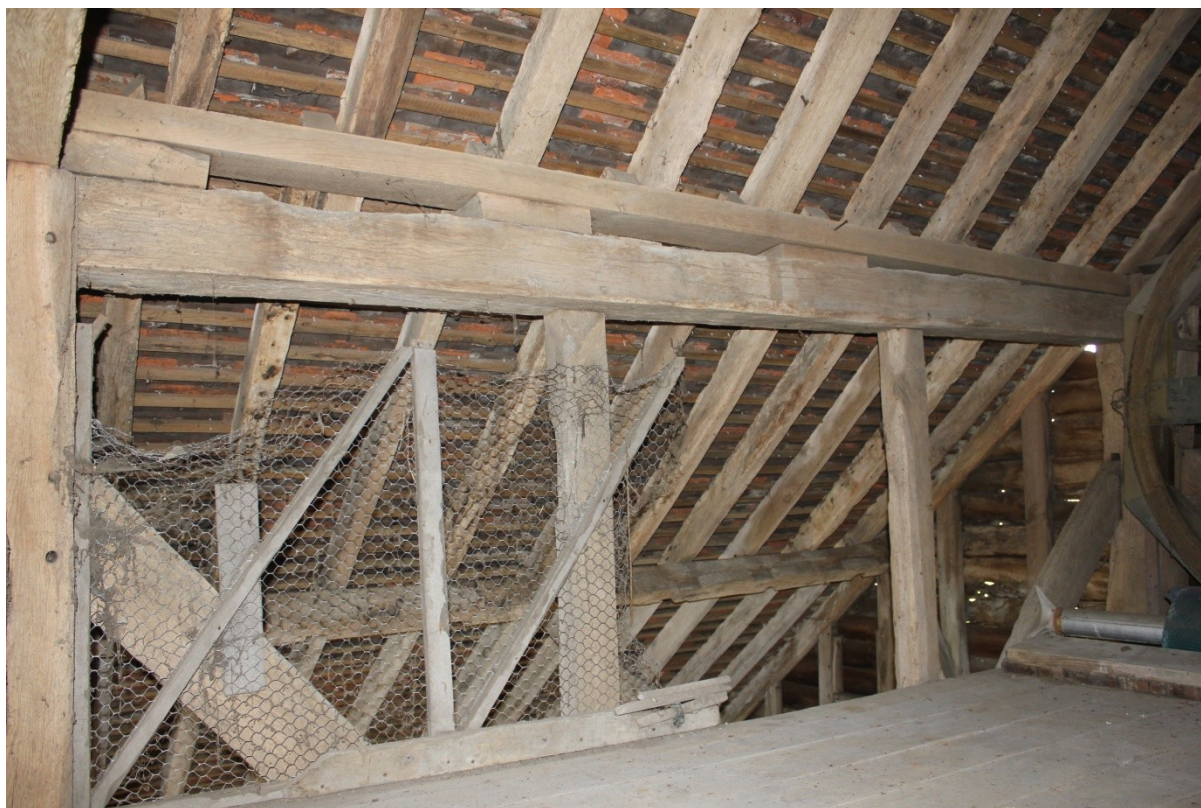
Plate 60. New top wallplates and packing pieces to level the roof.
