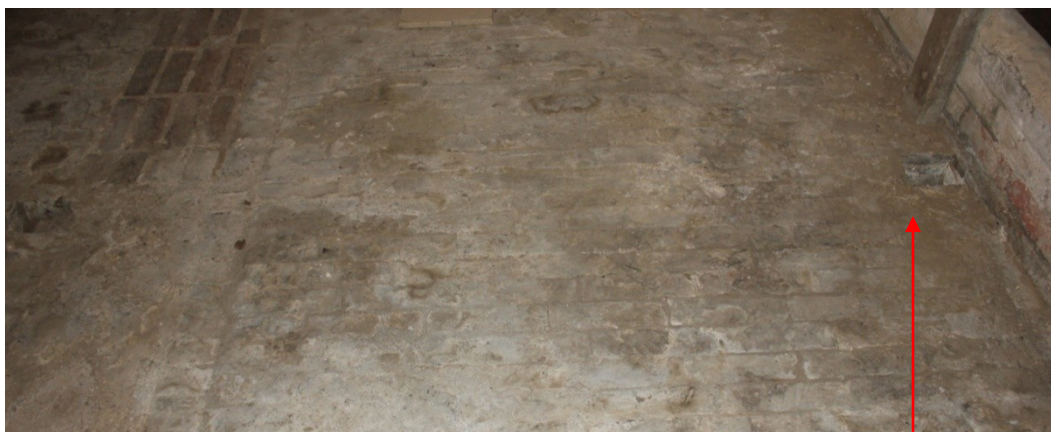
Plate 41. Brick flooring in the northern bay of the Barn with empty sockets within.
