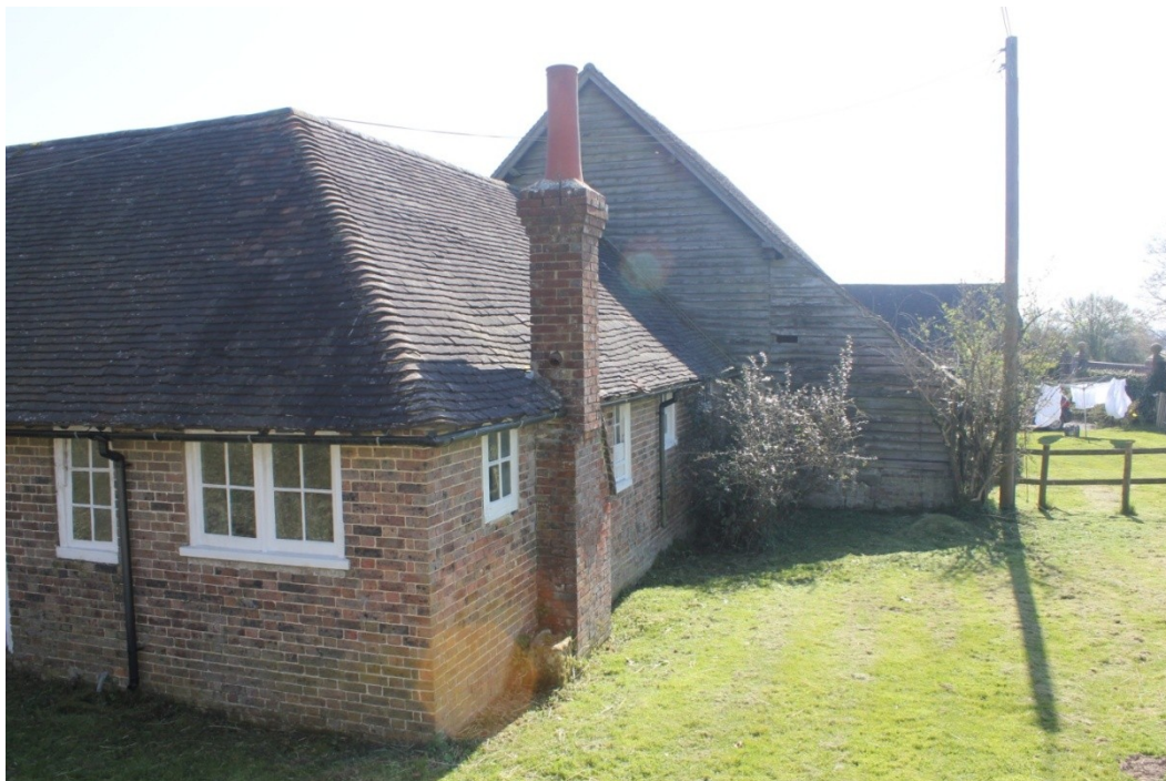
Plate 53. West elevation of the northern outbuilding with chimney stack and windows.
