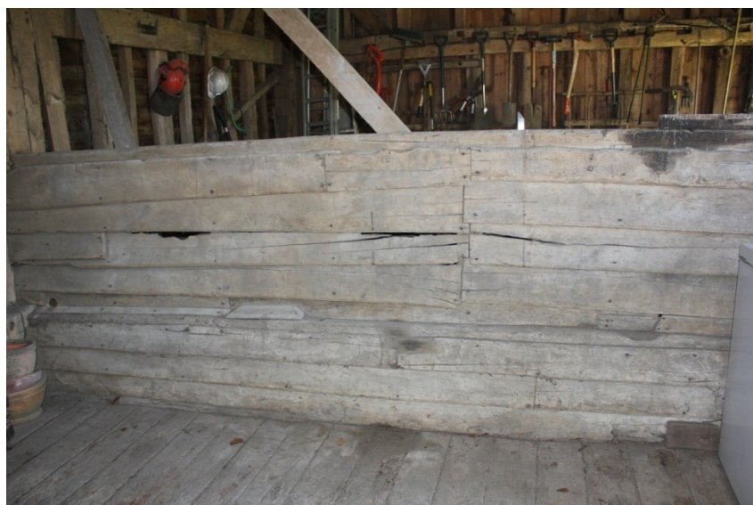
Plate 35. Threshold partition to the south side, with two phases evident.
