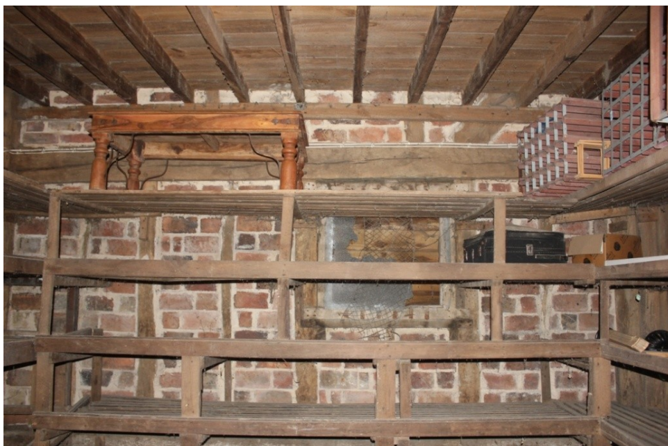
Plate 57. Window inserted in the eastern wall.
