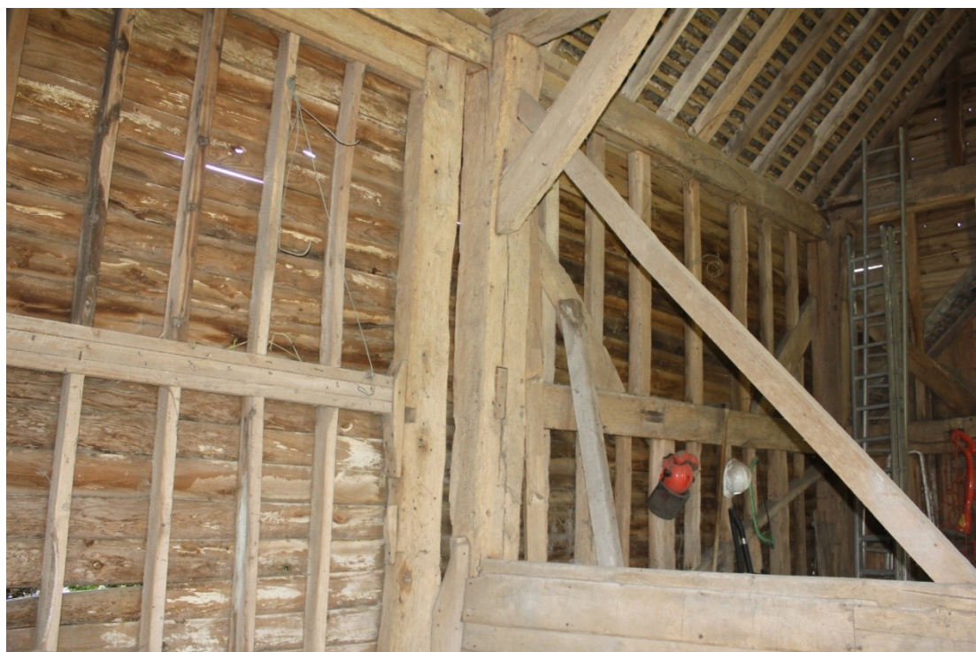
Plate 34. Raking shore morticed into Post BB.
