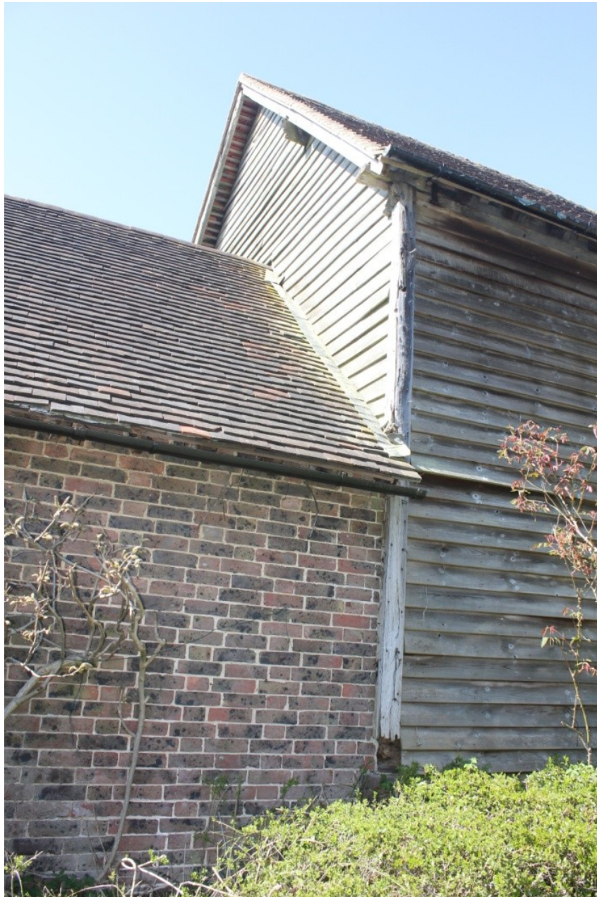
Plate 5. Projecting timbers in the south gable.
