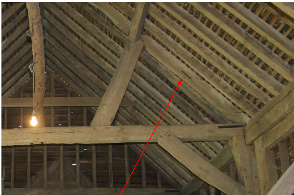
Plate 22. Wind brace mortice on the inner face of Truss B.
