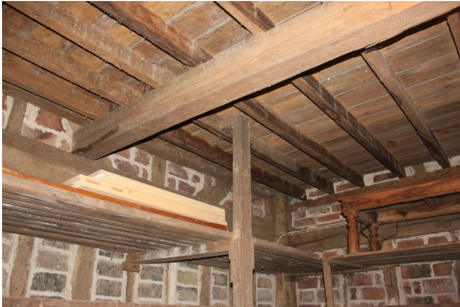
Plate 54. The enclosed storage room in the northern bay.
