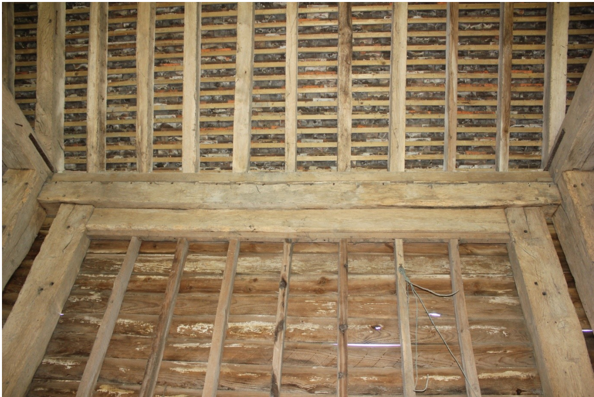
Plate 18. Internal frame within the Wagon way aperture.
