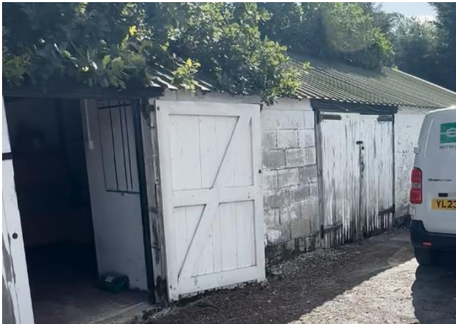
Figure 1; Photographs of the exterior of barn 4
