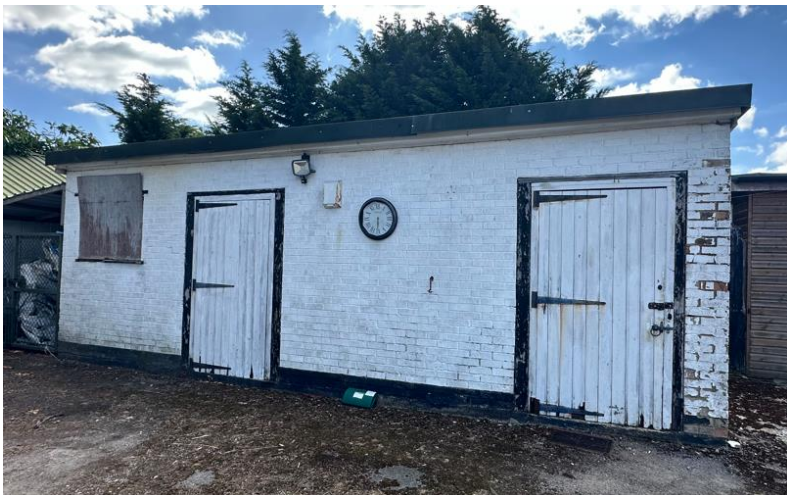
Figure 2; Photographs of the exterior of barn 5
